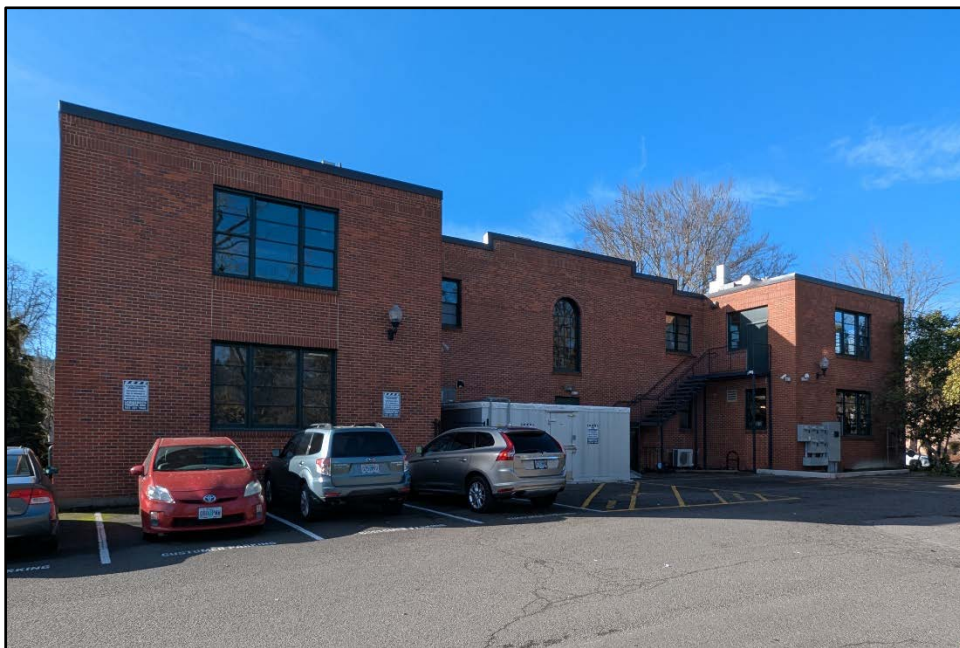
Photo 6 of 20: OR_ClackamasCounty_MilwaukieCityHall_0006 East Elevation (rear), camera facing northwest
