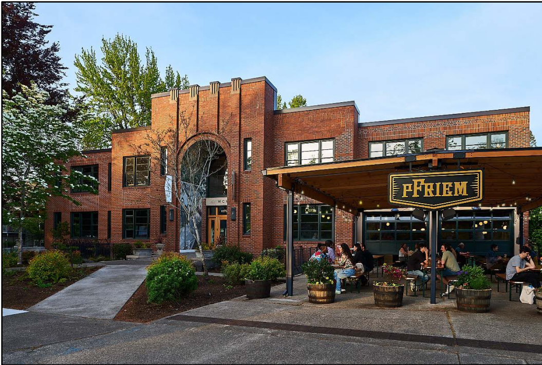
Photo 1 of 20: OR_ClackamasCounty_MilwaukieCityHall_0001 West Elevation (front), camera facing east
