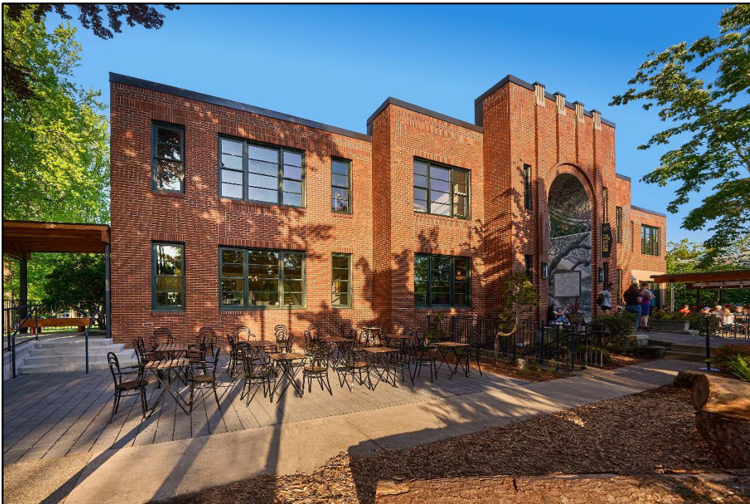
Photo 2 of 20: OR_ClackamasCounty_MilwaukieCityHall_0002 West Elevation (front), camera facing southeast
