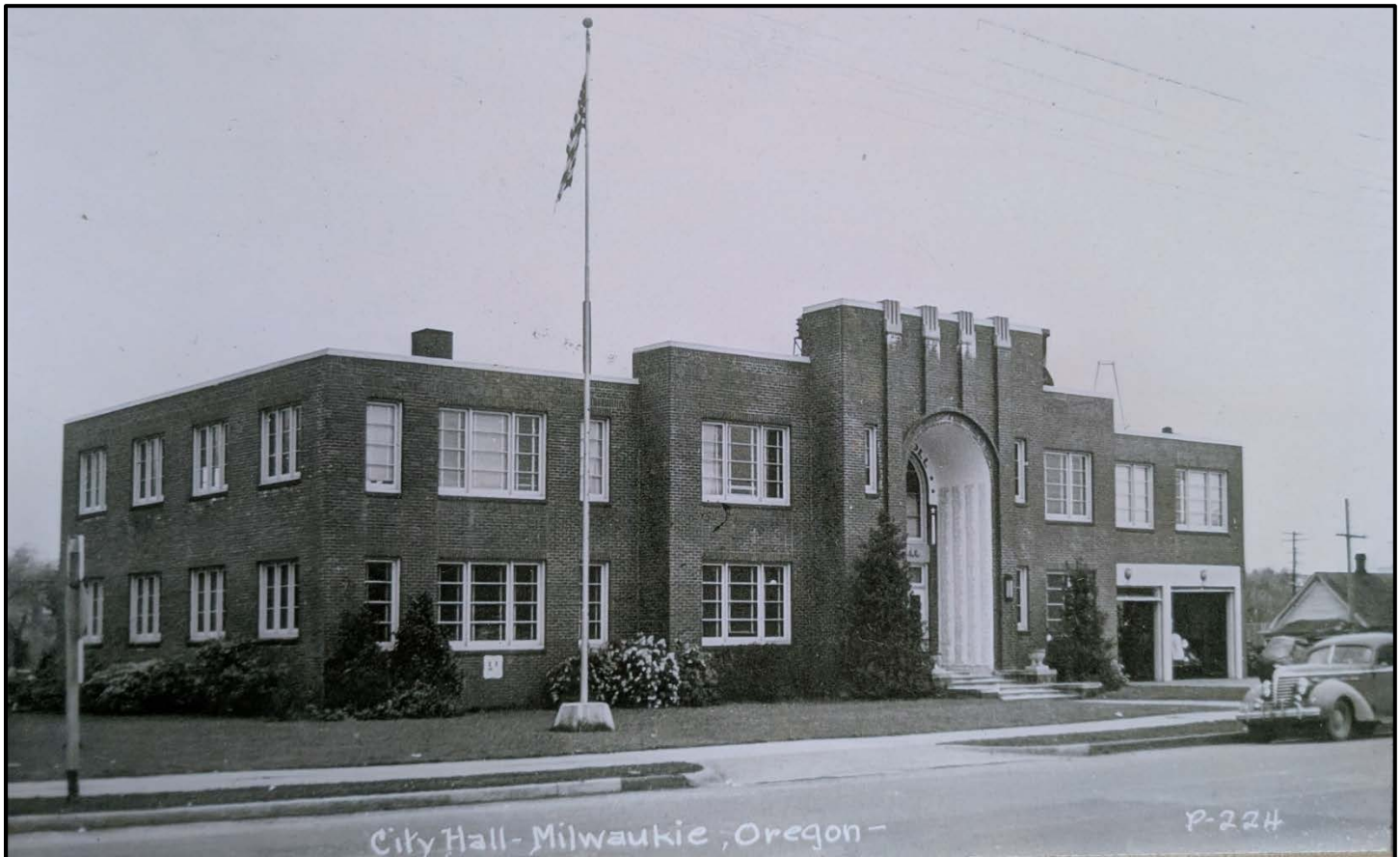
Figure 13. Front (west) side of Milwaukie City Hall, not long after completion. (c.1940). Source: City of Milwaukie.
