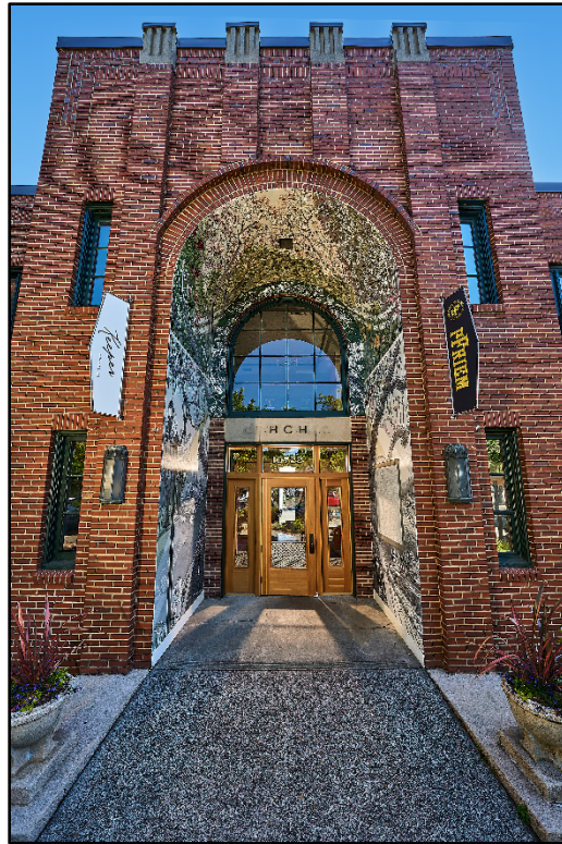
Photo 3 of 20: OR_ClackamasCounty_MilwaukieCityHall_0003 Front Entrance Detail, camera facing east
