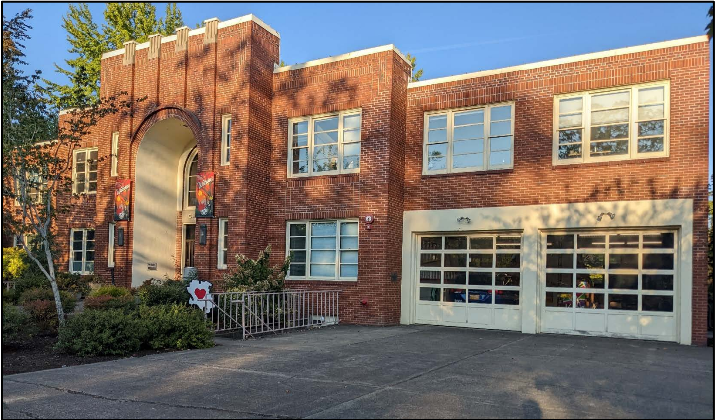
Figure 17. Front (west) side of Milwaukie City Hall in 2022, prior to building rehabilitation work. Source: Val C. Ballestrem.
