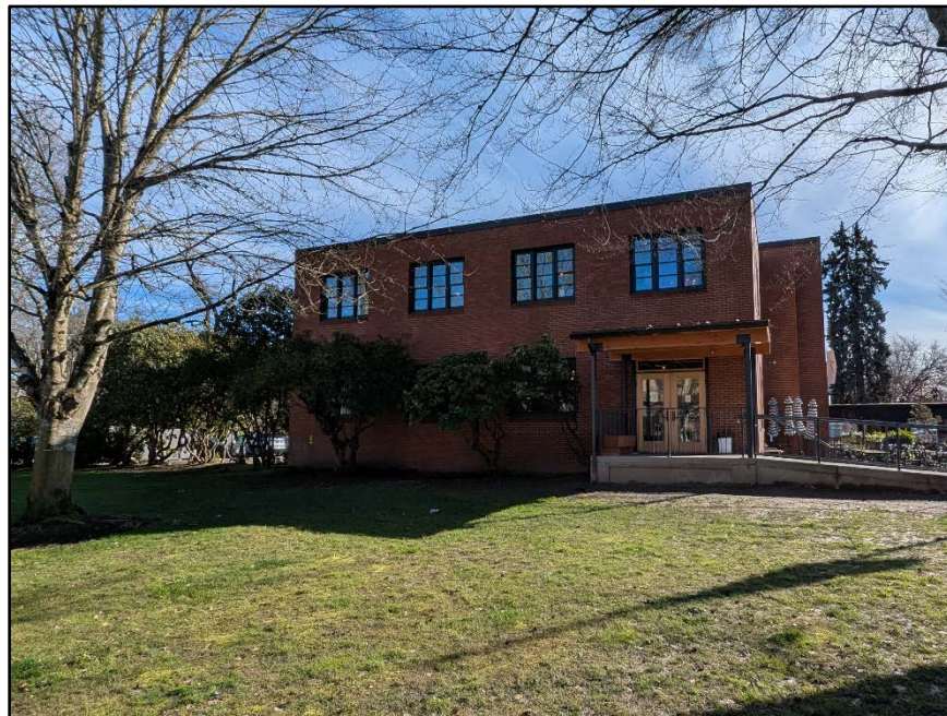
Photo 4 of 20: OR_ClackamasCounty_MilwaukieCityHall_0004 North Elevation, camera facing south
