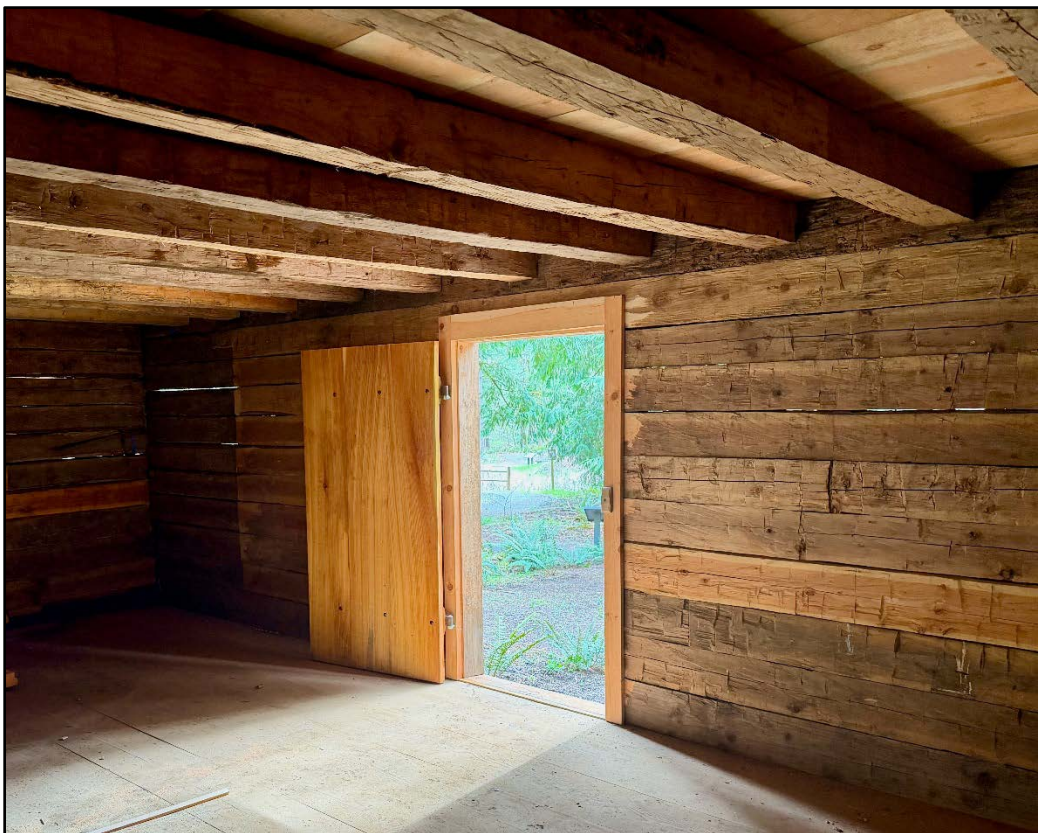
Photograph 12 of 15. OR_ClackamasCounty_MolallaLogHouse_0012 Interior, first floor, southeast corner.
