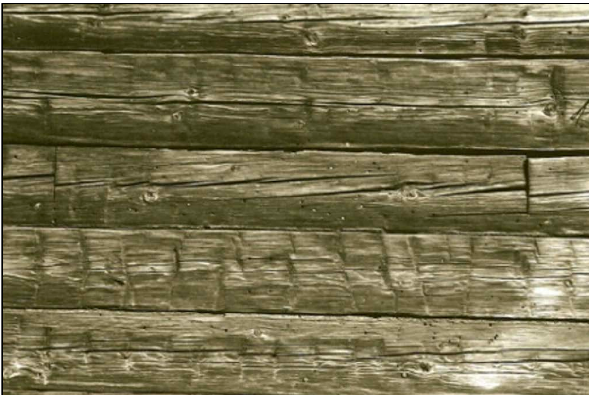
Photograph 9 of 15. OR_ClackamasCounty_MolallaLogHouse_0009 North elevation showing kerf marks indicating planned openings. Photographed 2008.
