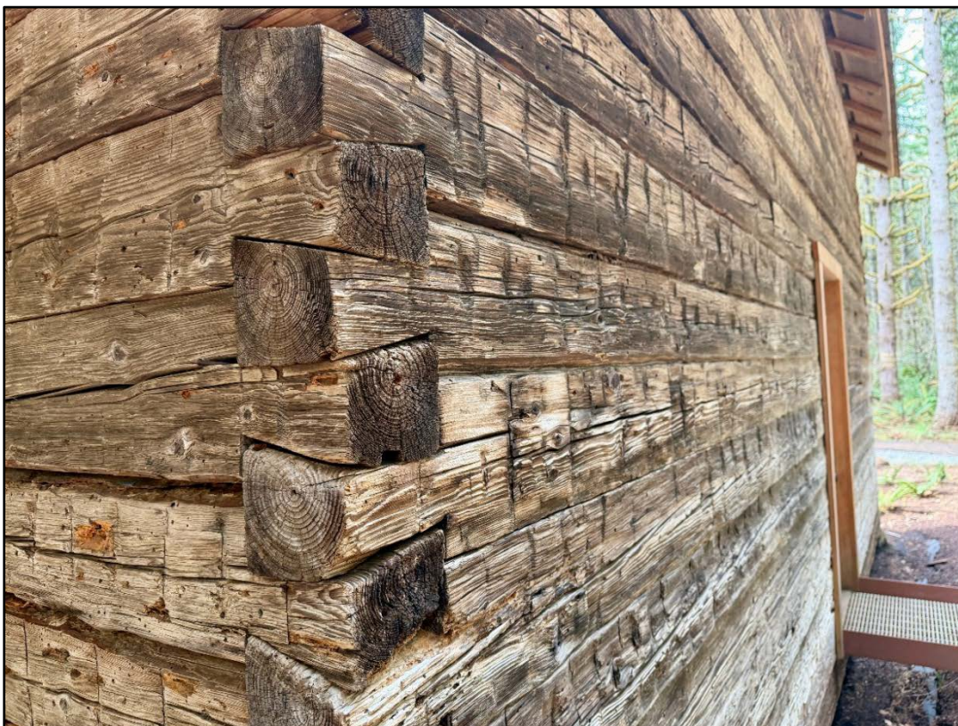
Photograph 8 of 15. OR_ClackamasCounty_MolallaLogHouse_0008 Northeast corner detail showing half-dovetail notching and axe marks. Photographed 2025.
