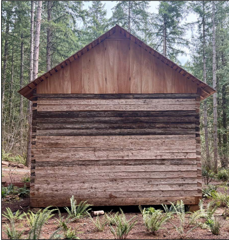
Photograph 5 of 15. OR_ClackamasCounty_MolallaLogHouse_0005 West elevation. View to the east.
