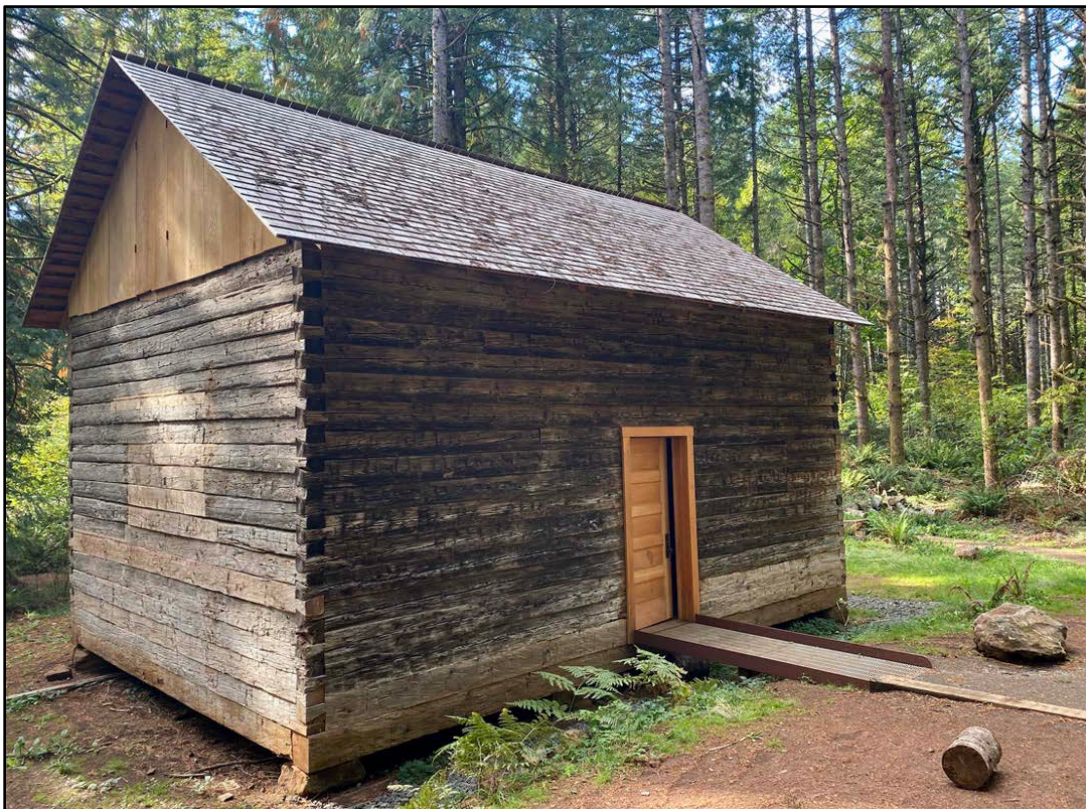
Photograph 6 of 15. OR_ClackamasCounty_MolallaLogHouse_0006 Oblique view of northeast corner prior to shed roof installation. Photographed 2025. View to the southwest.
