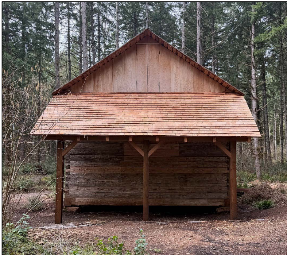
Photograph 4 of 15. OR_ClackamasCounty_MolallaLogHouse_0004 East elevation. View to the west.
