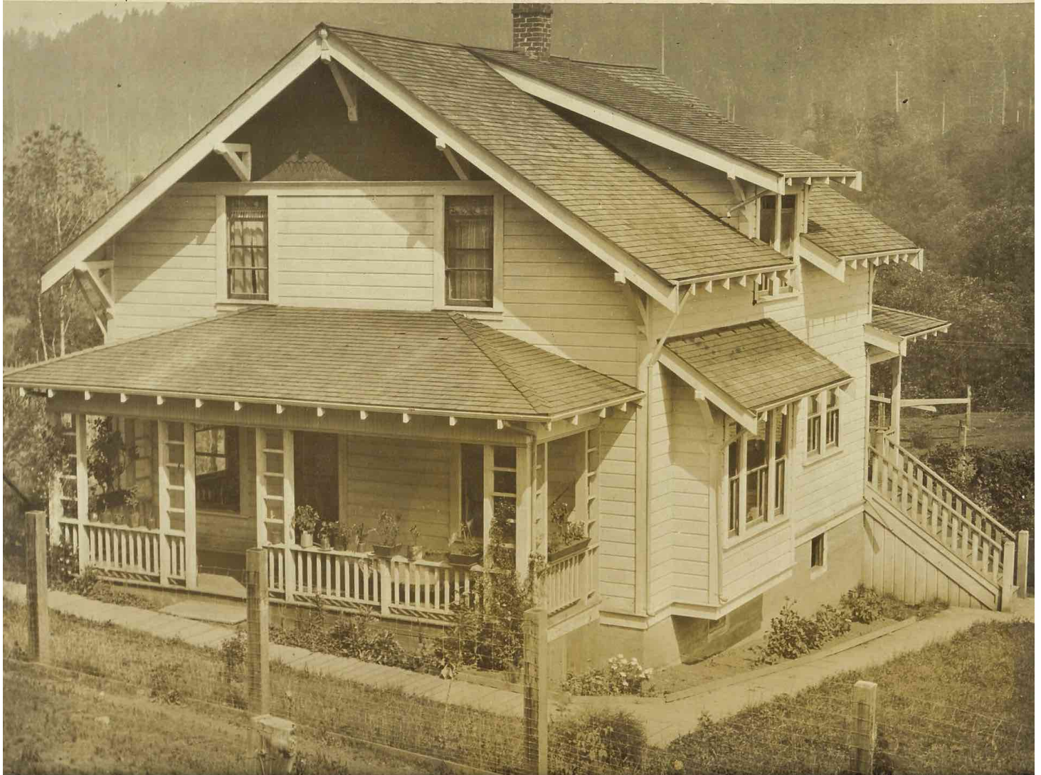
Figure 26. 1914 Cahill-Nordstrom House, circa 1915. Cahill-Nordstrom Family Collection.
