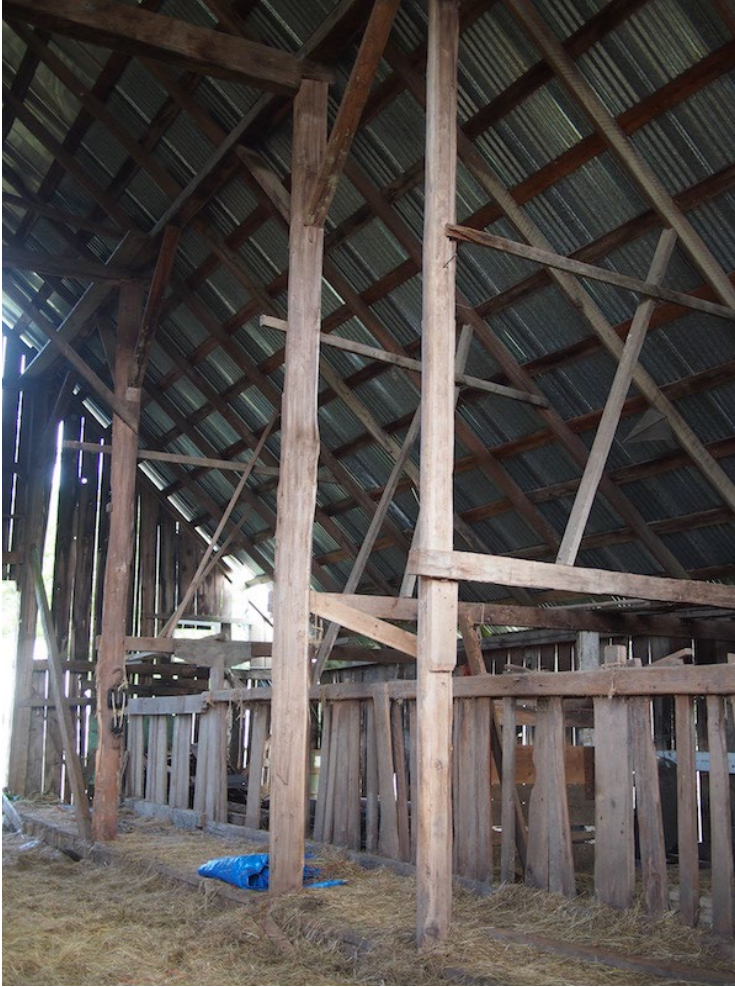
Photo 12. Interior of barn looking west showing structure and new metal roof, with remaining shingle roofing visible on right (north) slope.
