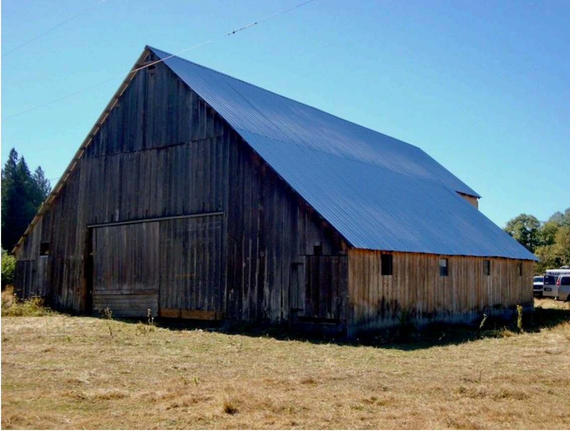
Photo 7. Cahill-Nordstrom barn, east and north sides, view looking west/southwest.
