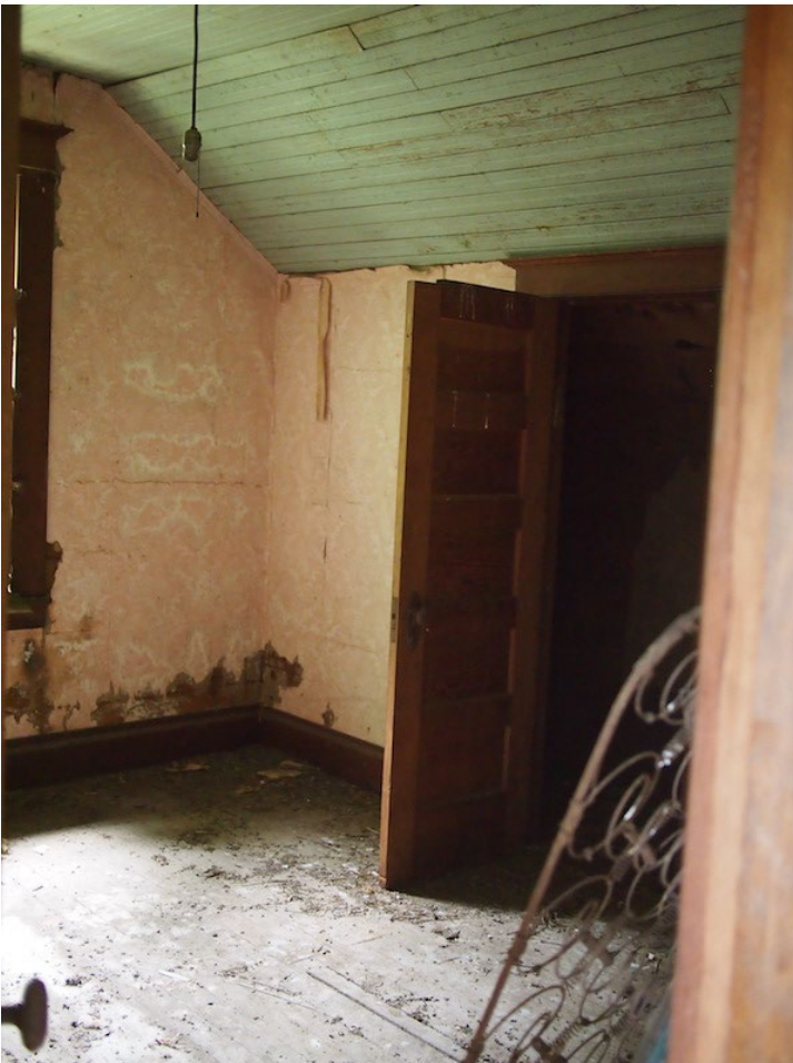
Photo 6. Cahill-Nordstrom house, upstairs bedroom.
