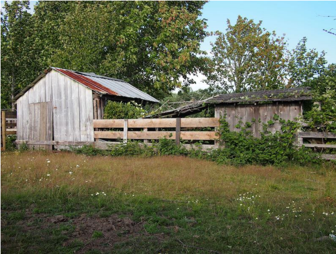
Photo 17. Woodshed and Gas House, view looking east toward Cahill Road.
