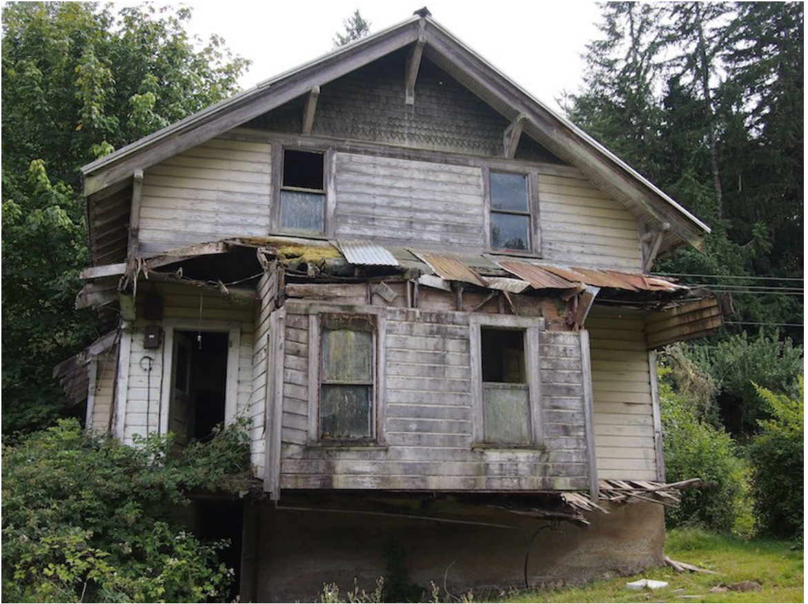
Figure 37. Cahill-Nordstrom House, rear elevation prior to removal of deteriorated back section, c. 2016. Courtesy Celena Kathan.
