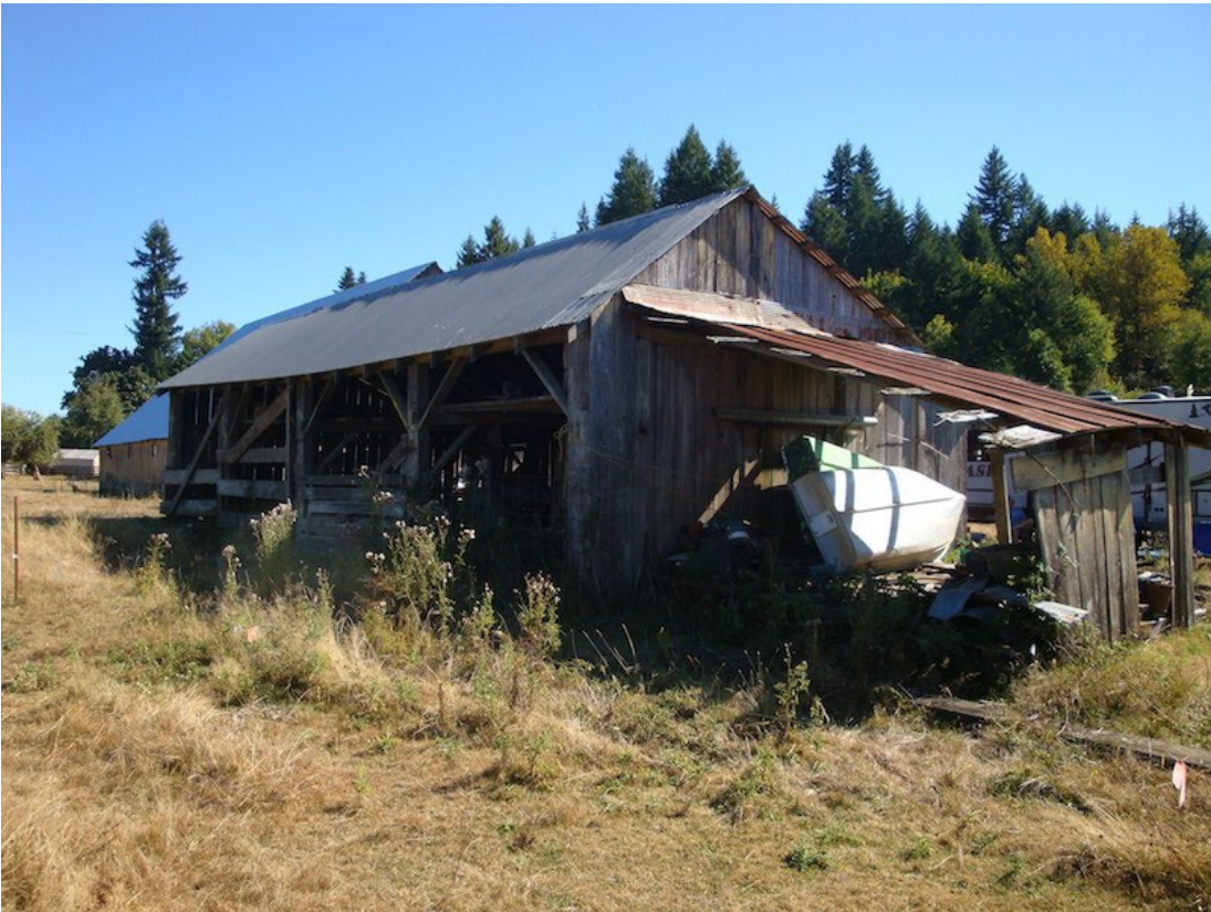
Photo 14. Machine shed, view looking southeast.
