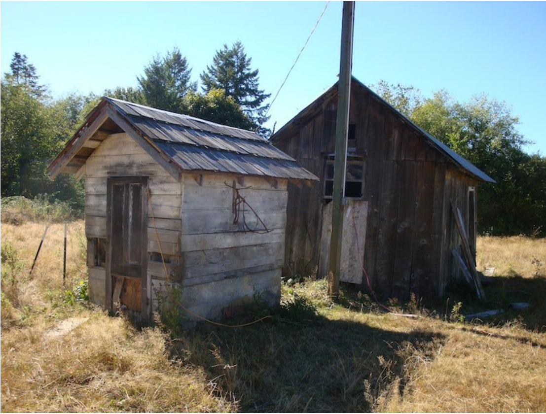
Photo 15. Pump house (left) and Shop (right), view looking west.
