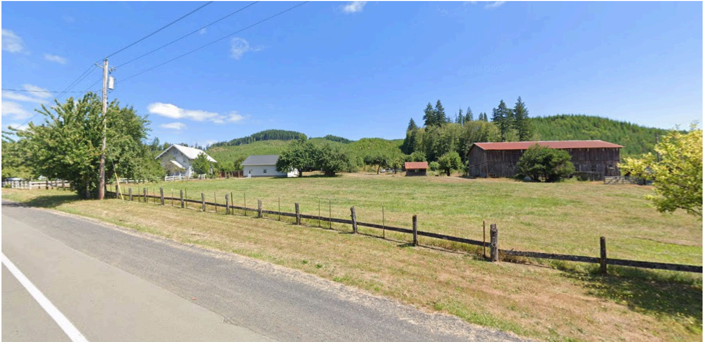
Figure 41. Anton and Julianna Birkenfeld House and Barn, 11164 Highway 202, Birkenfeld, Columbia County, July 2019. Courtesy Google.
