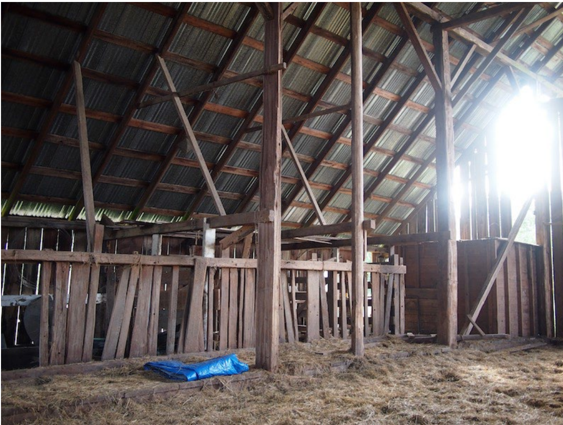
Photo 10. Cahill-Nordstrom barn, interior, southwest corner with walls of separator room visible.
