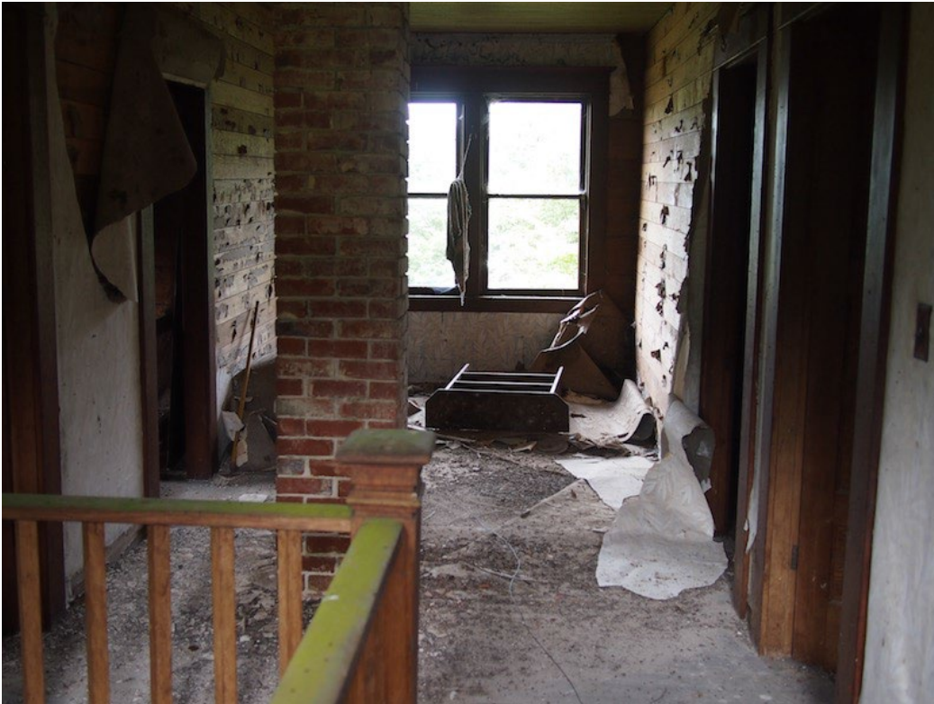
Photo 5. Cahill-Nordstrom house, upstairs hall looking east.
