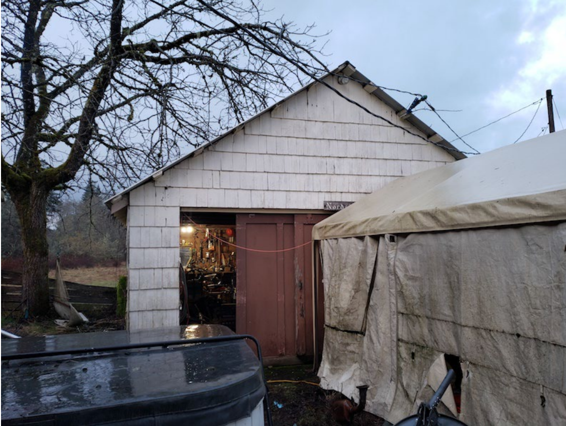
Photo 21. Francis and Helen Nordstrom garage, view of east elevation, looking west.
