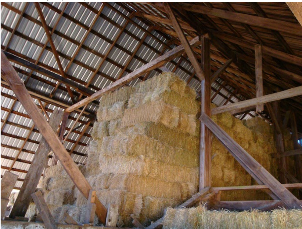
Photo 12. Interior of barn looking west showing structure and new metal roof, with remaining shingle roofing visible on right (north) slope.
