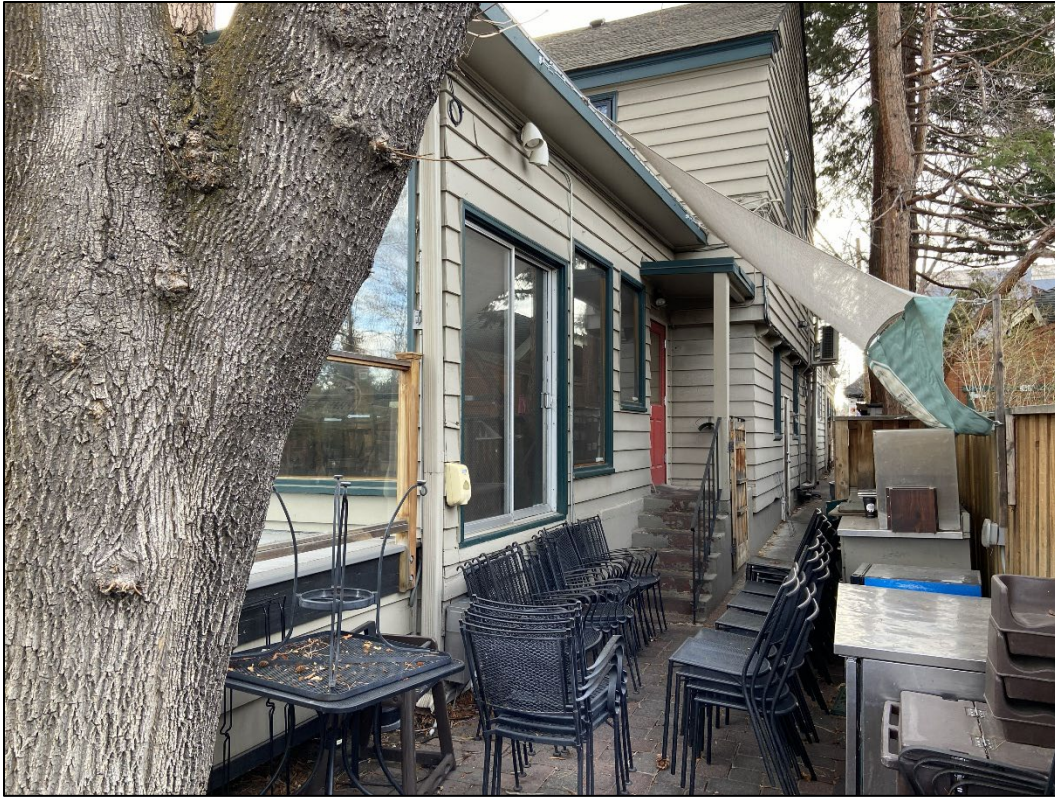
Photograph 7 of 15: OR_DeschutesCounty_PineTavern_0007 The west half of the Pine Tavern's southwest elevation, view facing northeast.
