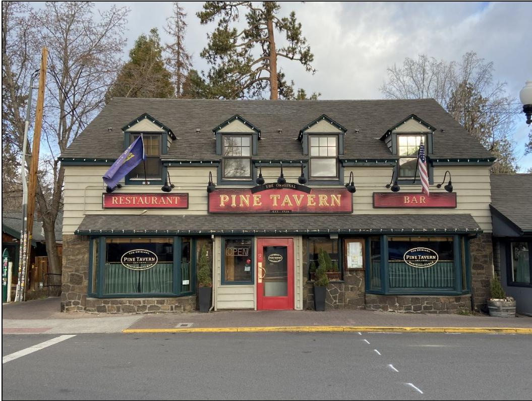
Photograph 1 of 15: OR_DeschutesCounty_PineTavern_0001 The Pine Tavern façade, view facing northwest.
