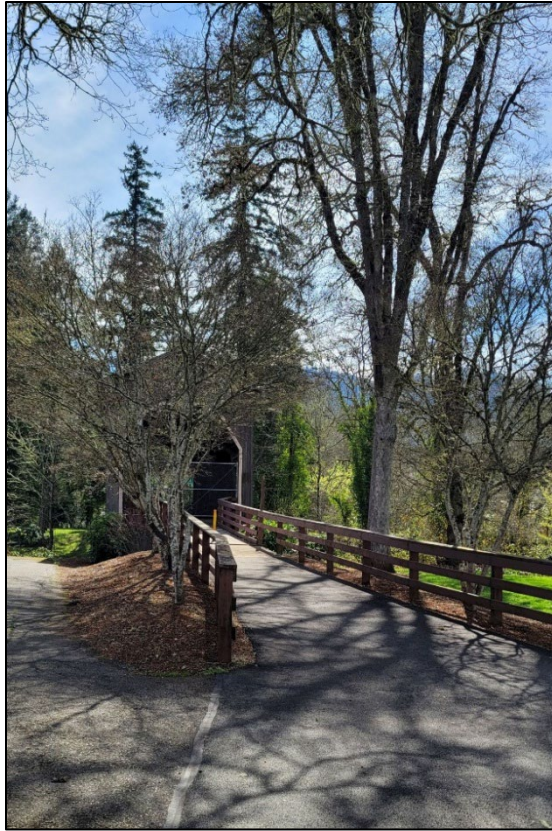
Photograph 3 of 9: OR_DouglasCounty_PassCreekCoveredBridge_0003 Overview of Pass Creek Covered Bridge, camera facing south.
