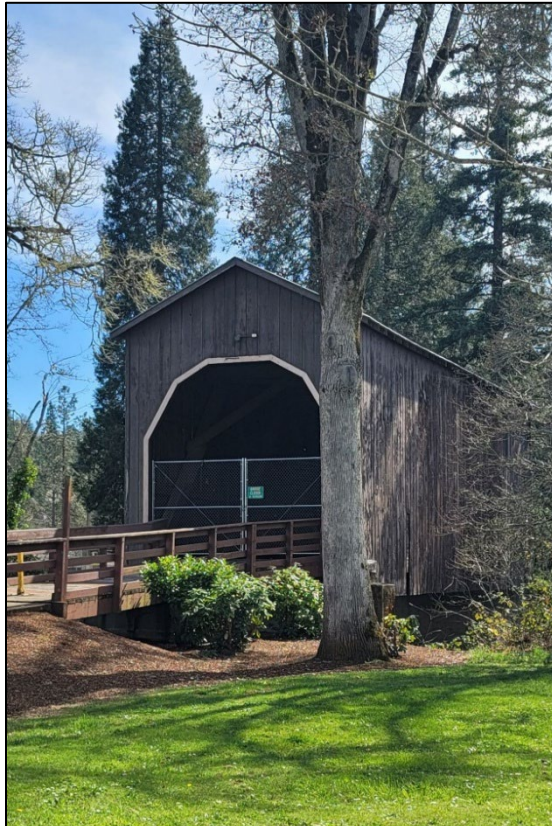
Photograph 4 of 9: OR_DouglasCounty_PassCreekCoveredBridge_0004 North portal and west wall of Pass Creek Covered Bridge, camera facing southeast.
