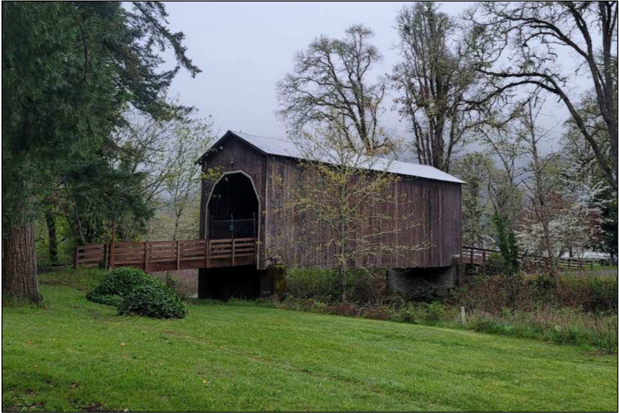
Photograph 1 of 9: OR_DouglasCounty_PassCreekCoveredBridge_0001 Overview of Pass Creek Covered Bridge, camera facing northwest.
