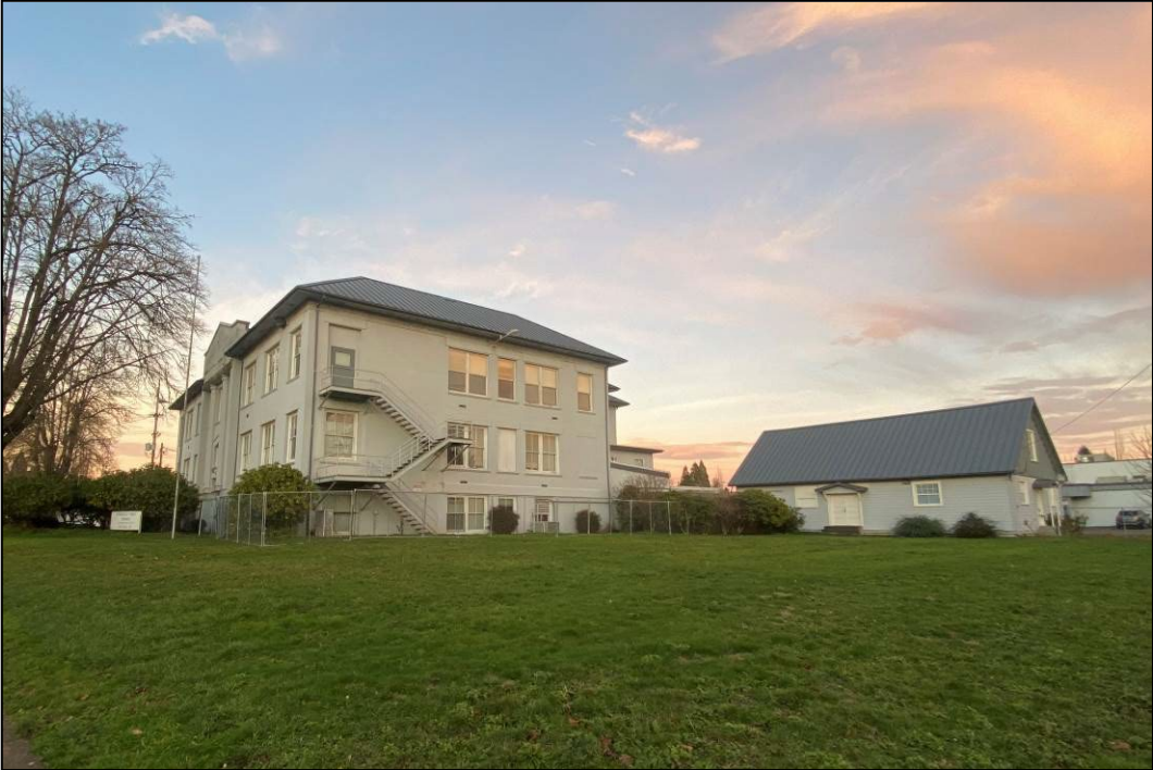
Photo 3 of 16: West and south elevations and west elevation of manual training building, looking northeast.
