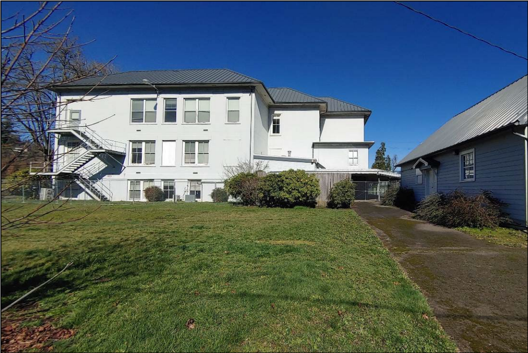
Photo 4 of 16: South elevation and manual training building, looking north.
