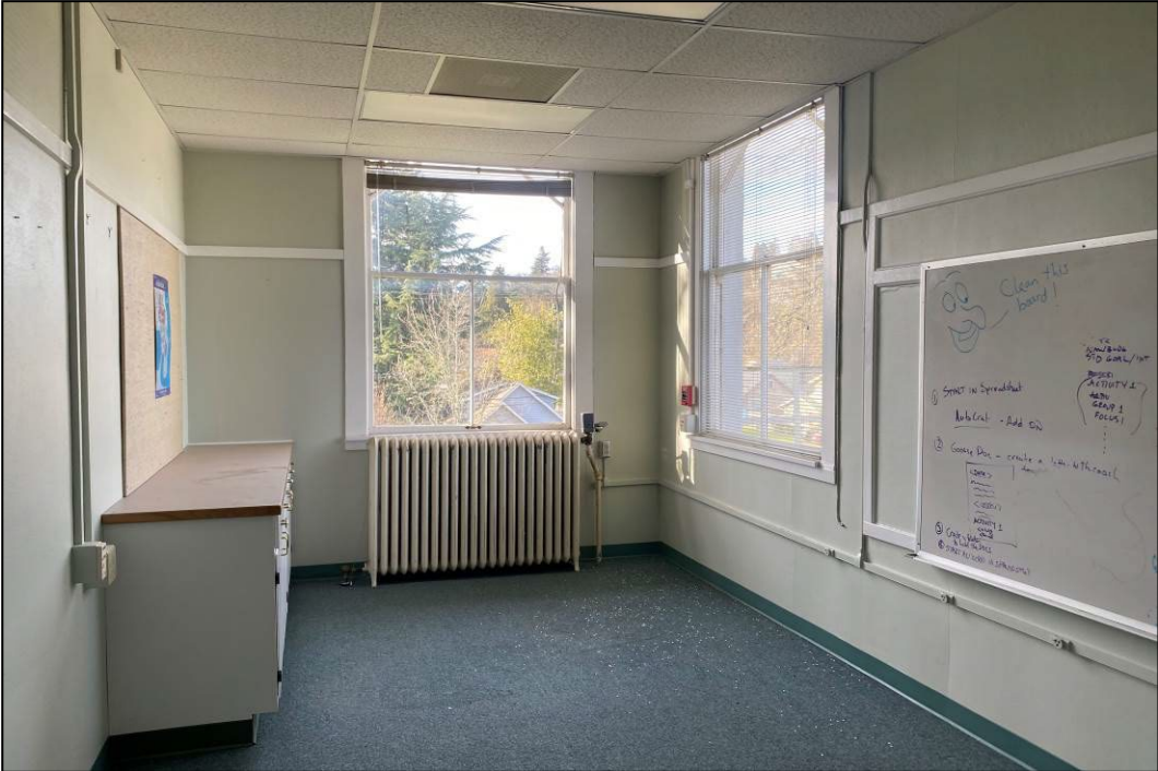
Photo 13 of 16: Corner room on second floor looking northwest.
