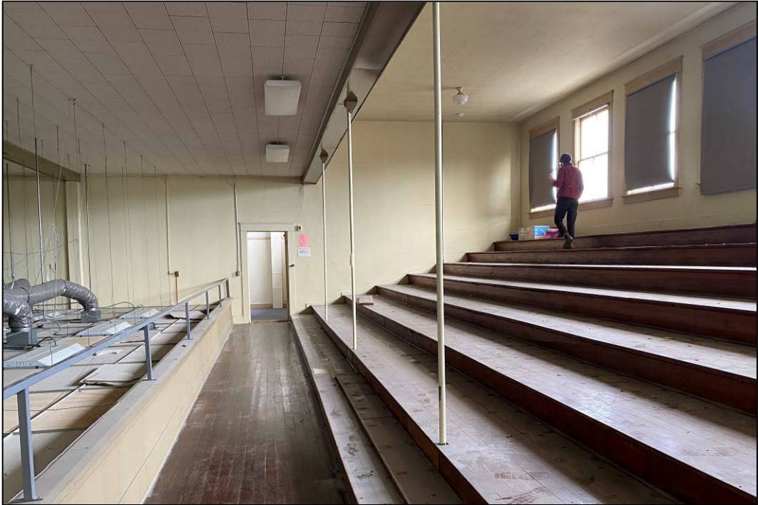
Photo 15 of 16: Auditorium balcony looking north.
