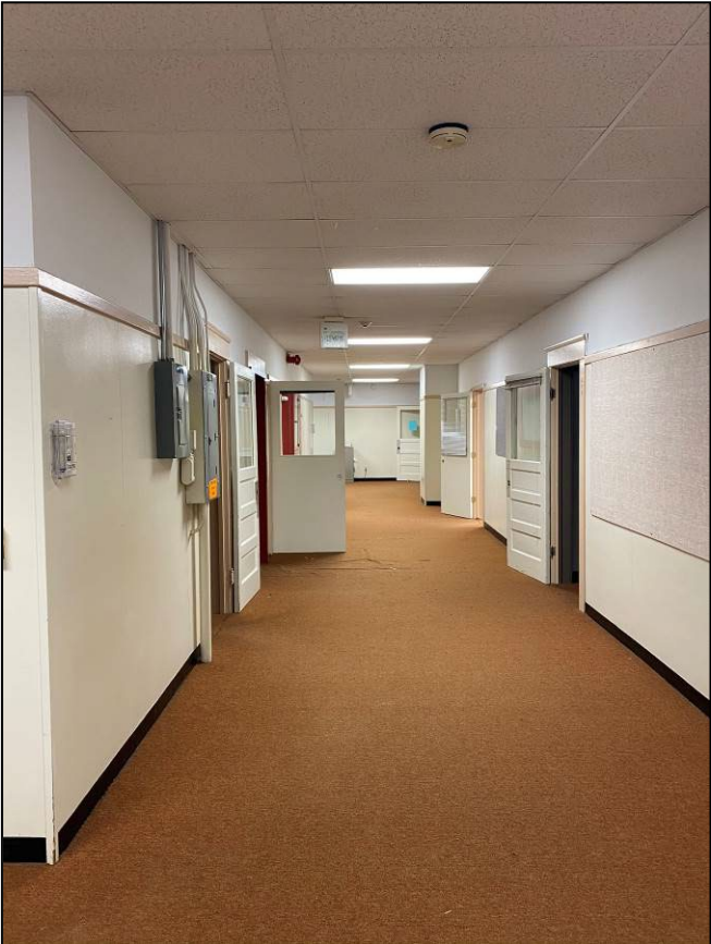
Photo 10 of 16: Corridor looking south.
