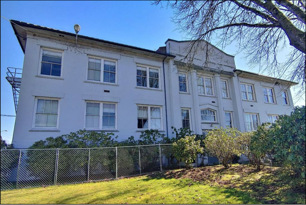
Photo 2 of 16: West elevation looking east.
