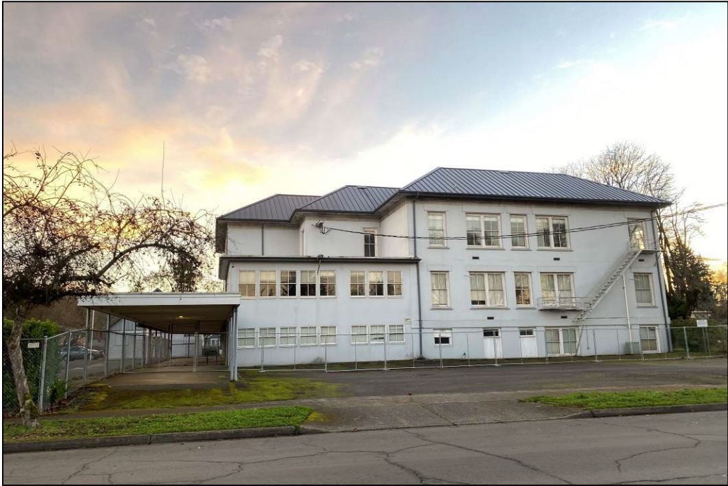
Photo 5 of 16: North elevation looking south.
