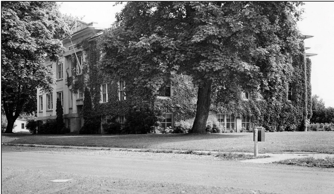
Figure 15: Springfield High school, c. 1945 with detail of front façade below. 258
