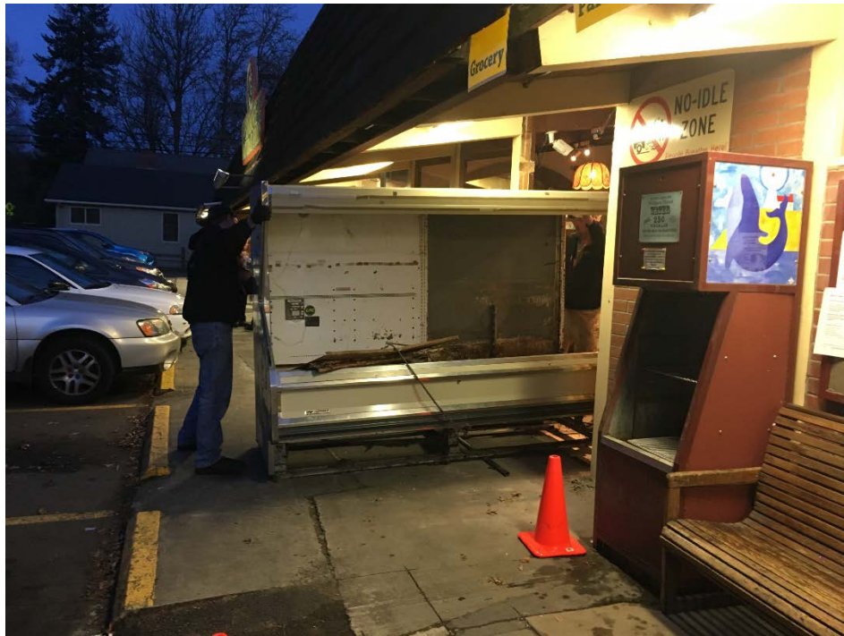
Figure 23a and 23b: Cooler replacement, 2018
