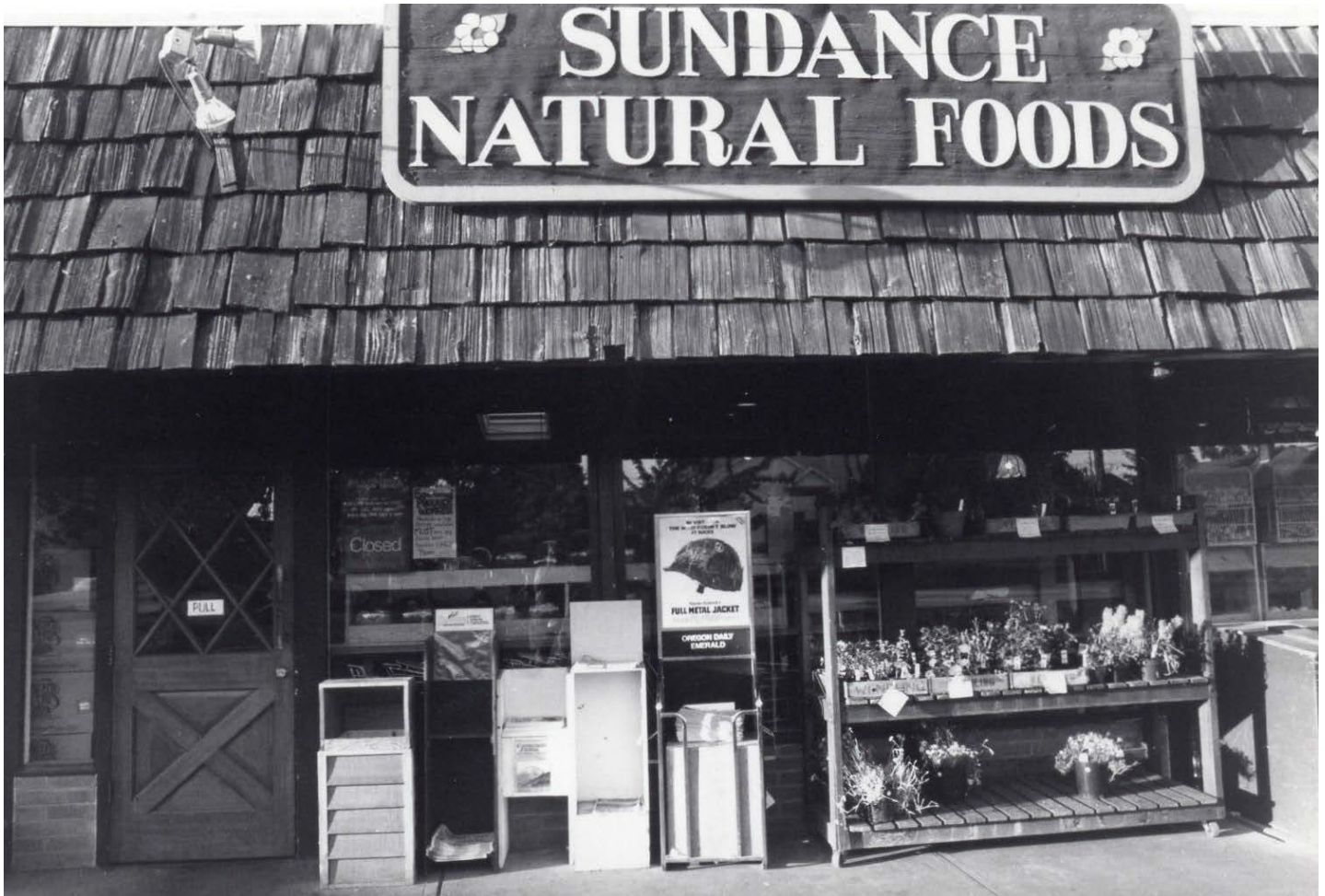
Figure 14: Exterior, main north elevation, 1987. (Sundance Natural Foods)
