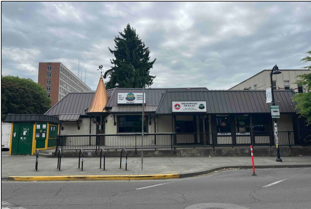
Photograph 3 of 15: OR_LaneCounty_TaylorsCoffeeShop_0003 North elevation, view south.
