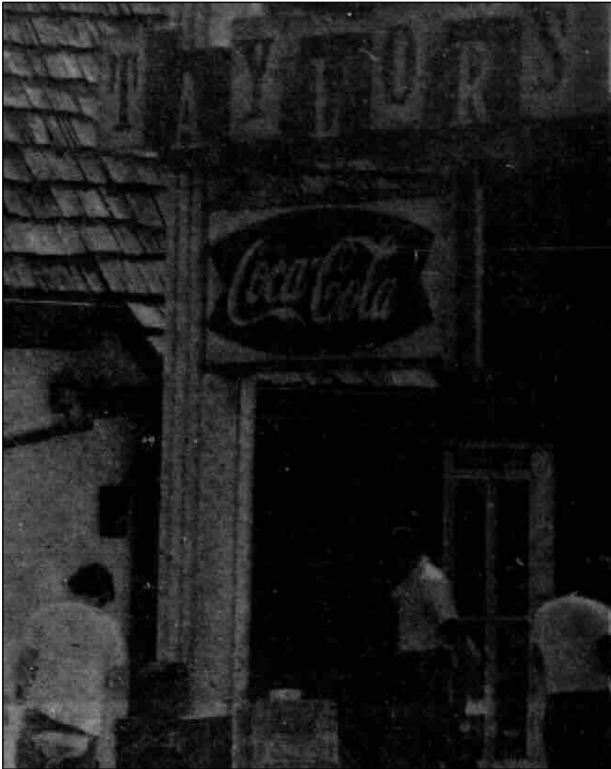
Figure 12 of 17: North elevation of Taylor's with shake roof visible and non-extant pole sign Oregon Daily Emerald, 1969
