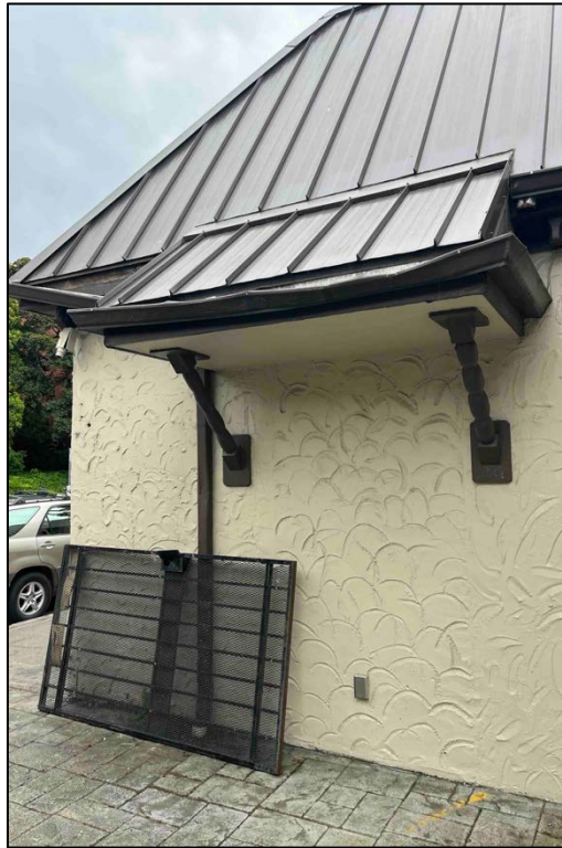
Photograph 7 of 15: OR_LaneCounty_TaylorsCoffeeShop_0007 Infilled door below awning at north elevation, view southeast.
