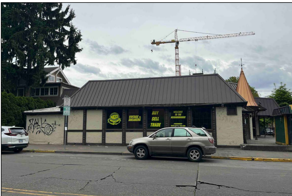
Photograph 4 of 15: OR_LaneCounty_TaylorsCoffeeShop_0004 East elevation, view west.
