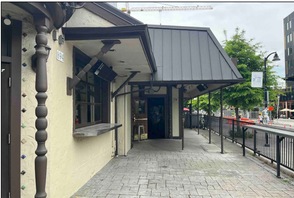
Photograph 8 of 15: OR_LaneCounty_TaylorsCoffeeShop_0008 West portion of building with second entrance visible, view west.
