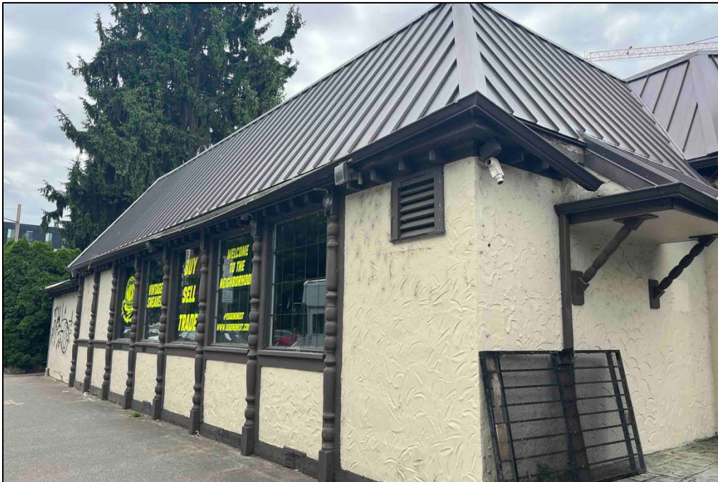
Photograph 9 of 15: OR_LaneCounty_TaylorsCoffeeShop_0009 East elevation, view southwest.
