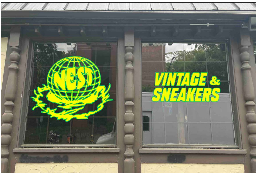
Photograph 10 of 15: OR_LaneCounty_TaylorsCoffeeShop_0010 Detail of windows, turned wood pilasters, and eave corbels, view west.
