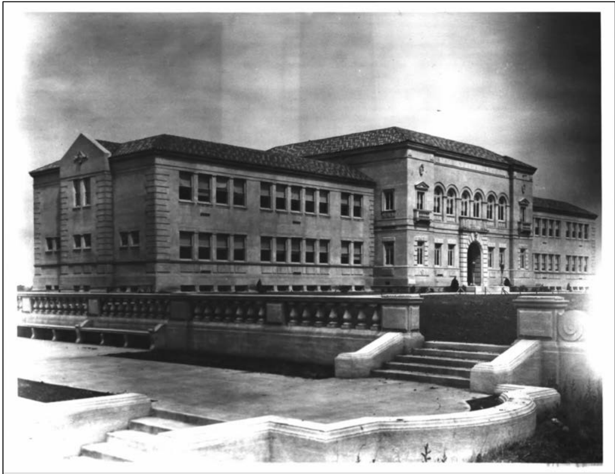
Figure 2. In 1929, Eastern Oregon Normal School (now Inlow Hall at 8th Street and K Avenue in La Grande) was founded to train teachers in the eastern part of the state. Source: Eastern Oregon Normal School NRHP nomination.
