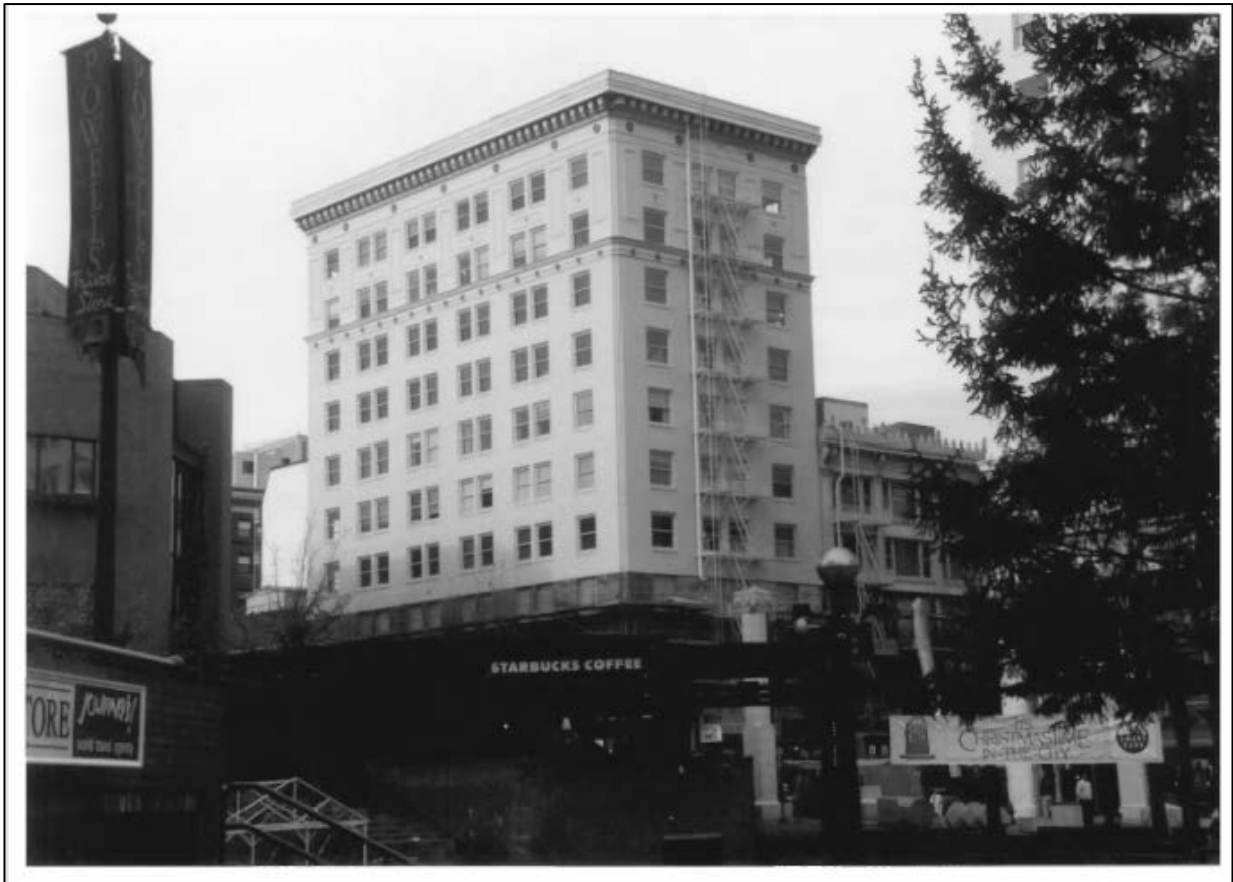
Figure 17. The Broadway Building (715 SW Morrison Street in Portland) is an example of a commercial building that housed many different businesses. Several abortion clinics, including Dr. Barnett's, were in this building during the early twentieth century. Source: Broadway Building NRHP nomination.
