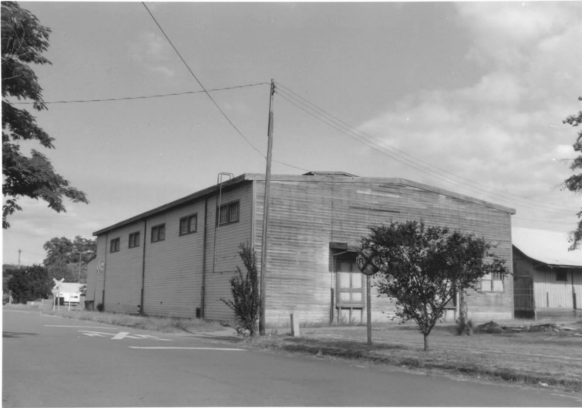
Figure 4. The hop warehouse at 2nd and D in the Independence Historic District in Polk County is an example of a functional utilitarian agriculture-related building. Source: Independence Historic District NRHP nomination.
