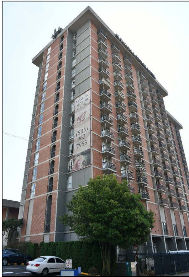
Photo 3 of 25: North and west elevations, camera facing southeast
