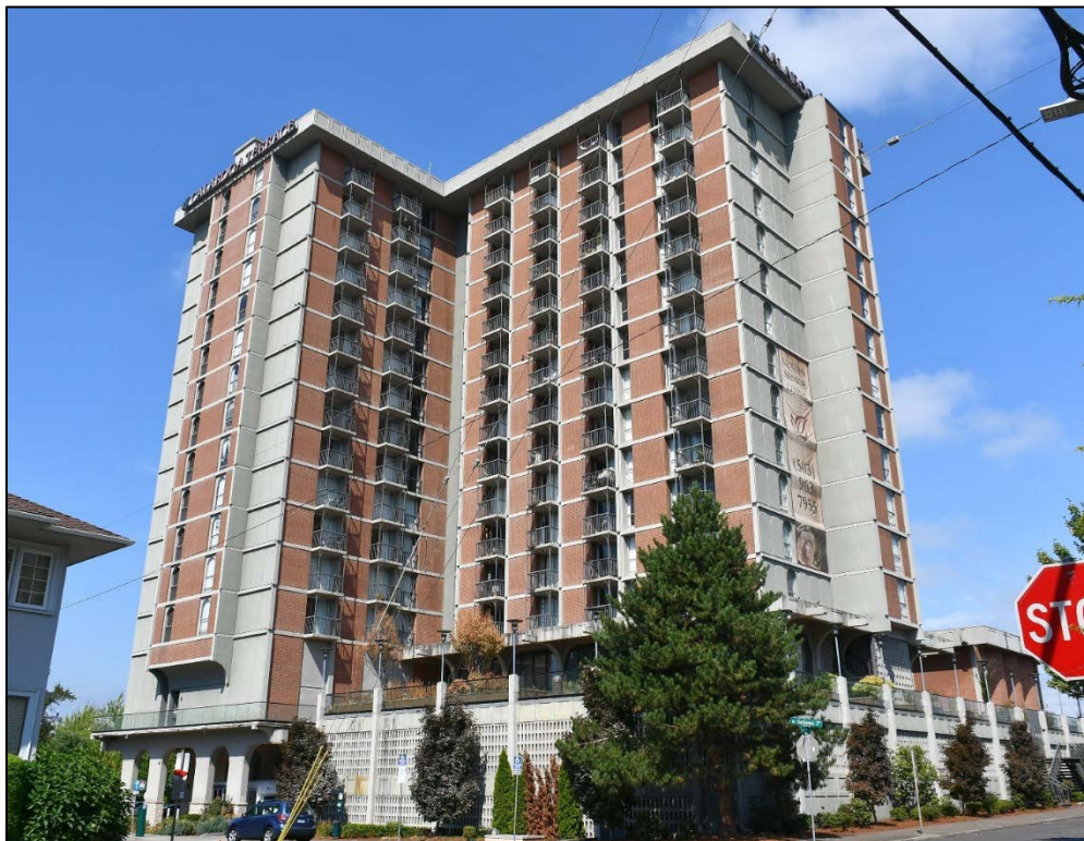
Photo 2 of 25: South elevation, camera facing northwest
