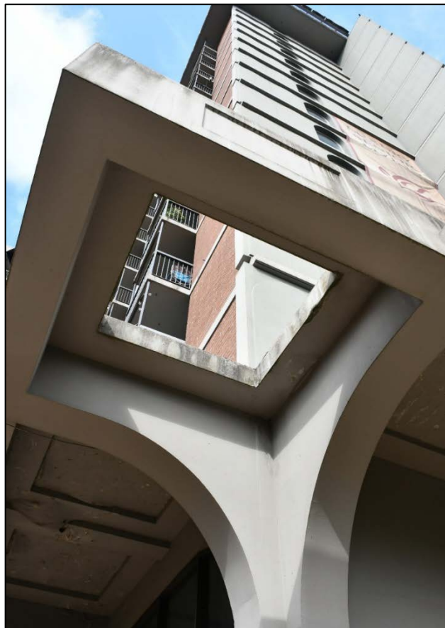
Photo 8 of 25: Architectural detail of arches and extruded panels from south terrace, camera looking up, facing northwest
