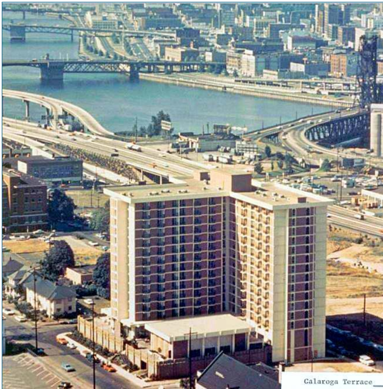
Figure 28: Aerial photograph of Calaroga Terrace nearing completion, July 1967. 193
