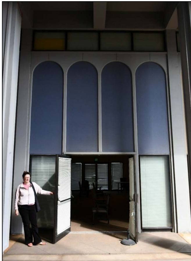
Photo 16 of 25: Multi-purpose room entrance from central terrace, camera facing north
