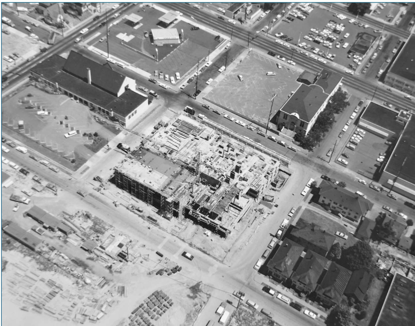
Figure 25: Aerial photograph of Calaroga Terrace under construction in 1966. 190
