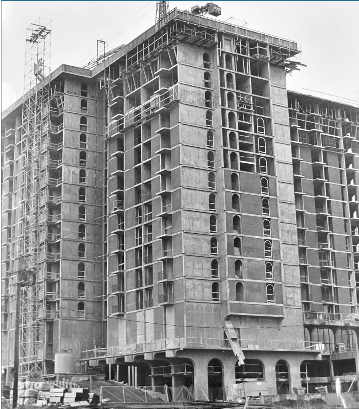
Figure 26: Calaroga Terrace under construction, December 1966. 191
