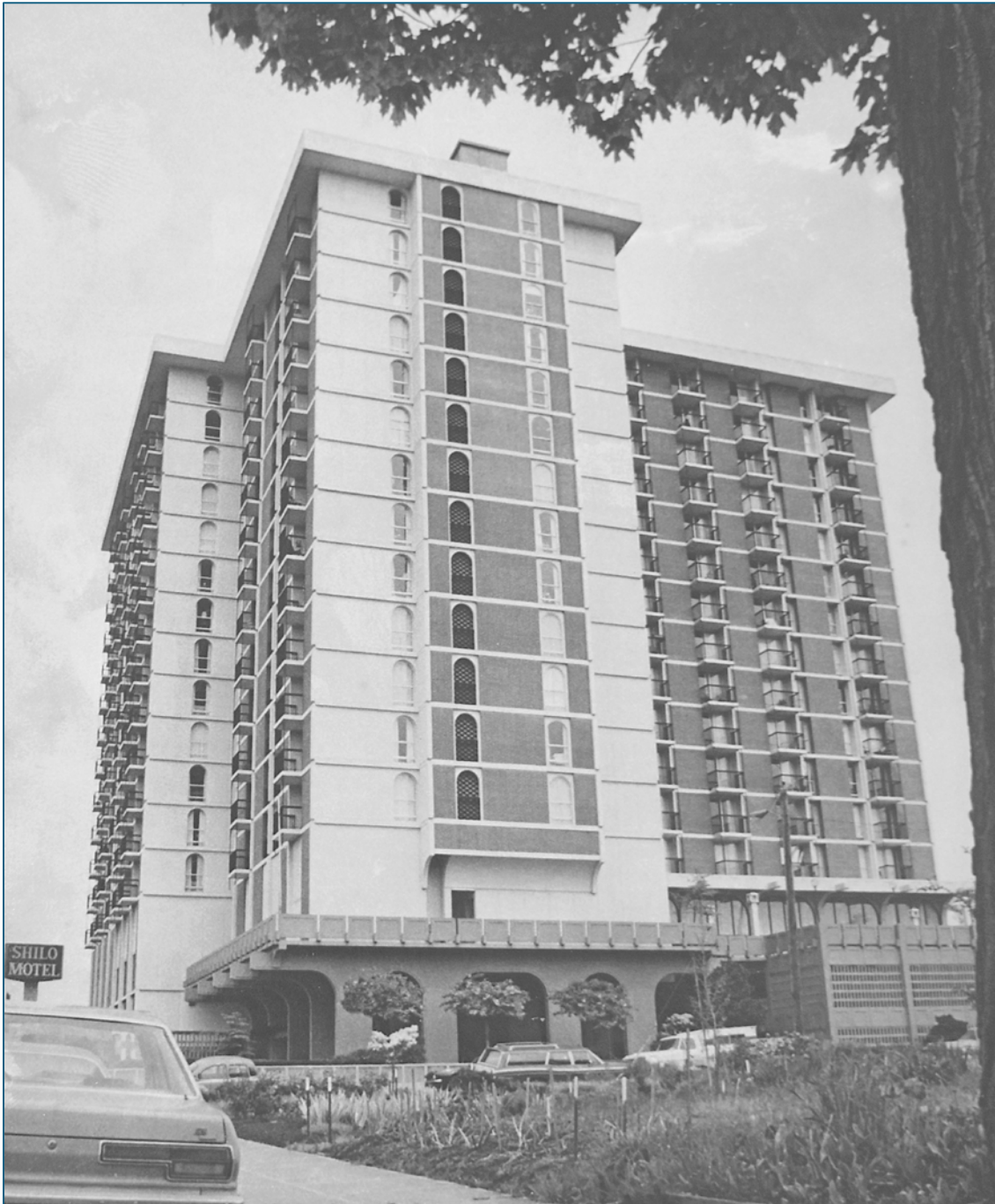
Figure 36: Photograph of Calaroga Terrace and the community garden in the foreground, 1978. 201
