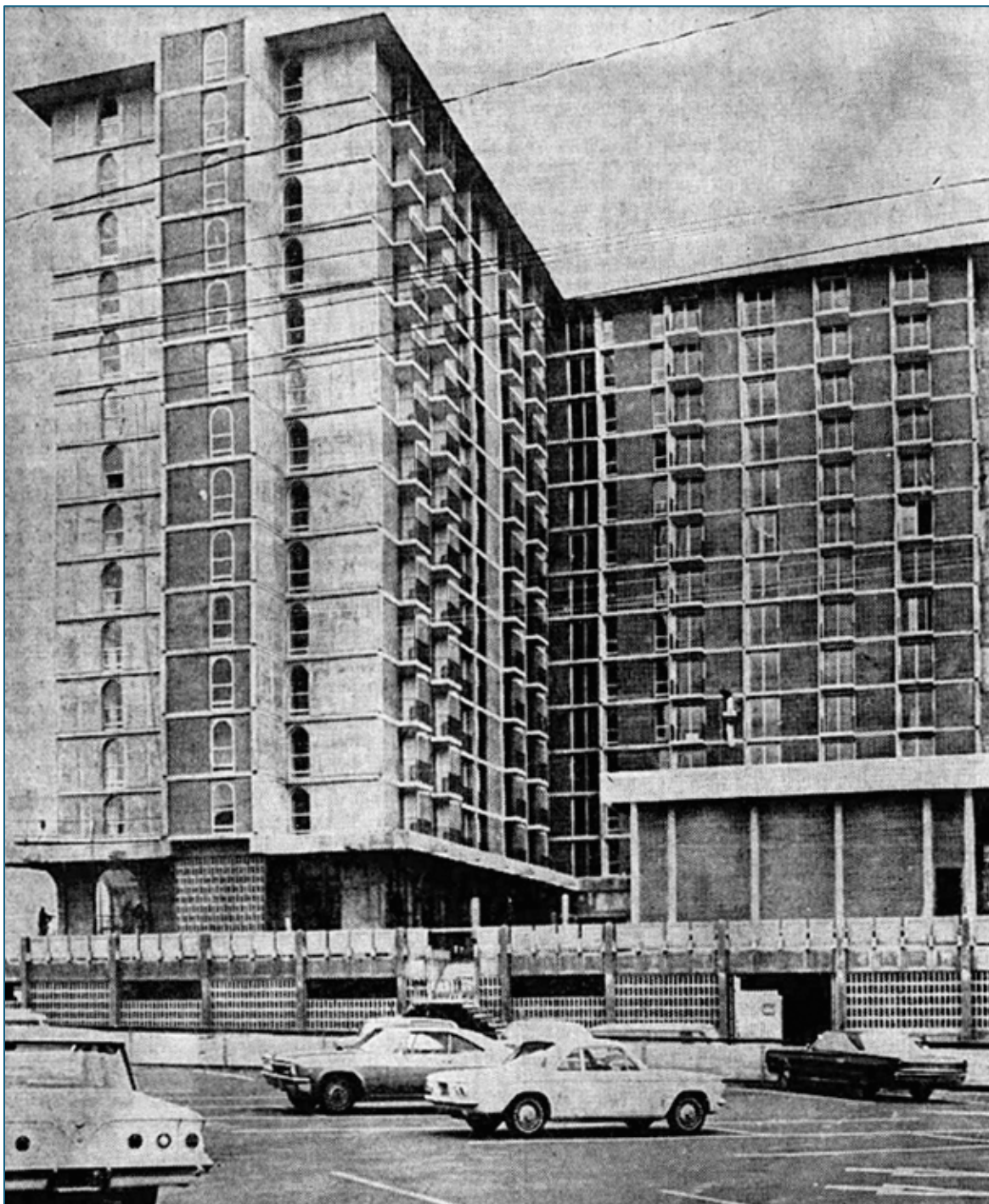
Figure 27: Construction of Calaroga Terrace approaching completion, March 1967. 192
