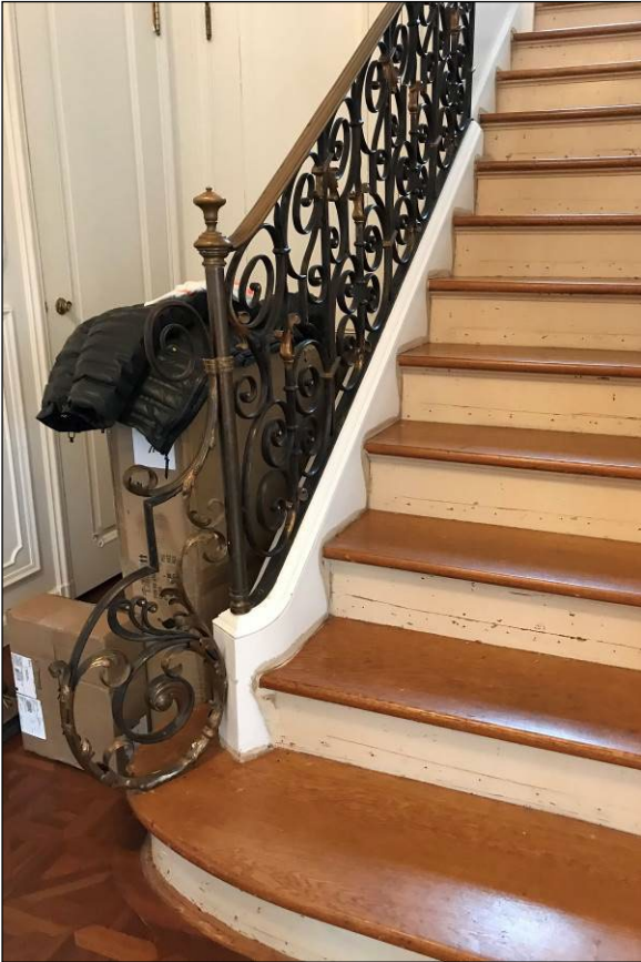
Photo 8 of 25: Stair looking northwest.
