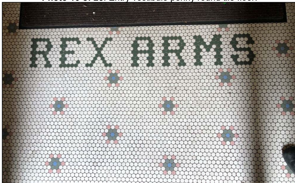
Photo 10 of 25: Entry vestibule penny round tile floor.
