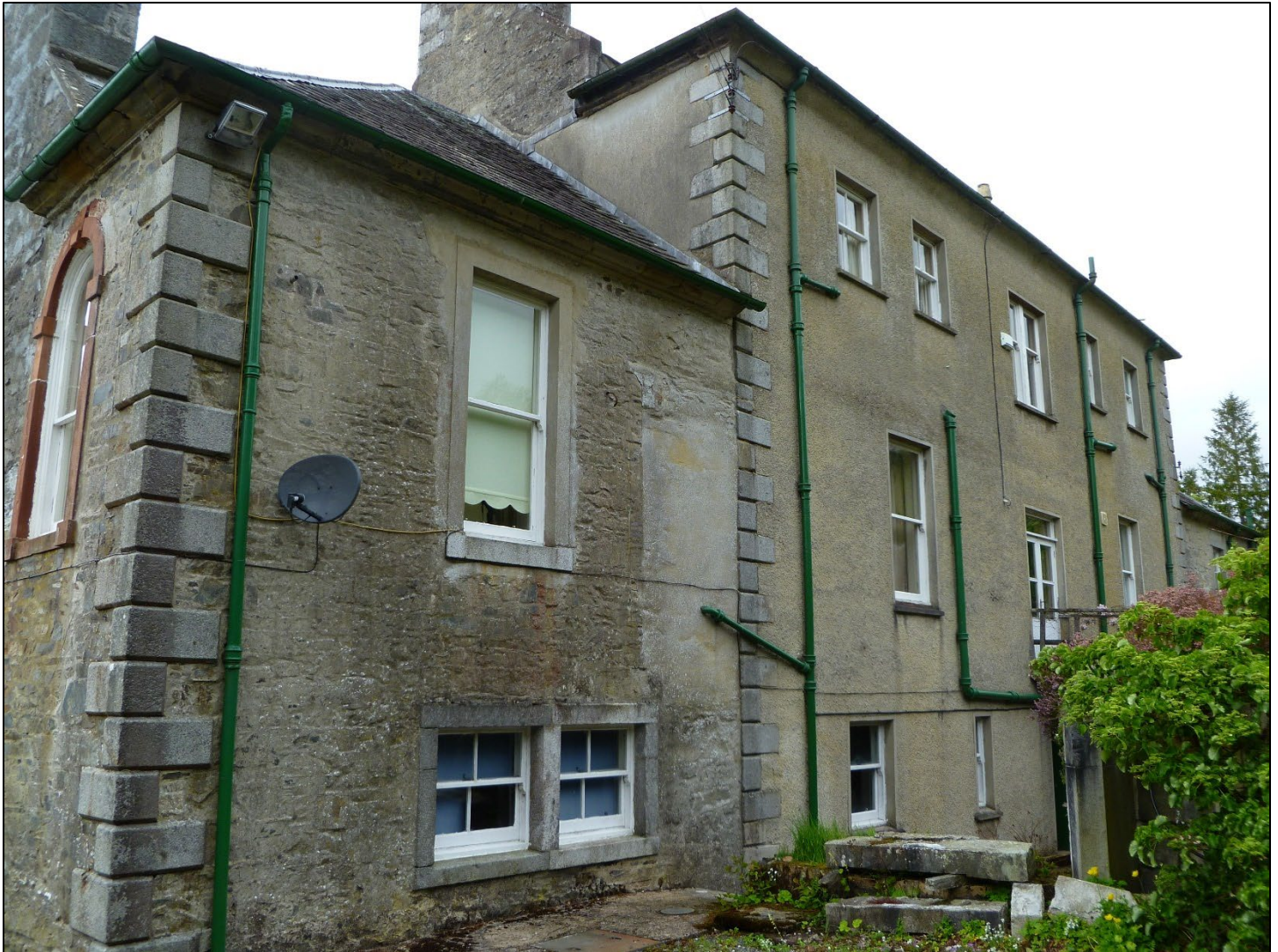
Figure 22: Stone houses with harling exterior, recessed windows, Newton Stewart, Scotland. Photo taken 2011, Eileen G. Fitzsimons.
