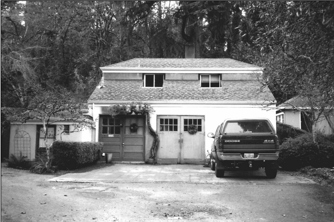
Photograph 7 of 18: OR_MultnomahCounty_KerrPeterandLaurieKingEstate_0007 East elevation of garage, camera facing west.
