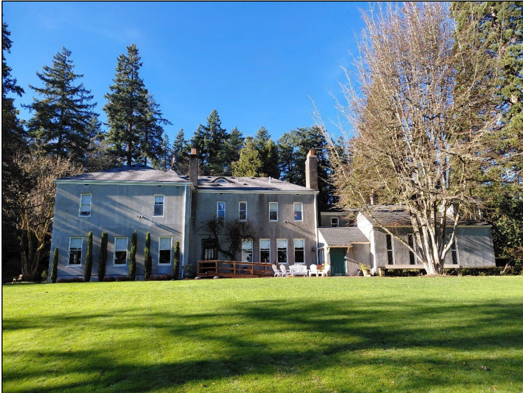
Photograph 5 of 18: OR_MultnomahCounty_KerrPeterandLaurieKingEstate_0005 East elevation of house, camera facing west.
