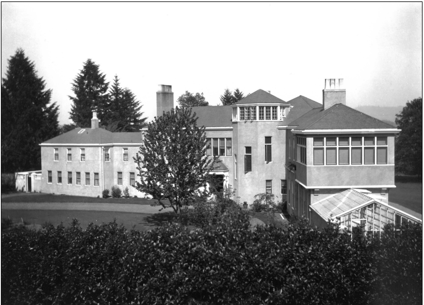
Figure 25: West façade (main entry) of Kerr house, looking east, ca. 1922. Kerr family collection, Coll 74, Box 4, folder 13, neg.1650, Oregon Historical Society Research Library.
