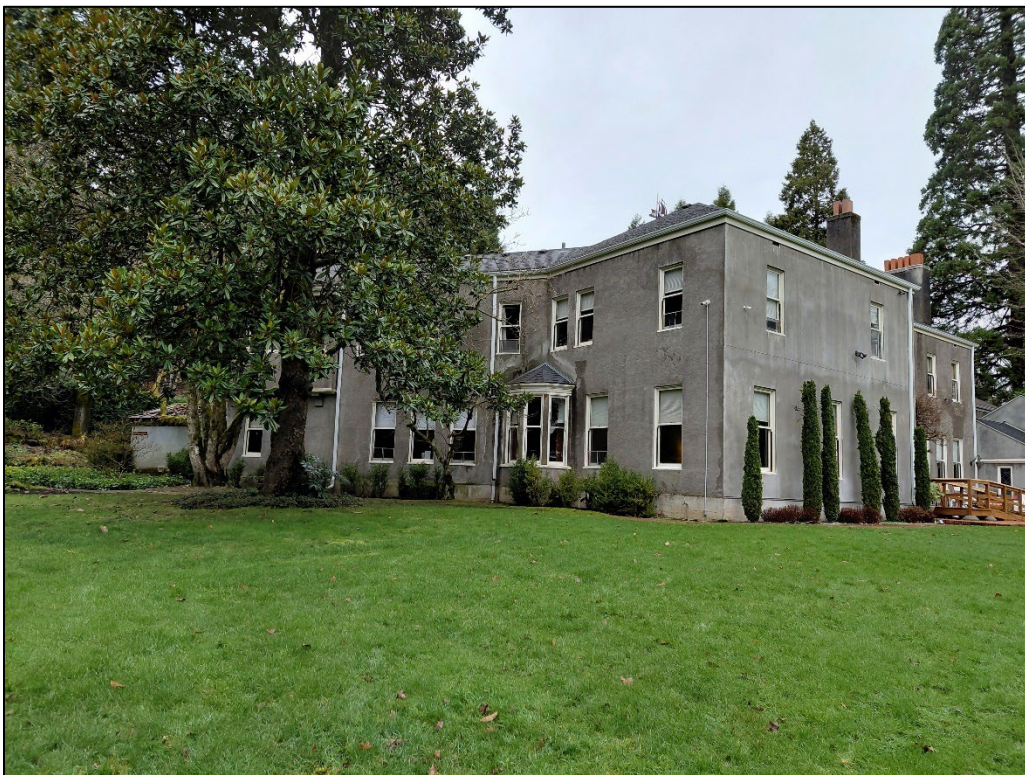
Photograph 6 of 18: OR_MultnomahCounty_KerrPeterandLaurieKingEstate_0006 South elevation of house, camera facing northwest.
