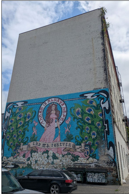
Photograph 5 of 15: OR_MultnomahCounty_OregonCasketCompanyBuilding_0005 West elevation, camera facing east.
