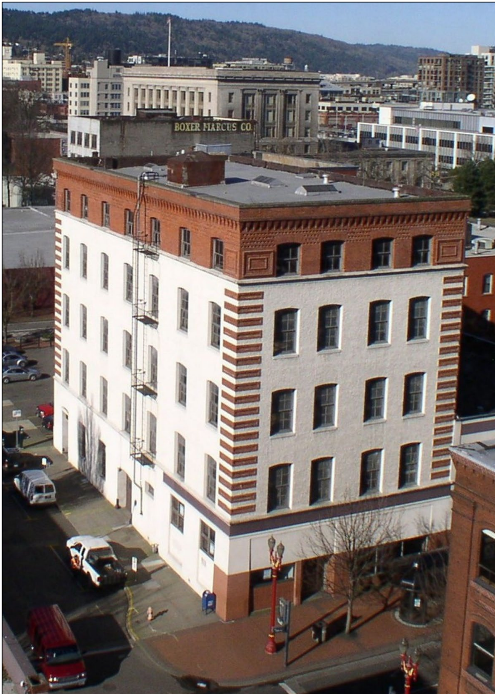
Figure 24: A c. 2006 bird's-eye view of the south and east elevations of the Oregon Casket Company Building, camera facing northwest. 131
