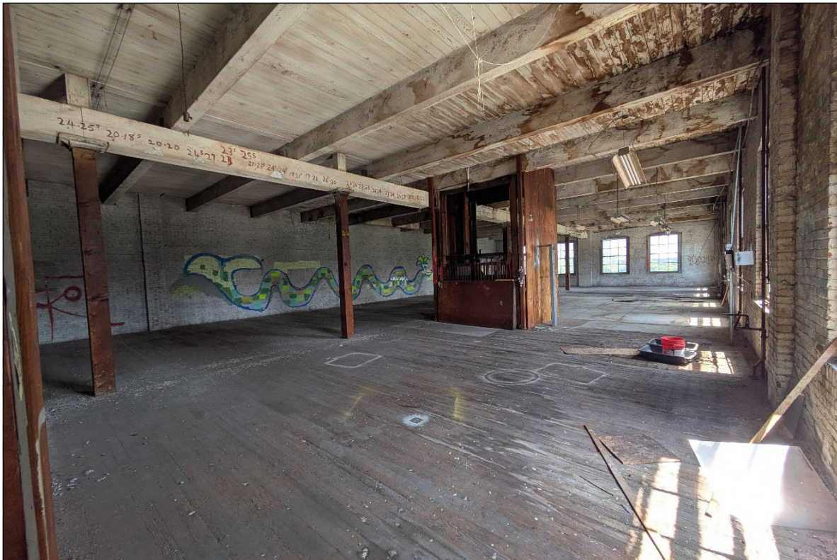
Photograph 13 of 15: OR_MultnomahCounty_OregonCasketCompanyBuilding_0013 Fourth floor showing elevator at middle; taken from door to stairs; camera facing northeast.
