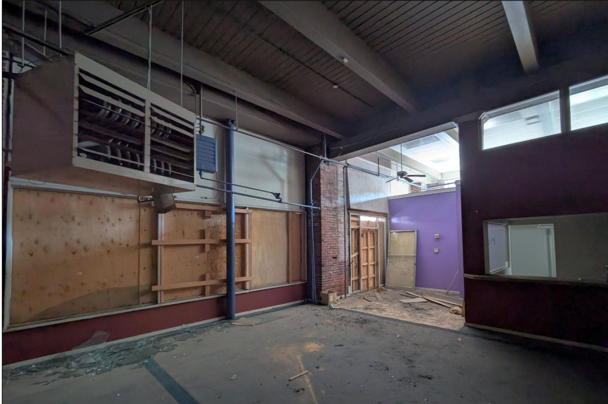
Photograph 8 of 15: OR_MultnomahCounty_OregonCasketCompanyBuilding_0008 Eastern portion of ground floor; camera facing southeast.
