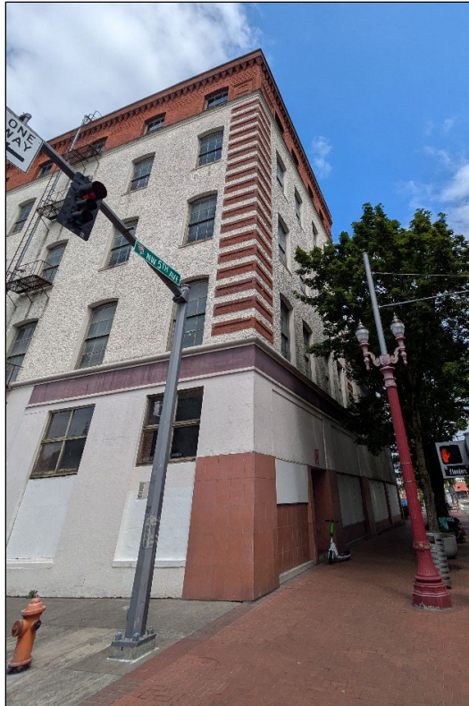
Photograph 1 of 15: OR_MultnomahCounty_OregonCasketCompanyBuilding_0001 South and east elevations; camera facing northwest.
