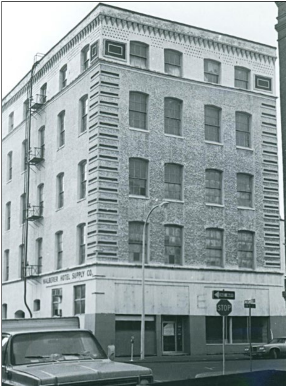
Figure 18: May 1980 photograph showing the east and south elevations of the Oregon Casket Company Building. 125
