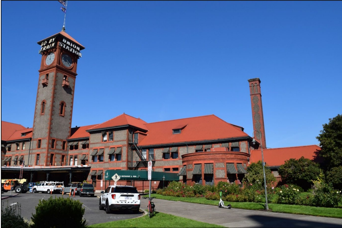
Photograph 1 of 18: OR_MultnomahCounty_UnionStationAmendment_0001 Clock tower, south wing, and front yard; looking north.
