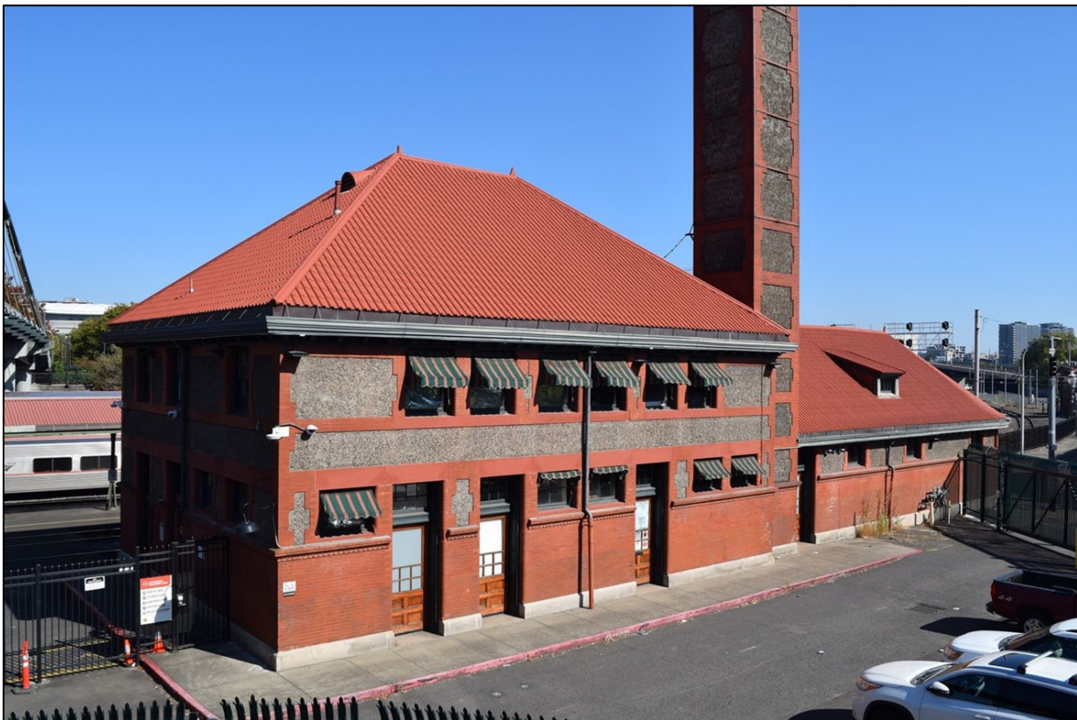
Photograph 8 of 18: OR_MultnomahCounty_UnionStationAmendment_0008 Annex northwest and southwest façades, looking east.
