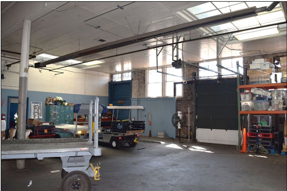
Photograph 14 of 18: OR_MultnomahCounty_UnionStationAmendment_0014 Interior of baggage handling room, looking south.
