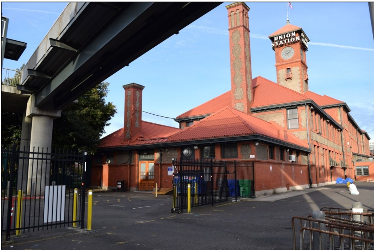
Photograph 4 of 18: OR_MultnomahCounty_UnionStationAmendment_0004 ] Southeast end of Primary Terminal; looking north.
