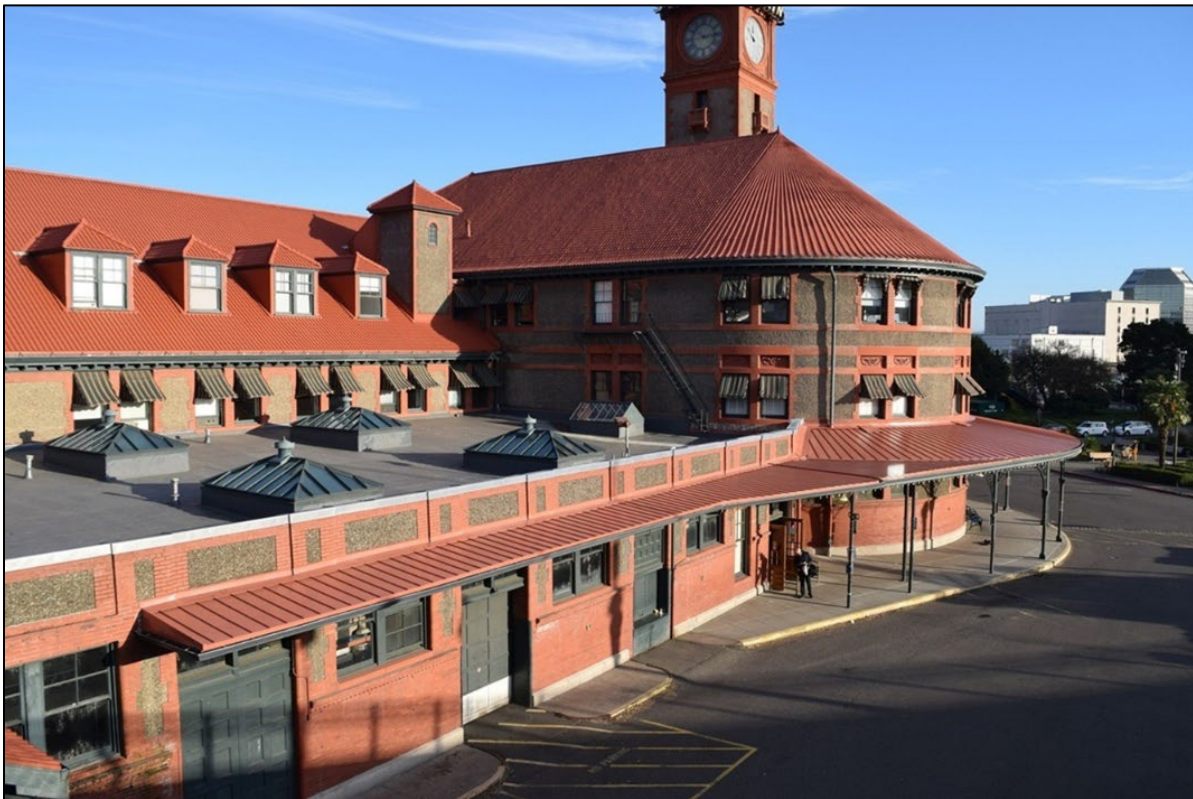
Photograph 2 of 18: OR_MultnomahCounty_UnionStationAmendment_0002 North wing on left and Main hall, looking southeast.
