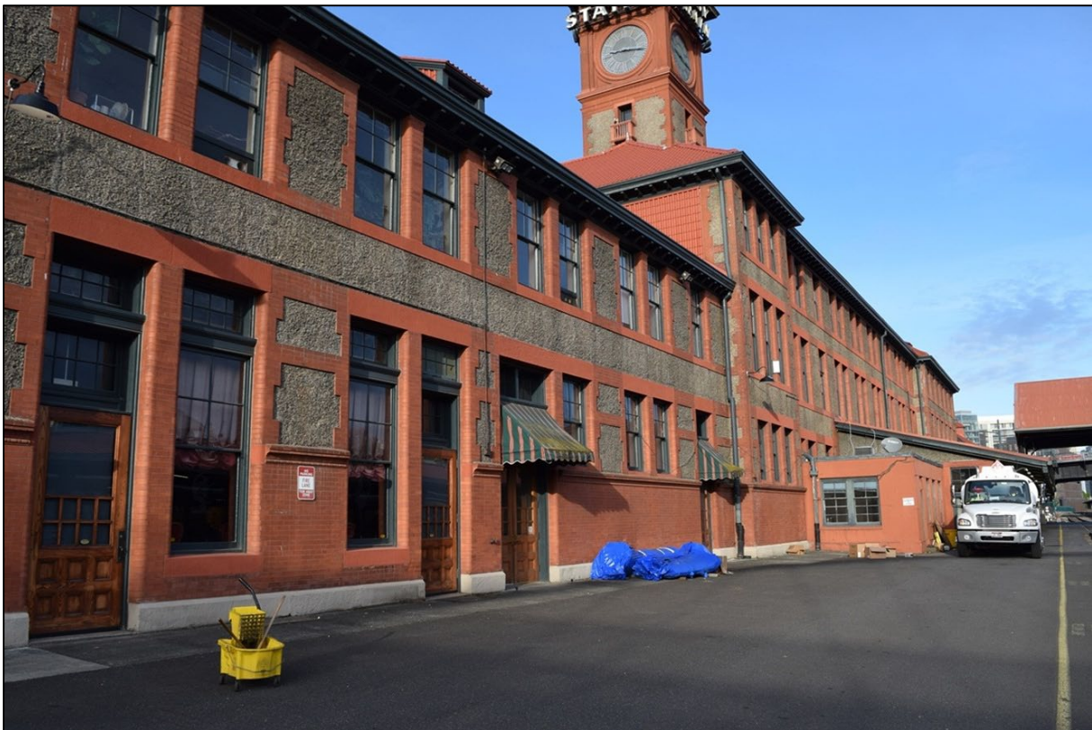
Photograph 6 of 18: OR_MultnomahCounty_UnionStationAmendment_0006 Northeast façade and Nursery addition, looking east.
