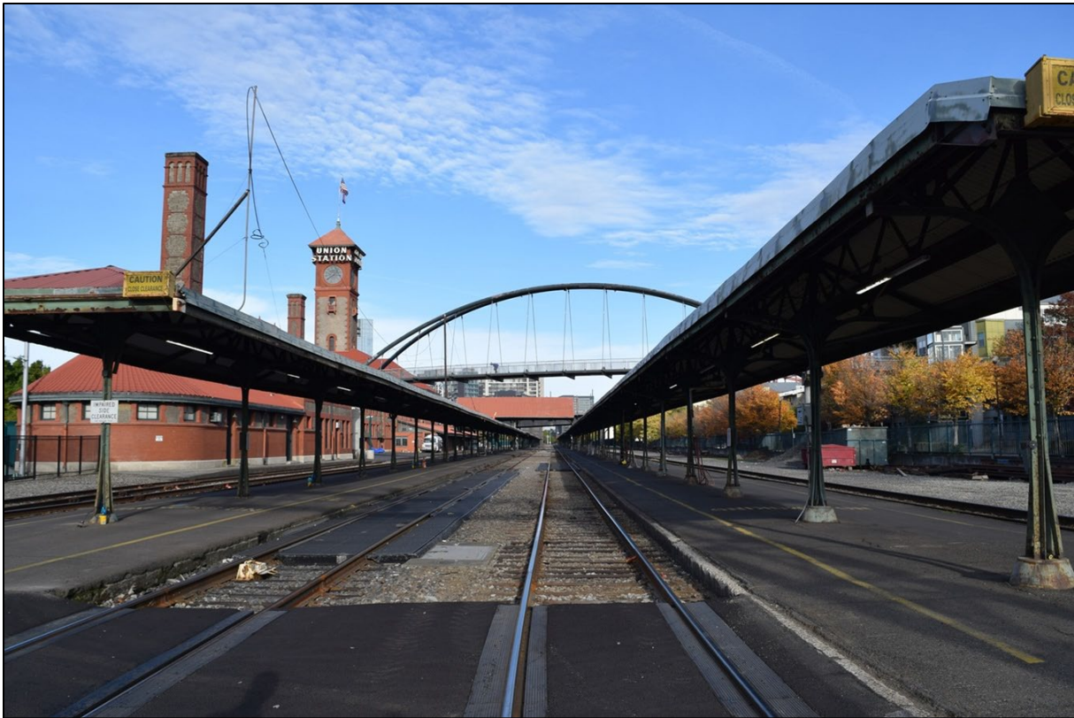
Photograph 5 of 18: OR_MultnomahCounty_UnionStationAmendment_0005 Southeast end of Annex on left, Platform Canopy 1 on left; looking northwest.
