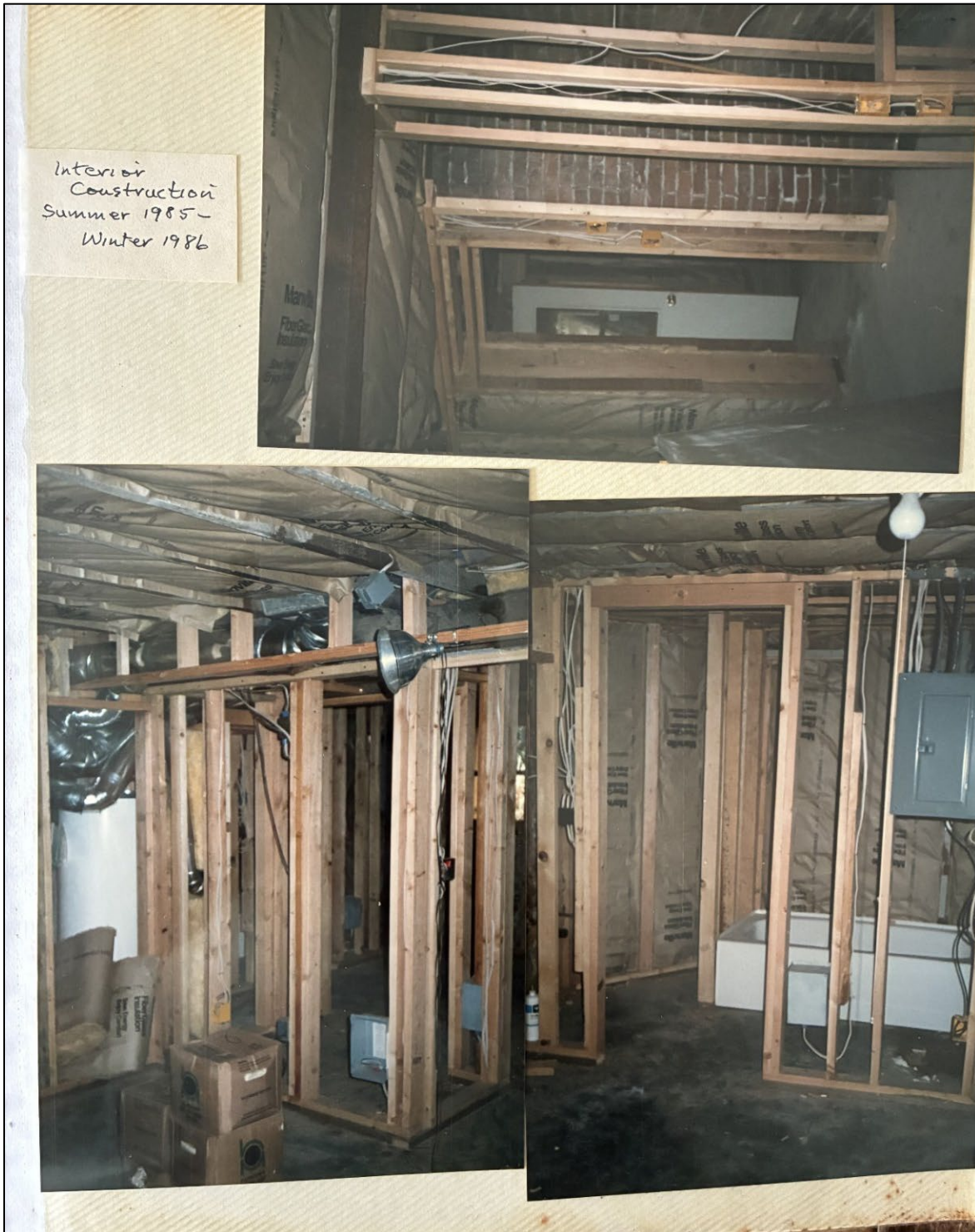
Figure 18: Basement apartment unit construction photos, 1985-86. Source: Le Guin Family Collection.
