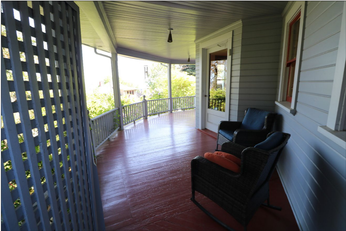
Photograph 7 of 18: OR_MultnomahCounty_LeGuinUrsulaKHouse_0007 North Elevation, Covered Porch, view looking east.
