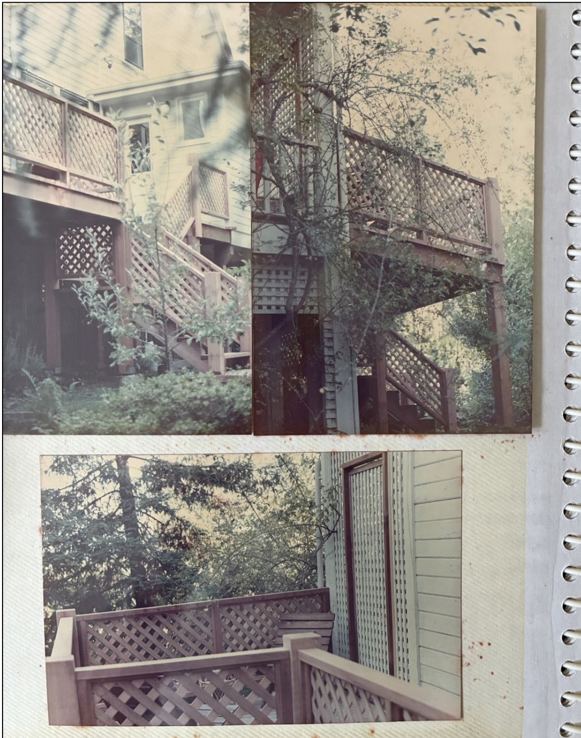
Figure 15: Construction photos showing new Laundry Room Addition and deck, 1984. Views looking at west elevation. Source: Le Guin Family Collection.
