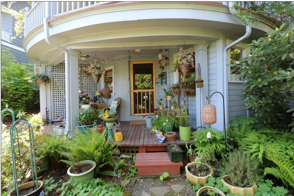
Photograph 6 of 18: OR_MultnomahCounty_LeGuinUrsulaKHouse_0006 North Elevation, view looking south towards apartment unit entry.
