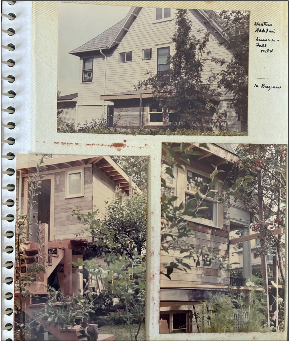
Figure 12: Construction photos showing 1984 Laundry Room Addition. View looking northeast at west elevation. Source: Le Guin Family Collection
