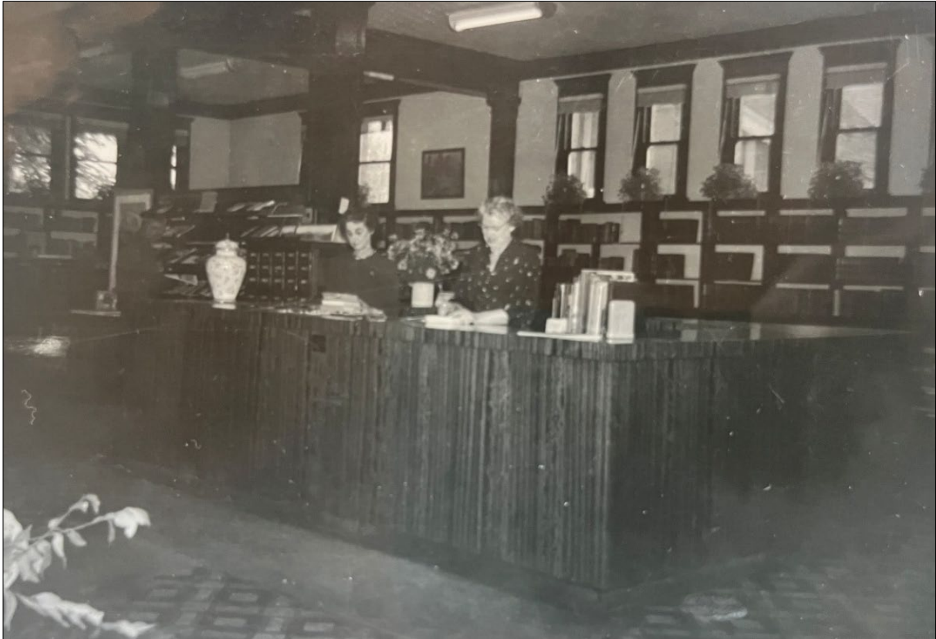
Figure 12: Library interior showing replacement circulation desk, c1960 (La Grande Public Library Collection).
