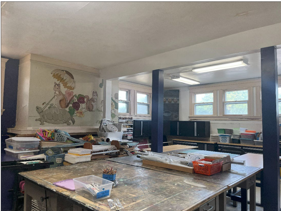
Photograph 10 of 10: OR_UnionCounty_LaGrandeCarnegieLibrary_0010 View of former children's room at basement level, looking northwest, September 5, 2025.
