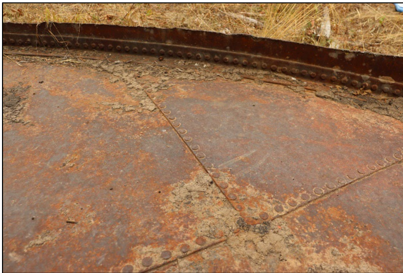
Photo 10 of 18. Detail of the rivets and bitumen lining of the Structure 1 water tank, September 2022. Maxville Heritage Interpretive Center.
