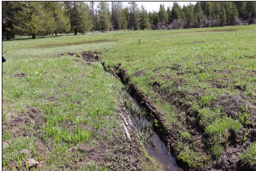
Photo 14 of 18. A portion of Contributing Structure, Structure 5 ,view south-southeast, May 2022. This is a portion of Maxville's water system, showing an excavated trench reinforced by large pieces of milled lumber and containing a cast iron ferrous metal pipe. Maxville Heritage Interpretive Center.
