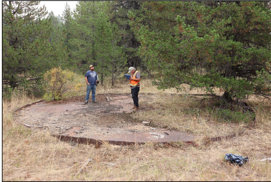
Photo 9 of 18. Contributing Structure, Structure 1, view east, September 2022. Structure 6 is the base of a cast iron and rivetted water tank located in the industrial area of the Maxville District. Maxville Heritage Interpretive Center.
