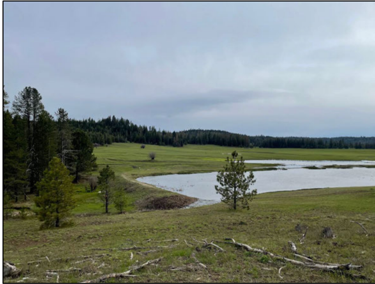
Photo 15 of 17. Contributing Structure 6, view south, June 2022. Structure 11 is an earthen dam on Bishop Creek that creates a log holding pond used during the Maxville operations.
