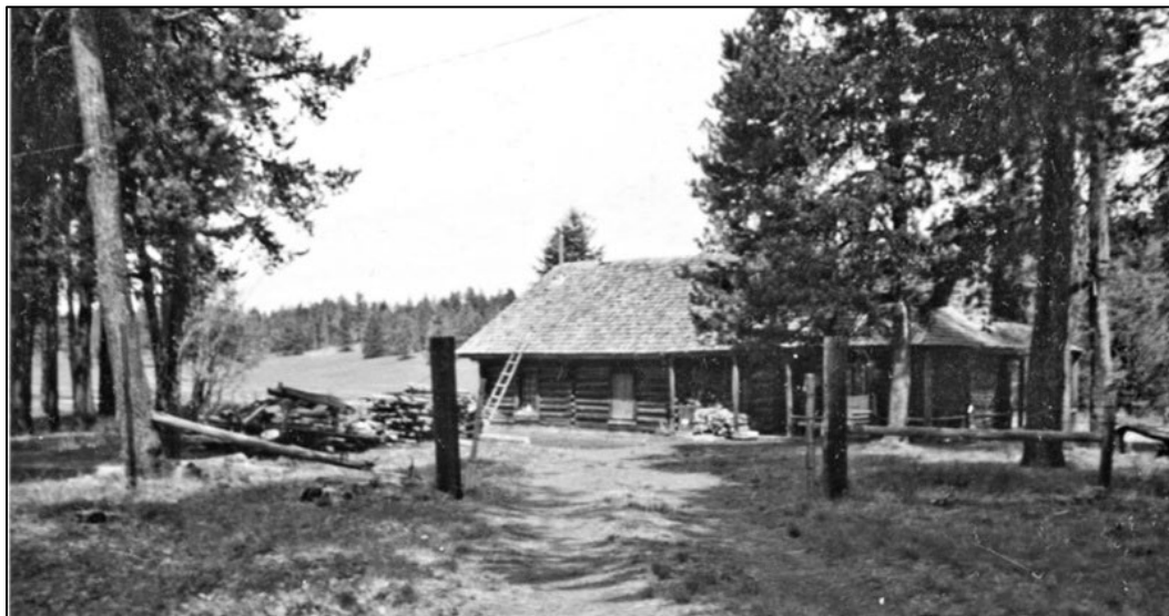
Figure 17. The Maxville Superintendent's Lodge, 1923. View west-northwest. Maxville Heritage Interpretive Center.
