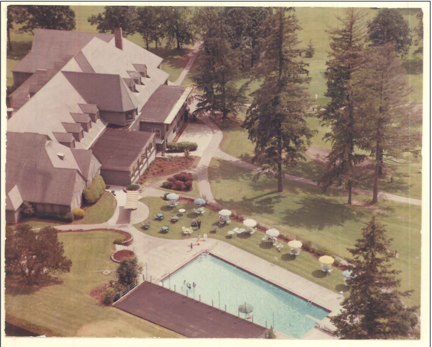
Figure 11: 1966 Aerial Photograph of the Clubhouse from the Southwest
