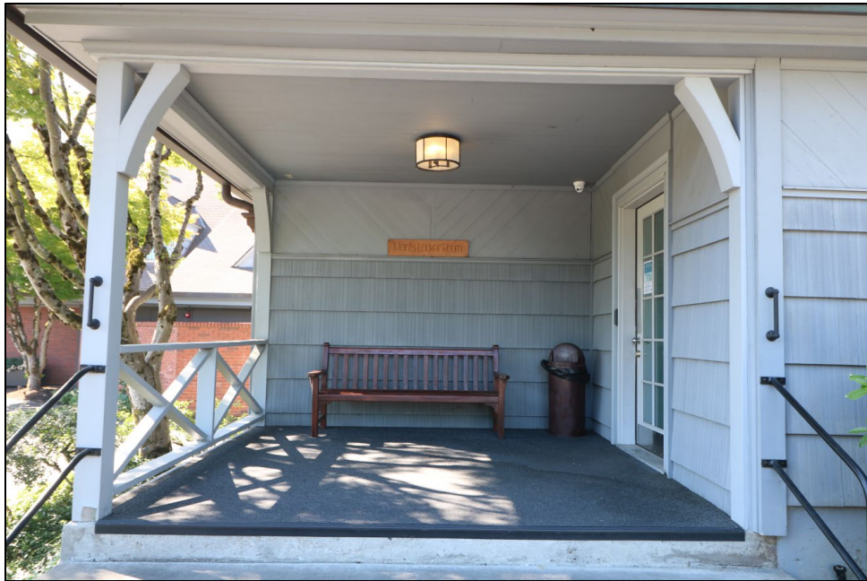
Photo 7. Portland Golf Club Clubhouse, North Elevation, view looking south.
