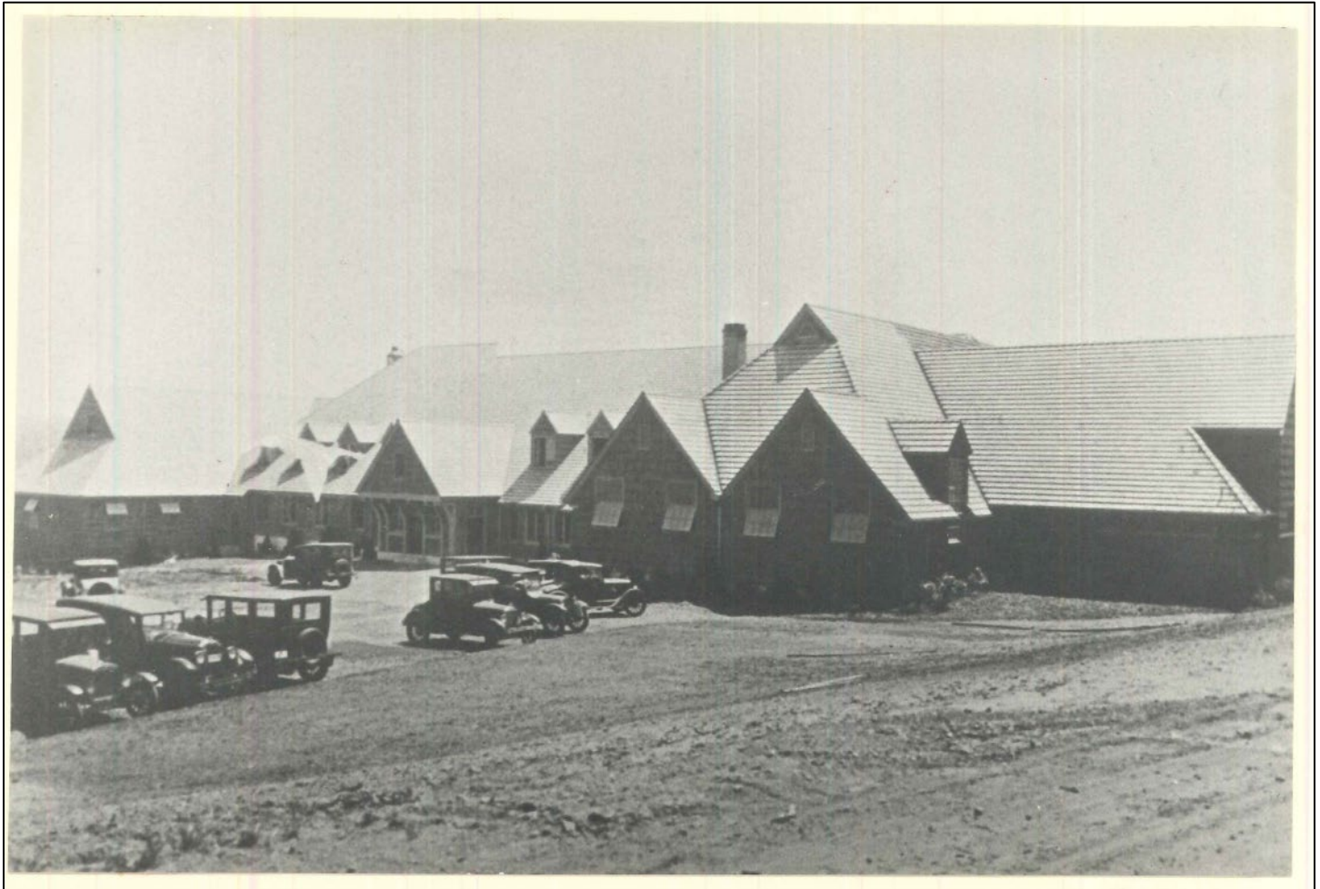
Figure 8: Photograph of the Clubhouse Shortly After Construction Looking Southwest at the North Elevation
