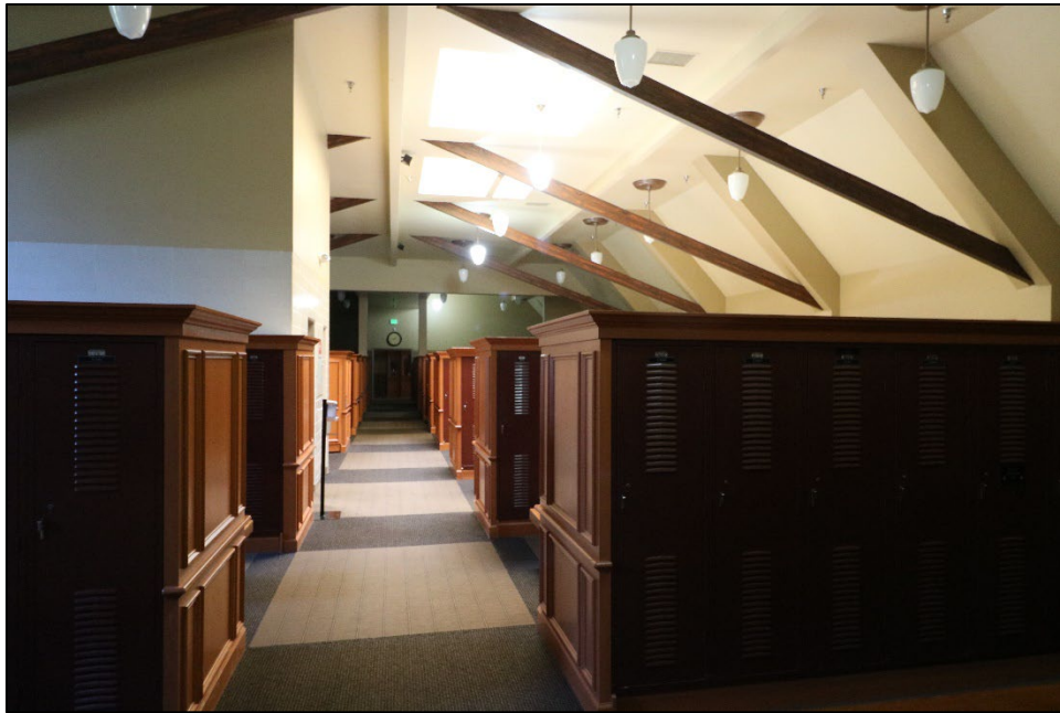
Photo 21. Portland Golf Club Clubhouse, First Floor, Men's Locker Room, view looking north.
