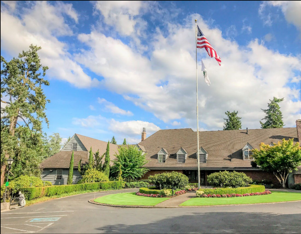
Photo 2. Portland Golf Club Clubhouse, North Elevation, view looking south.
