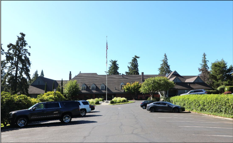
Photo 1. Portland Golf Club Clubhouse, North Elevation, view looking south.
