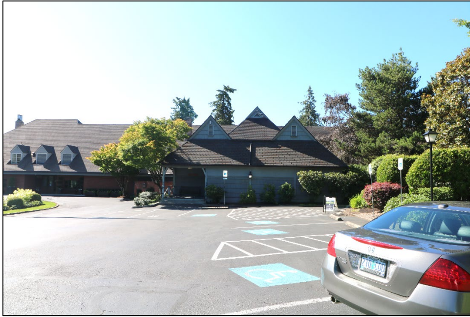
Photo 3. Portland Golf Club Clubhouse, North Elevation, view looking south.
