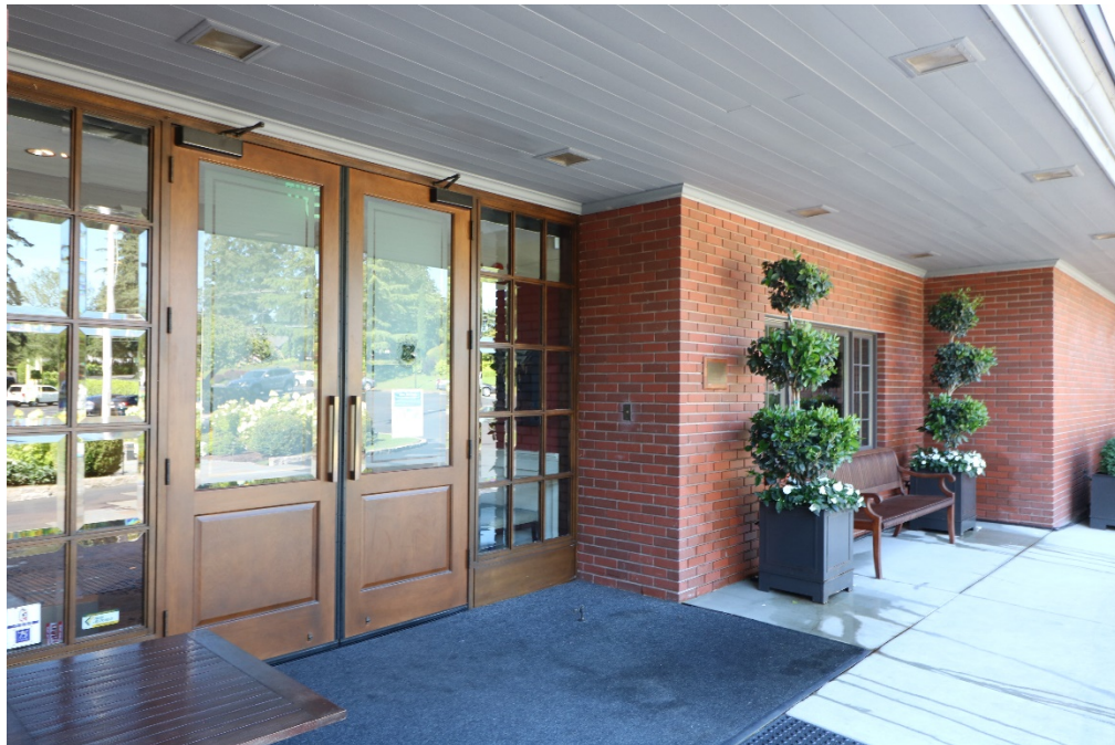
Photo 4. Portland Golf Club Clubhouse, North Elevation, view looking northeast.
