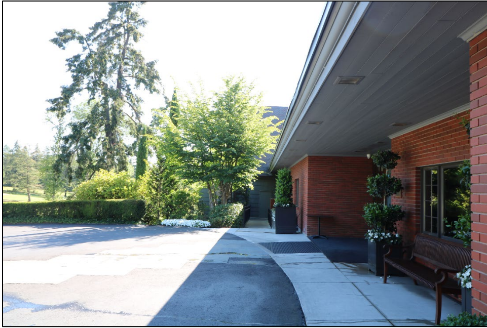
Photo 5. Portland Golf Club Clubhouse, North Elevation, view looking northeast.
