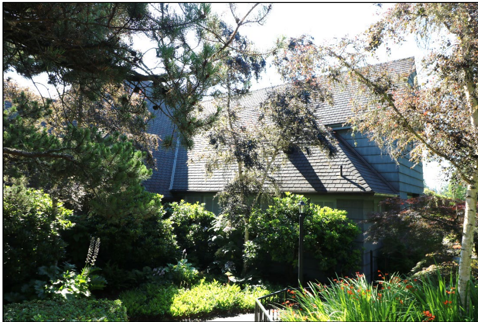
Photo 8. Portland Golf Club Clubhouse, West Elevation, view looking east.
