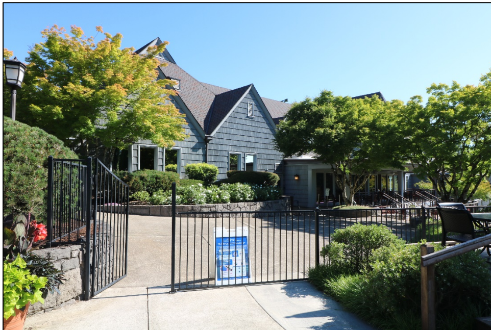
Photo 10. Portland Golf Club Clubhouse, South Elevation, view looking east.
