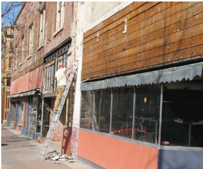
Elmira Arts Project in downtown Ellensburg.
