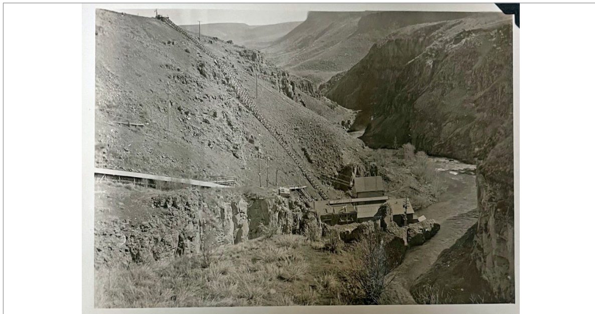
Fig. 37. Ca. 1912 powerhouse photograph. Looking southeast showing the north addition under construction. Source: OPRD.
