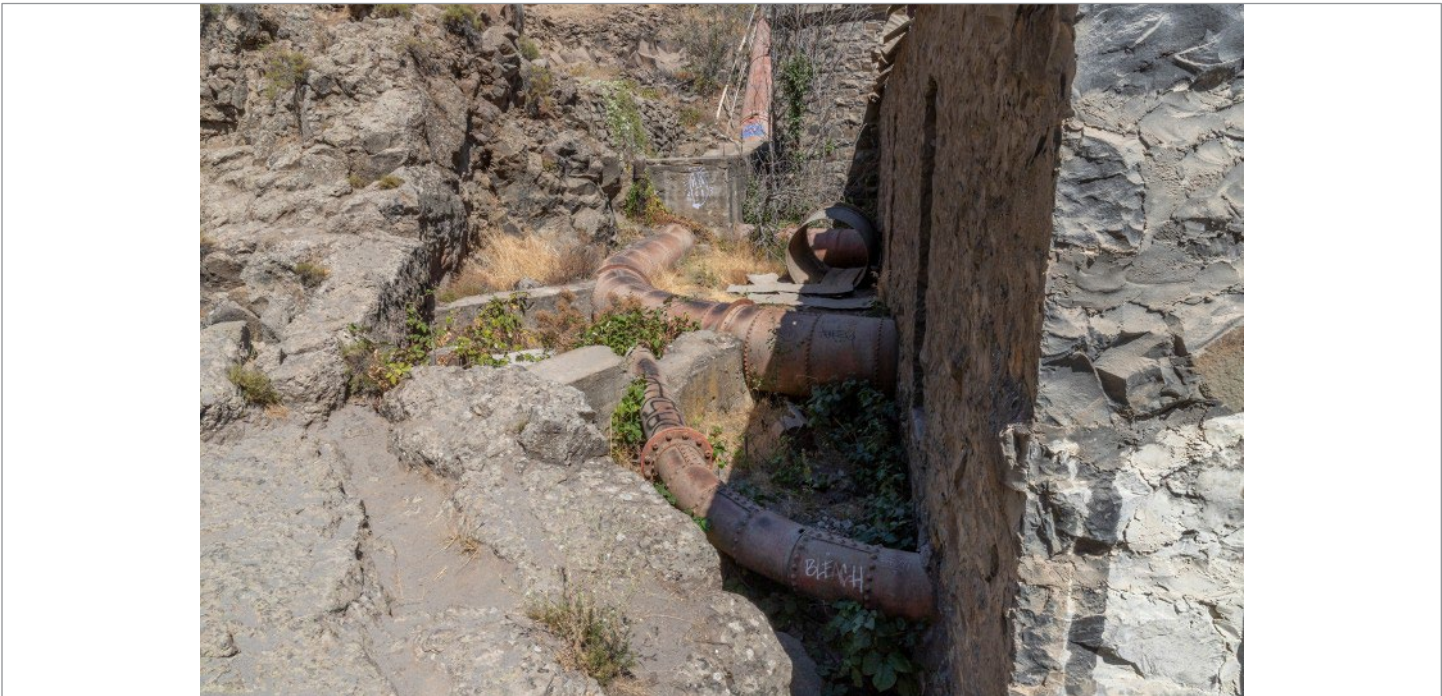
OR_Wasco County_Wasco Warehouse & Milling Company Hydroelectric Project Historic District_0024. Steel penstock connect to powerhouse, looking north.
