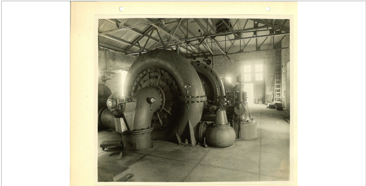
Fig. 32. 1921 penstock connection photograph. Looking north showing the 1911 penstock connection to the powerhouse. Source: OPRD.
