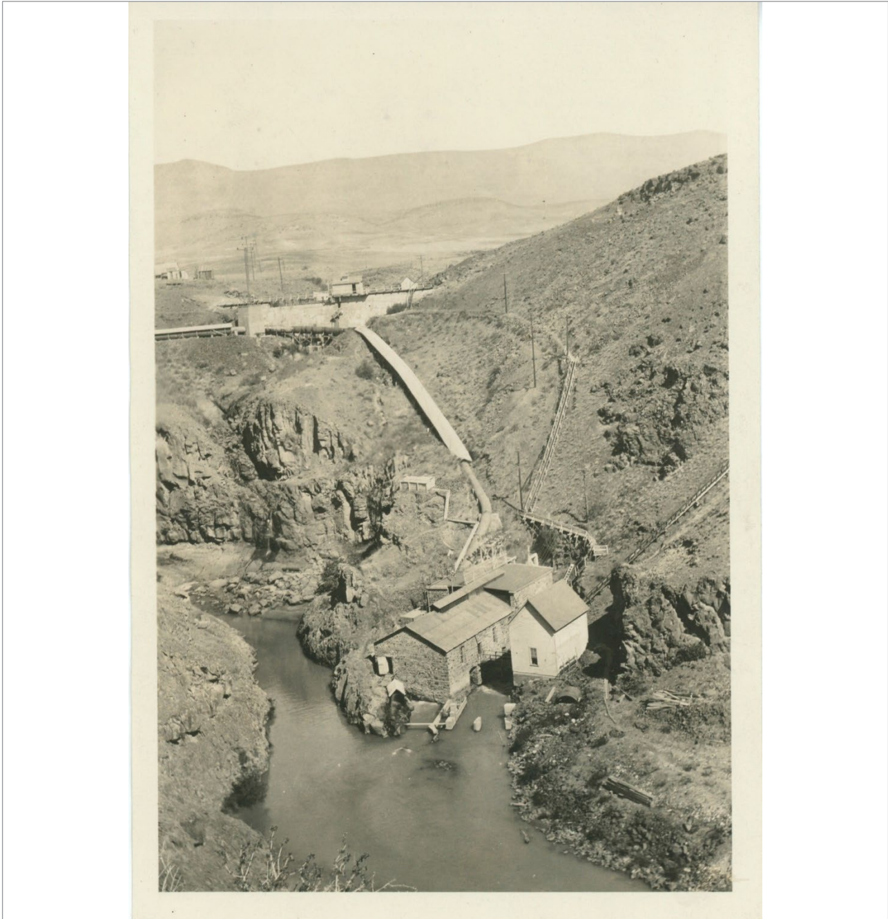
Fig. 38. Ca. 1934 system photograph. Looking north with the valve house at the west end of the reservoir completed. Source: OPRD.
