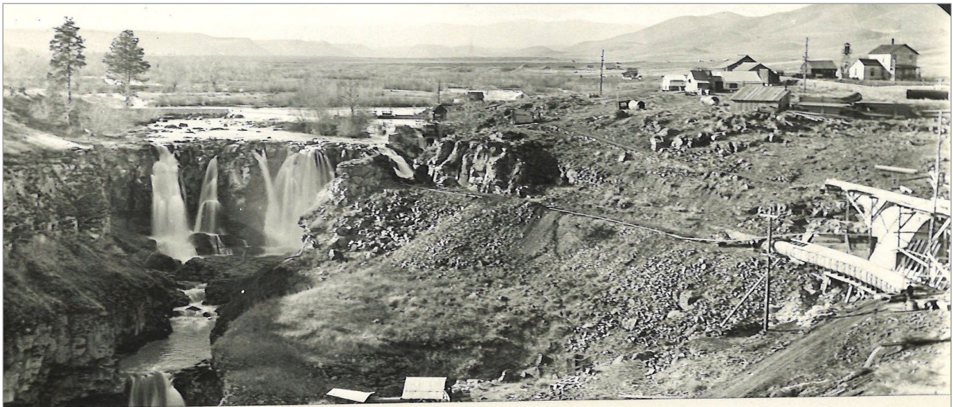
Fig. 25. Ca. 1901 headrace photograph. East end of the masonry headrace canal and the original penstock continuing east into the tunnel in the canyon wall prior to construction of the holding basin and reservoir dams. Source OPRD.
