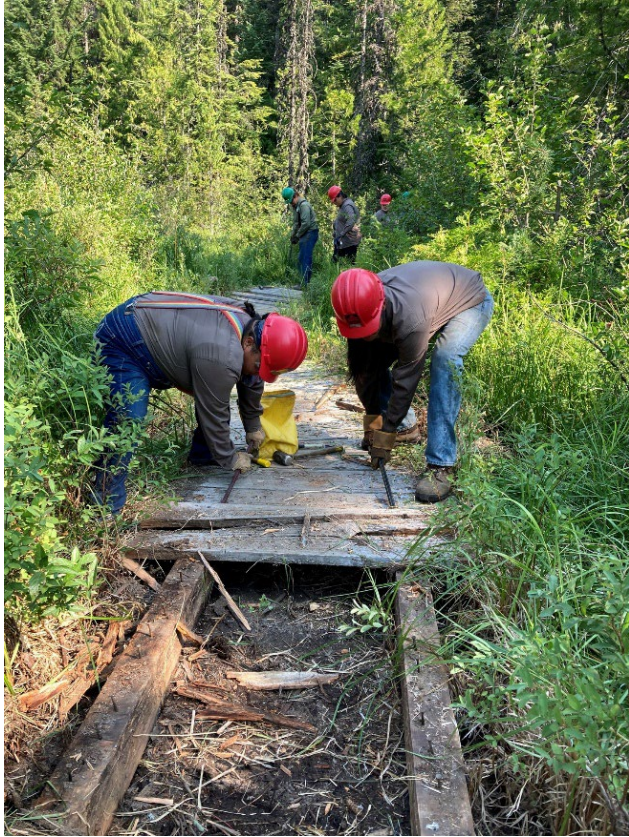
Photos: Trail crew removing old boardwalk and replacing with accessible boardwalk (Northwest Youth Corp (left), OPRD (right))
