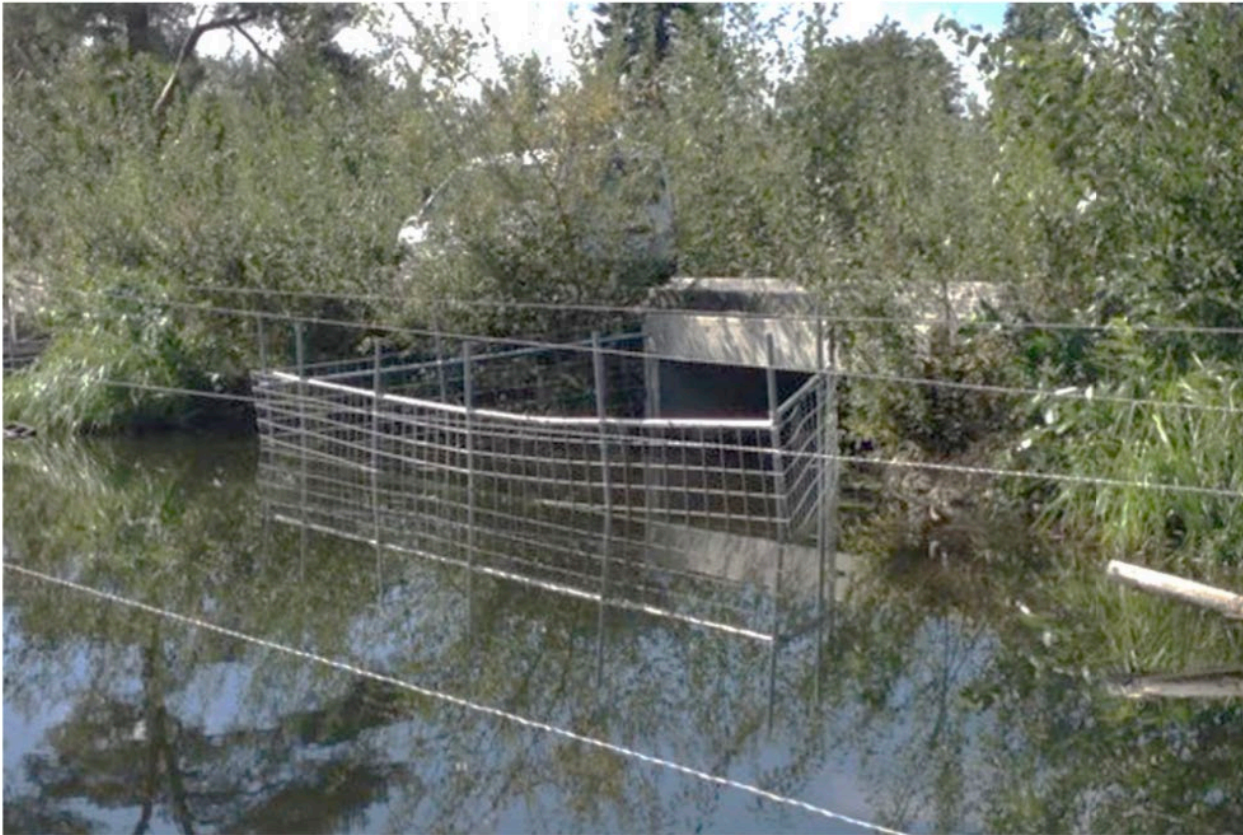
Figure 3. King County example: trapezoidal aquatic exclusionary fencing on box culvert inlet at Lower Stensland Creek.
