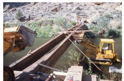
Bridge reconstruction, circa 1990.
