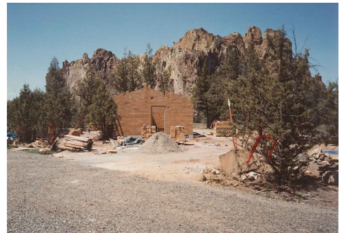
Restroom construction, circa 1990.
