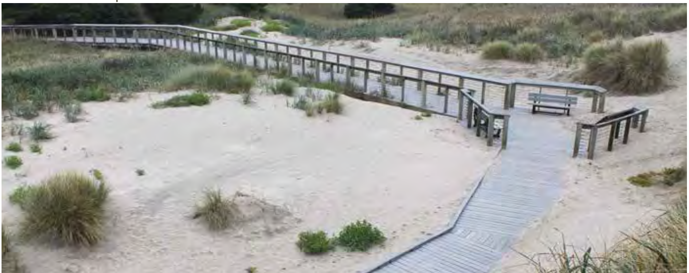
An accessible interpretive boardwalk was constructed in 2006 at South Beach State Park
