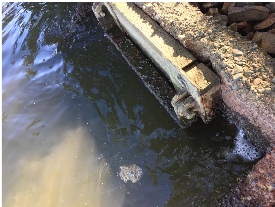
Closed tide gate at the outside of Beltz Dike, 2/12/2018.
