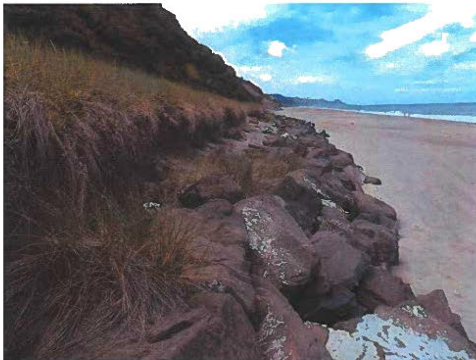
Photo 22 – View of the revetment near the southern extent of the site. Note the erosion above and behind the top of the revetment indicating previous overtopping of the revetment. (Photo taken 07/06/2018)
