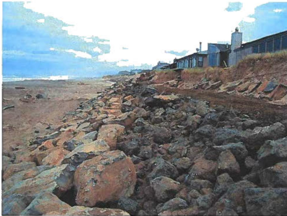
Photo 9 – Northerly view of the revetment fronting Tax Lot 218, Map 08-11-03CC during permitted repair work. Note the single layer of armor stone and lack of filter fabric backing the revetment. Photo taken by HGSA on 05/21/2016.
