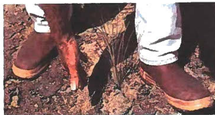
A beachgrass hand-planting operation includes (a) opening a 12-inch-deep hole in wet sand with a tile spade, (b) placing a beachgrass propagule in the hole and leaving an 8-inch top, and (c) tamping sand around the propagule with the heel of a boot.
