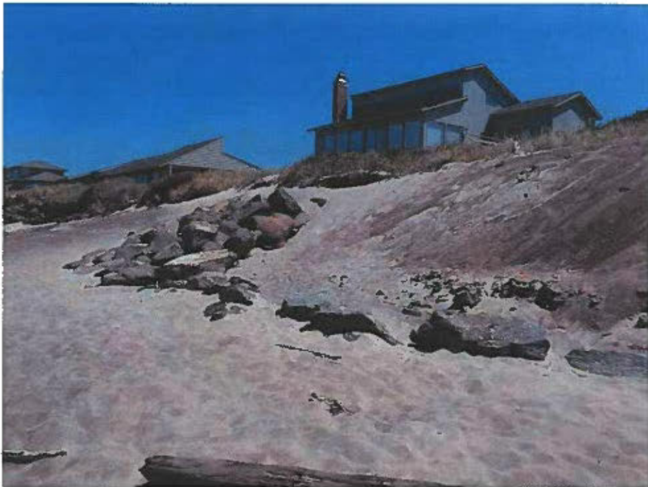
Photo 12 – View of the revetments fronting the beach in the area of Tax Lot 700, Map 08-11-03CB where the rock quality improves. Reconstruction of revetments occurred between Tax Lot 700, Map 08-11-03CB and Tax lot 204, Map 08-11-03CC to the south after severe erosion along this stretch of beach in 2016. (Also see Appendix A-2)
