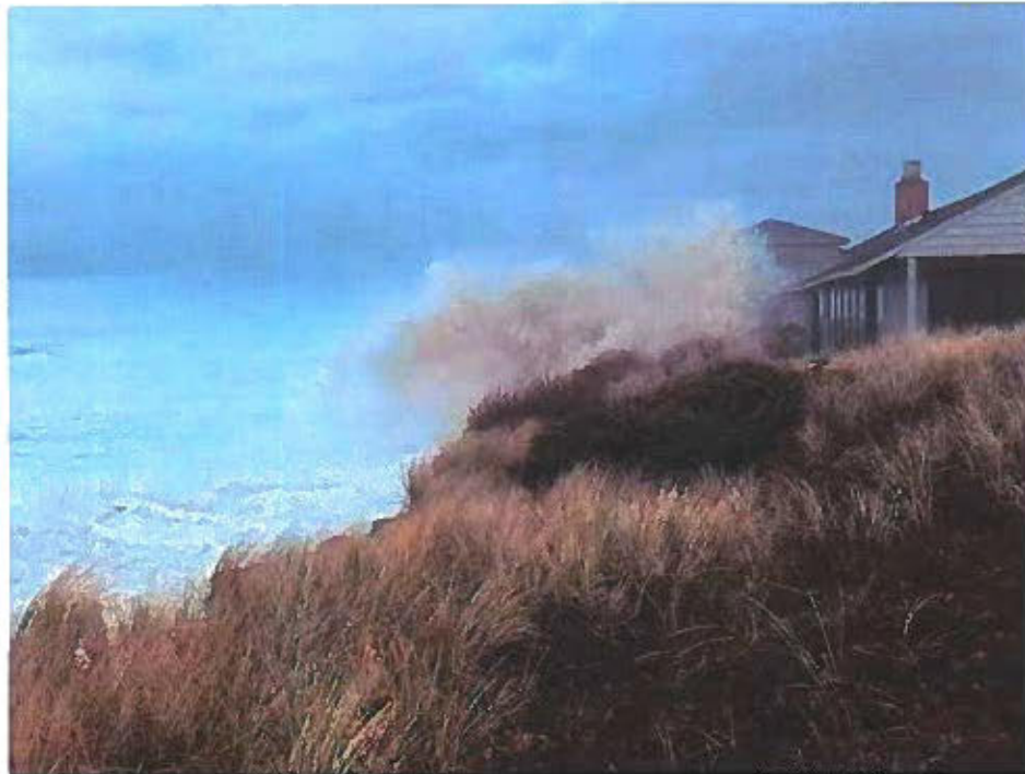
Photo 12 – View of wave splash overtopping the reveitment fronting Tax Lot 701, Map 08-11-03CB, and landing on the roof of the house. Photo extracted from video provided by Jay Sennewald.
