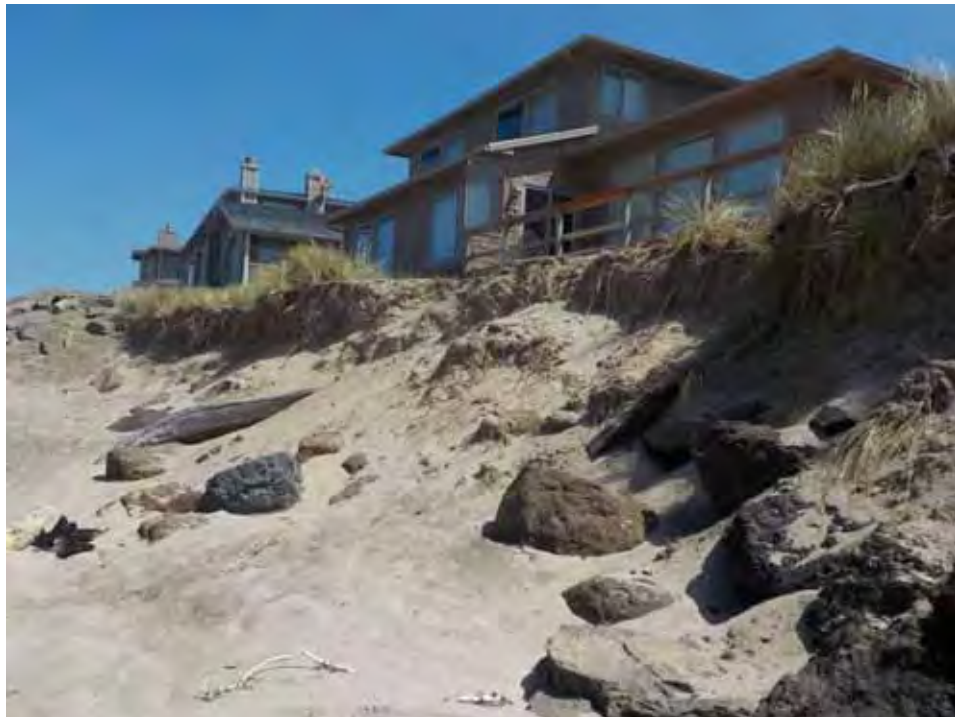
Photo 10 – View of the erosion scarp and damaged revetment fronting Tax Lot 900, Map 08-11-03CB. Note the inadequate size and poor quality of the armor stone of the damaged revetment. (Also see Appendix A-2)
