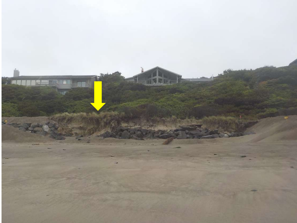
Photo 3 – Easterly view of the site from the beach. Photo taken June 10, 2022. Note that the revetment has been damaged since our 2019 visit (Photo 1), and adjacent revetments had been recently repaired and covered with sand. Approximate location of existing walkway indicated with yellow arrow.
