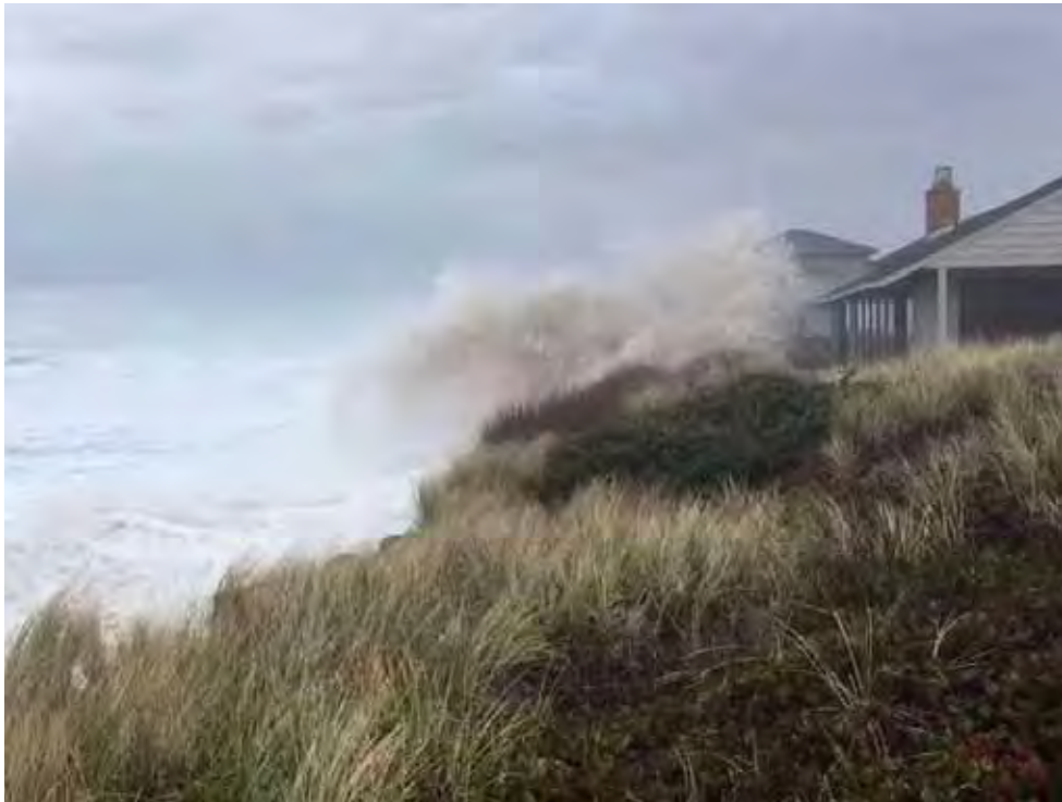
Photo 12 – View of wave splash overtopping the revetment fronting Tax Lot 701, Map 08-11-03CB, and landing on the roof of the house. Photo extracted from video provided by Jay Sennewald.
