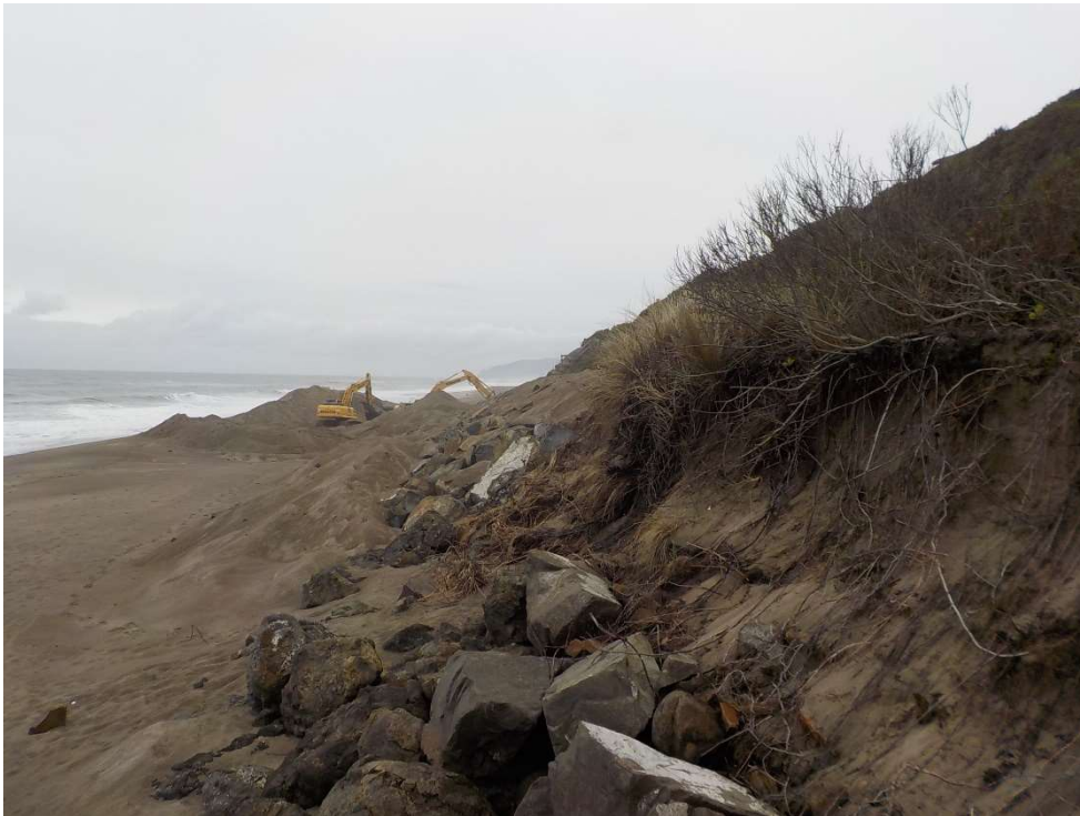
Photo 6 – Northerly view along the top of the existing damaged revetment at the site and the adjacent, recently repaired revetment. Photo taken May 27, 2022.
