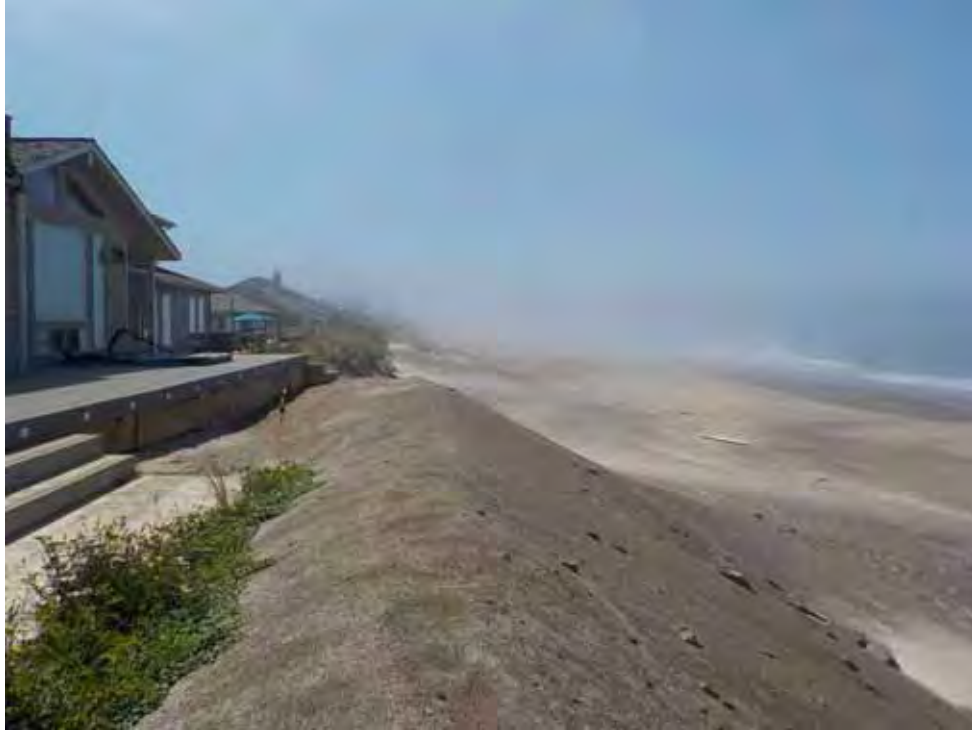
Photo 9 – Southerly view along the top of a recently built revetment fronting Tax Lot 1000, Map 08-11-03CB. Severe erosion during winter 2018/2019 necessitated emergency construction of this revetment to prevent further damage to the house. (Also see Appendix A-2)
