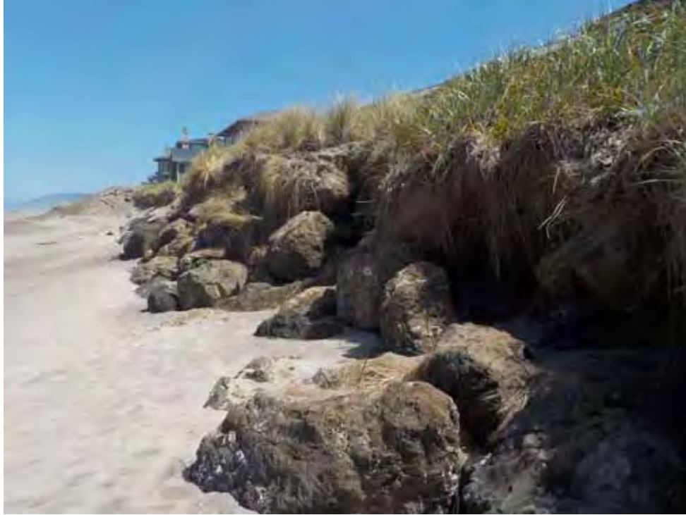
Photo 11 – Close-up view of the inadequate armor stone exposed during the winter of 2018/2019.
