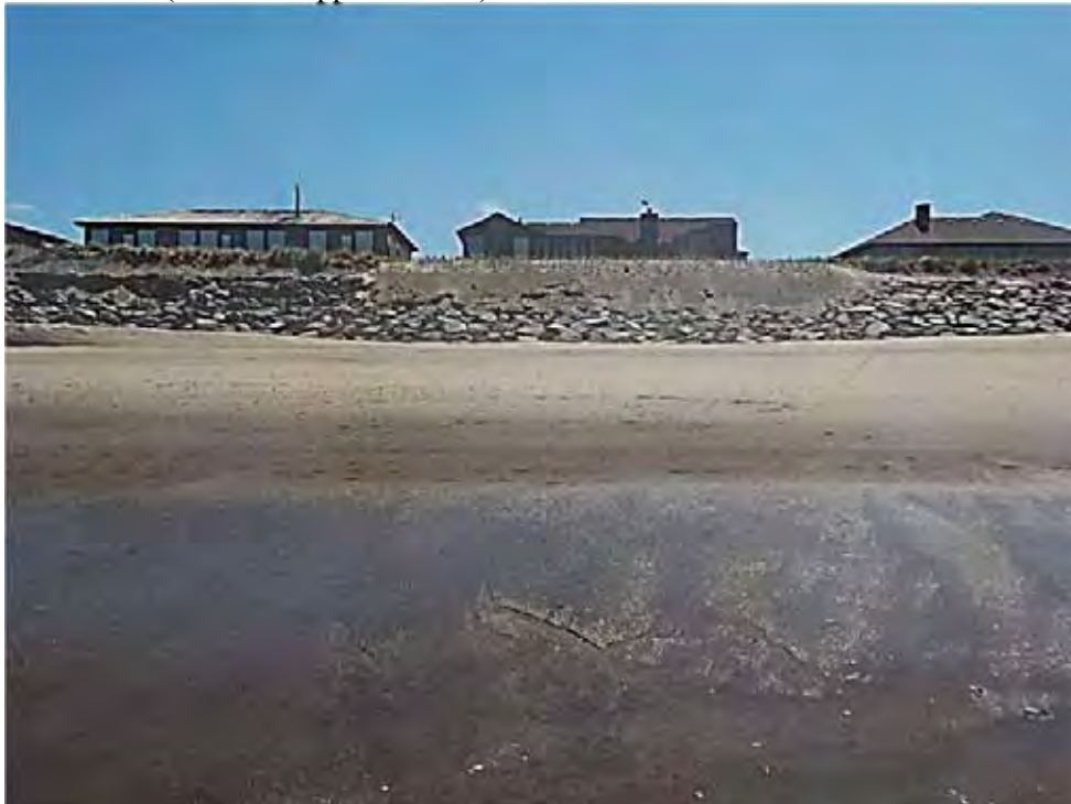
Photo 16 – View to the west of the revetments fronting Tax Lots 217 (right), 218 (center) and 219 (left), Map 08-11-03CC. The height of the revetment fronting Tax Lot 218 was recently raised to help mitigate overtopping (Also see Appendix A-2).
