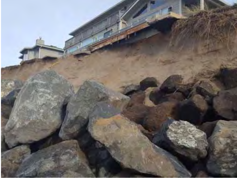
Photo 11 – View of the erosion that damaged the structure at Tax Lot 1000, Map 08-11-03CB, and riprap placed under an emergency permit. Photo taken on January 7, 2019 and submitted to oregonshores.org by user “ORbeach”.
