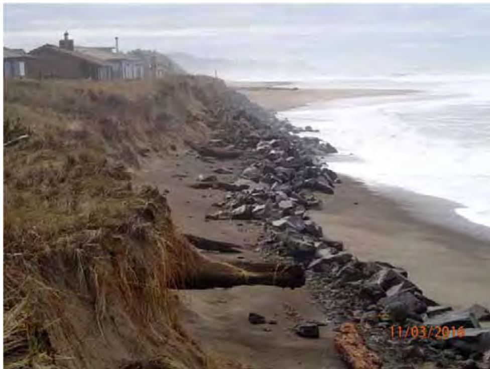
Photo 6 – March 2016 storm damage to riprap at Salishan affected 11 properties. Wave overtopping, inadequate design and poor construction contributed to the problem. From Sennewald (2018)
