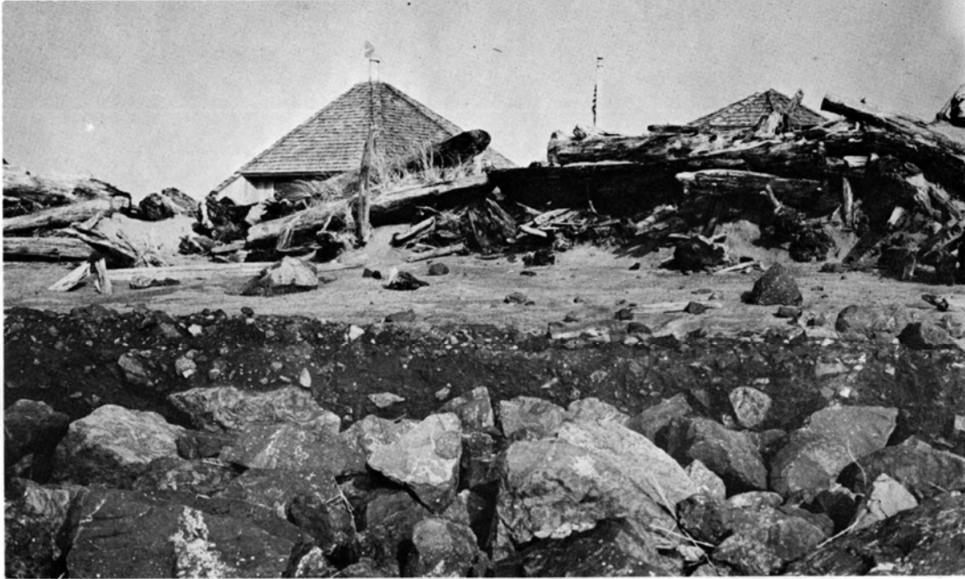
Figure 8. Erosion of the riprap seaward of the northern-most house, photographed on 20 March 1976. It is seen that some of the finer-grained material backing the larger rocks has been eroded away. Waves washed over the riprap pushing back the drift logs into a pile.
