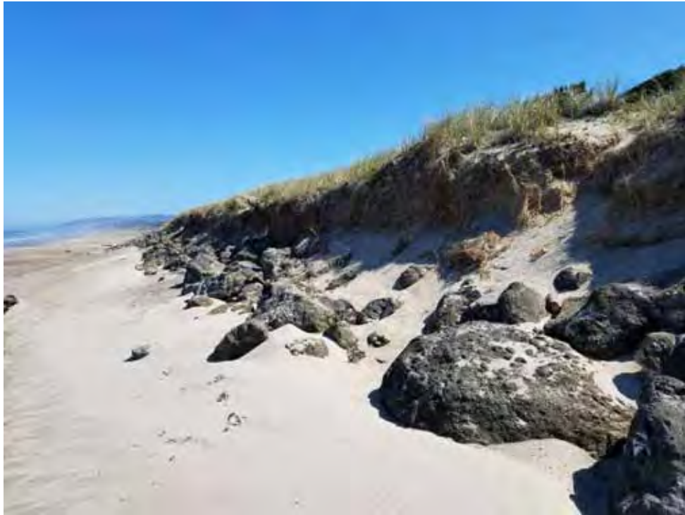
Photo 18 – View of the loosely stacked basalt breccia armor stones used in construction of the original revetments.
