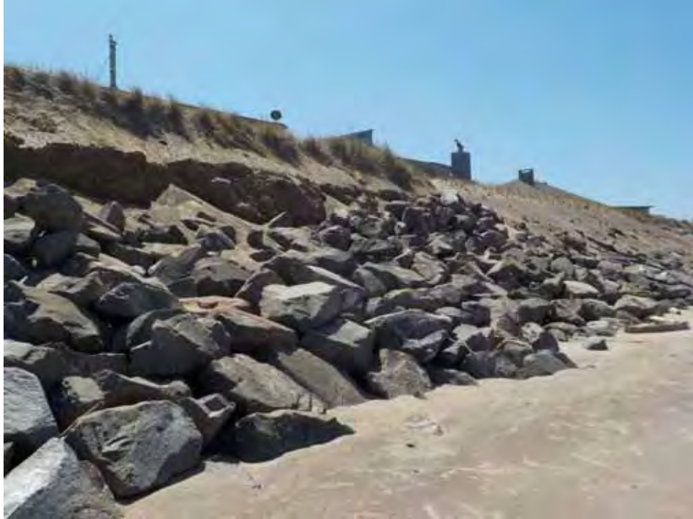
Photo 15 – View of damaged recently constructed revetment fronting Tax Lot 219, 08-11-03CC (Also see Appendix A-2).
