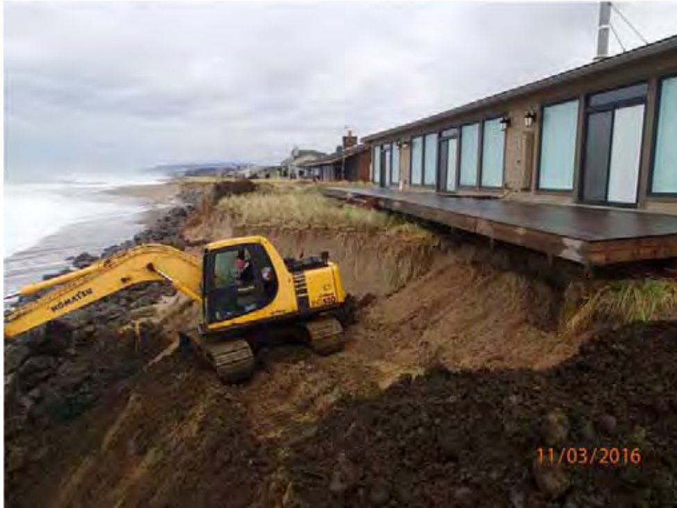
Photo 7 – Photo of emergency repairs underway to protect Tax Lot 219, Map 08-11-03CC. From Sennewald (2018)
