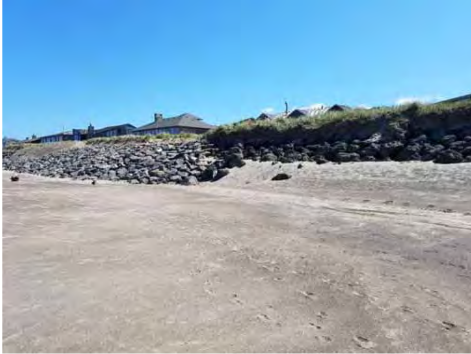
Photo 17 – Southeasterly view of the transition from competent high-quality rock at the southern extent of the recently constructed (2016) revetments to low-quality basalt breccia rock to the south.
