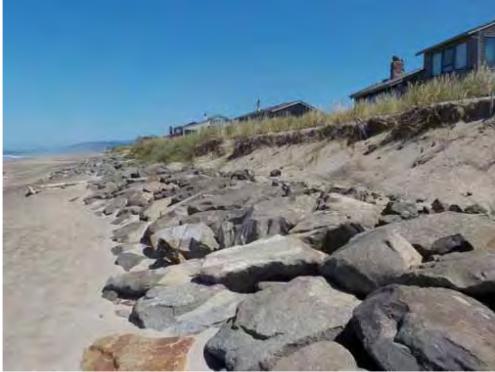
Photo 13 – Close-up view of the top of the revetment fronting Tax Lot 401, Map 08-11-03CB. Note the shallow revetment angle ( \sim 15^\circ ; \sim 3.5H:1V ) and the erosion on the dune east of the revetment caused by overtopping of the revetment.
