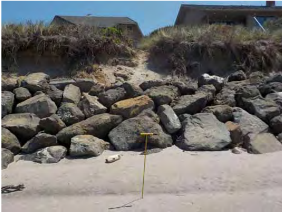
Photo 20 – View of a revetment where competent rock is mixed with poor-quality basaltic breccia.
