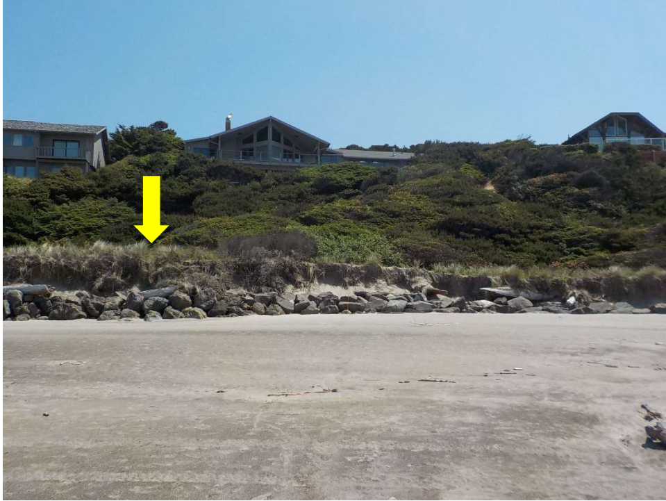
Photo 1 – Easterly view of the site from the beach. Photo taken May 31, 2019. Note the erosion scarp present above the revetment indicating overtopping by waves. Approximate location of existing walkway indicated with yellow arrow.
