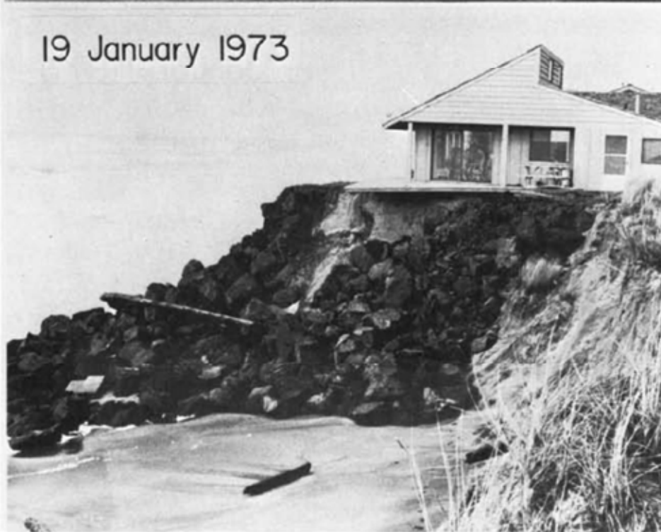
Figure 3. Erosion around the house on lot 229-A. Rapid erosion required placement of riprap fronting home in upper photo; but no riprap was installed in adjacent vacant lot, so erosion continued along the side as seen in lower photo.
