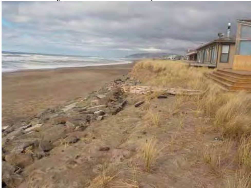
Photo 10 – Northerly view of the top of the revetment at Tax Lot 218, Map 08-11-03CC after the 2018/2019 winter when the revetment was overtopped. Note the erosion of the topping sand, the drift log on the top of the dune, and the plywood used to protect the windows. Photo taken by HGSA on 03/01/2019.
