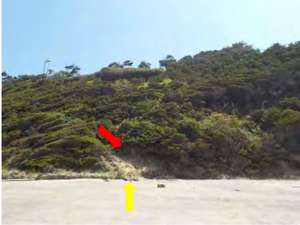
Photo 23 – Westerly view of the southern termination of the revetment (indicated with yellow arrow) along the northern property boundary of Tax Lot 156, Map 08-11-09DD. Note the erosion at the toe of the bluff immediately south of the termination of the revetment (indicated with red arrow). (Photo taken 05/31/2019)
