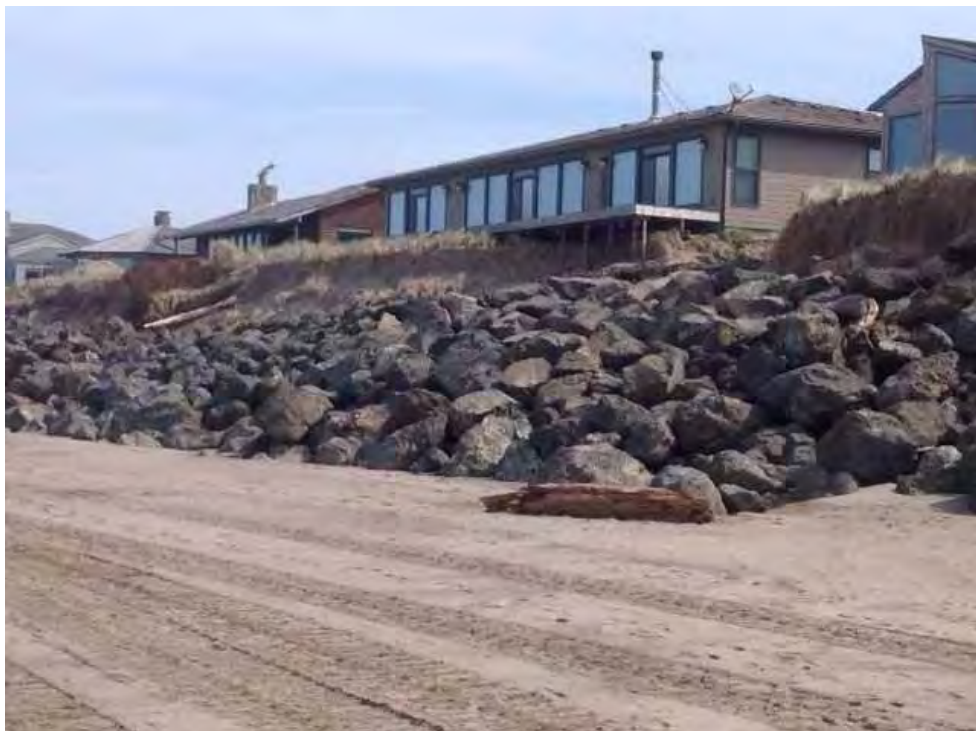
Photo 8 – Photograph taken 16 March, 2016, of emergency repairs completed at Tax Lot 219, Map 08-11-03CC. Provided to HGSA by a Salishan Leaseholder.
