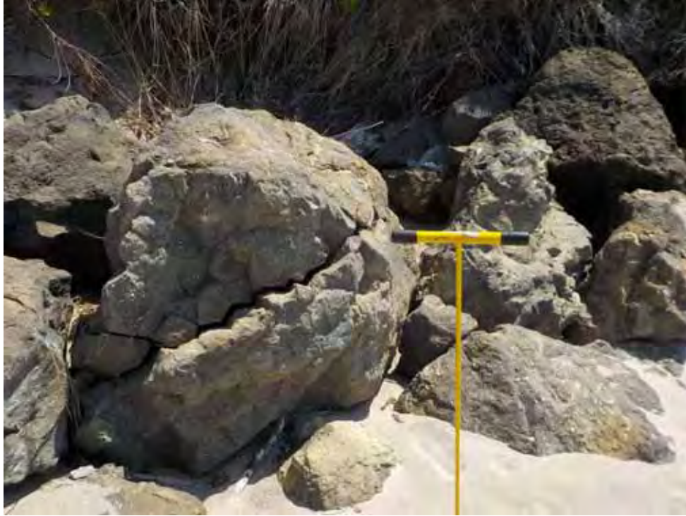
Photo 21 – Close-up view of poor-quality basaltic breccia and pillow basalt armor stones. Note the fractures in the stones.
