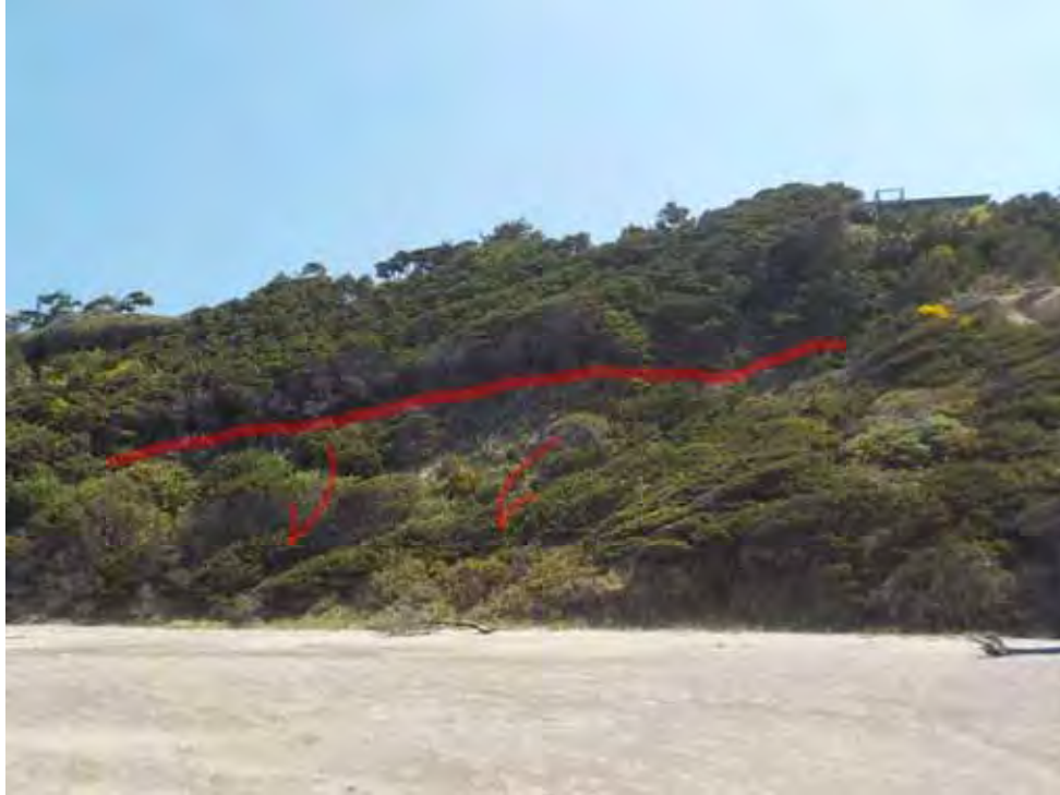
Photo 24 – View of the bluff slope on the western portion of Tax Lot 156, Map 08-11-09DD that has experienced shallow failures due to erosion of the toe of the bluff. Shallow landslide scarp indicated with red line; direction of movement indicated with red arrows.
