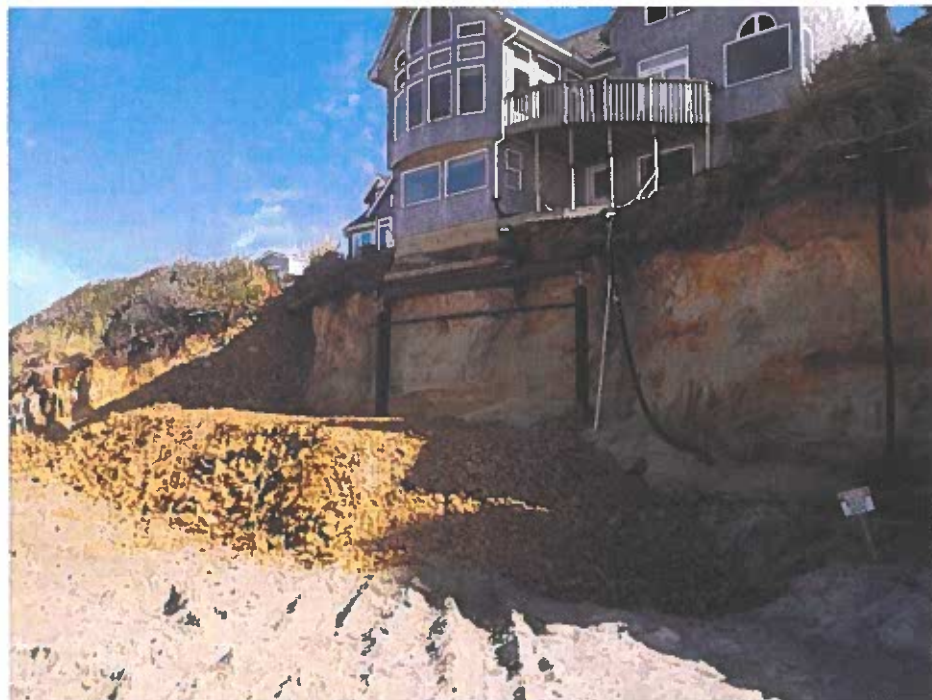
Photo 8 – Northeasterly view of Tax Lots 15000, 15100 and the public walkway/utility easement during placement of quarry-run rock to provide emergency protection. Photograph taken August 17, 2021.
