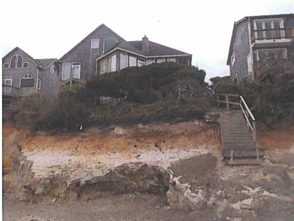
Photo 2 – Easterly view of the bluff slope fronting Tax Lot 14900. Note the erosion is undermining the concrete access stairs and the erosion scarp at the toe of the slope. Photograph taken August 17, 2021.
