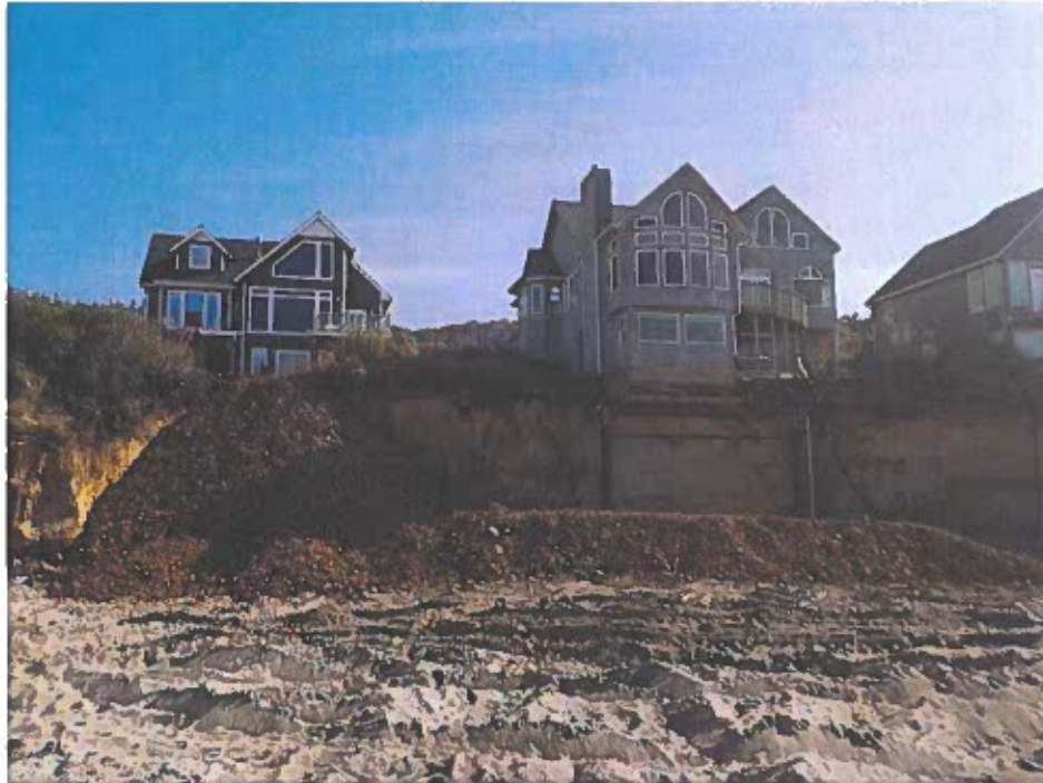
Photo 7 – Easterly view of Tax Lots 15000, 15100 and the public walkway/utility easement during placement of quarry-run rock to provide emergency protection. Photograph taken August 17, 2021.
