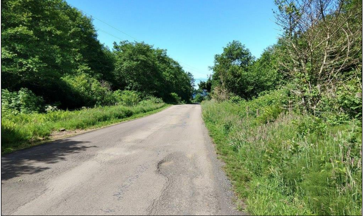
Figure 5. View generally west of location of Vault 5 to be installed on north side of Winema Road (frame right) in center foreground.
