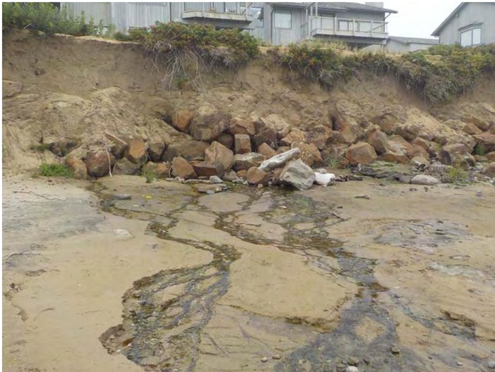
Photo 4 – View of a portion of the curtain drain exposed after severe erosion of the fronting dune and bluff slope (From 08/15/2018).
