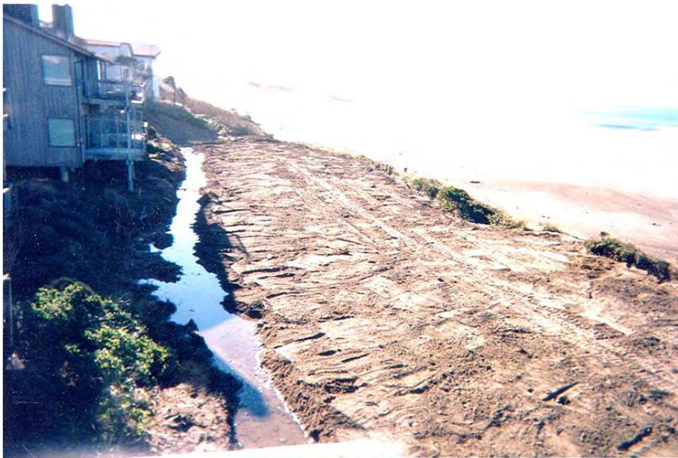
Photo 23 - View of the curtain drain construction (From December 1999 by SeaRidge).
