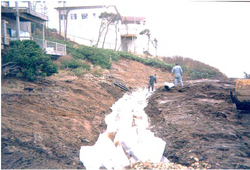
Photo 22 – View of the curtain drain construction (From December 1999 by SeaRidge).
