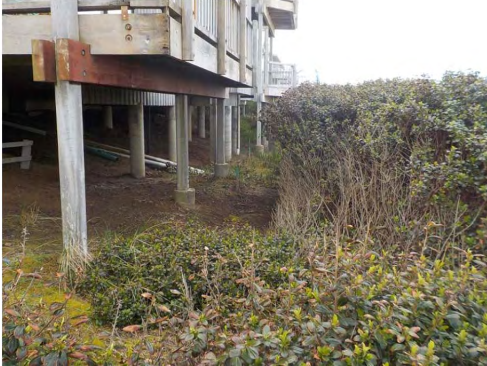
Photo 9 – View of the foundation and deck supports typical of the oceanfront buildings at the site (From 04/25/2022).
