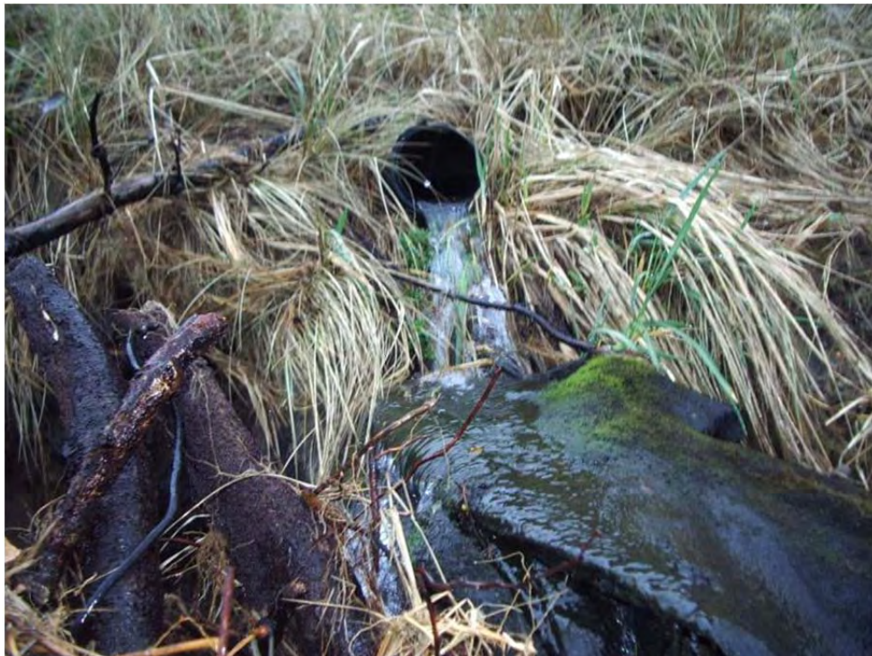
Photo 10 – Close-up view of a stormwater pipe daylighted at the bluff slope (From 02/15/2017).
