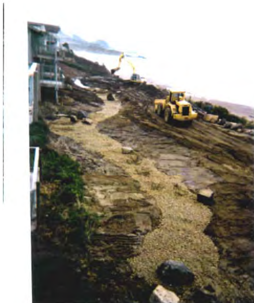
Photo 21 – Composite of 3 photographs showing the construction of the curtain drain (From 2/8/2000 by SeaRidge).
