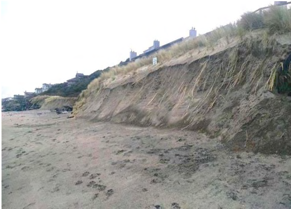
Photo 18 – View of the oversteepened bluff slope after a severe erosion episode (From March 2016 by SeaRidge)
