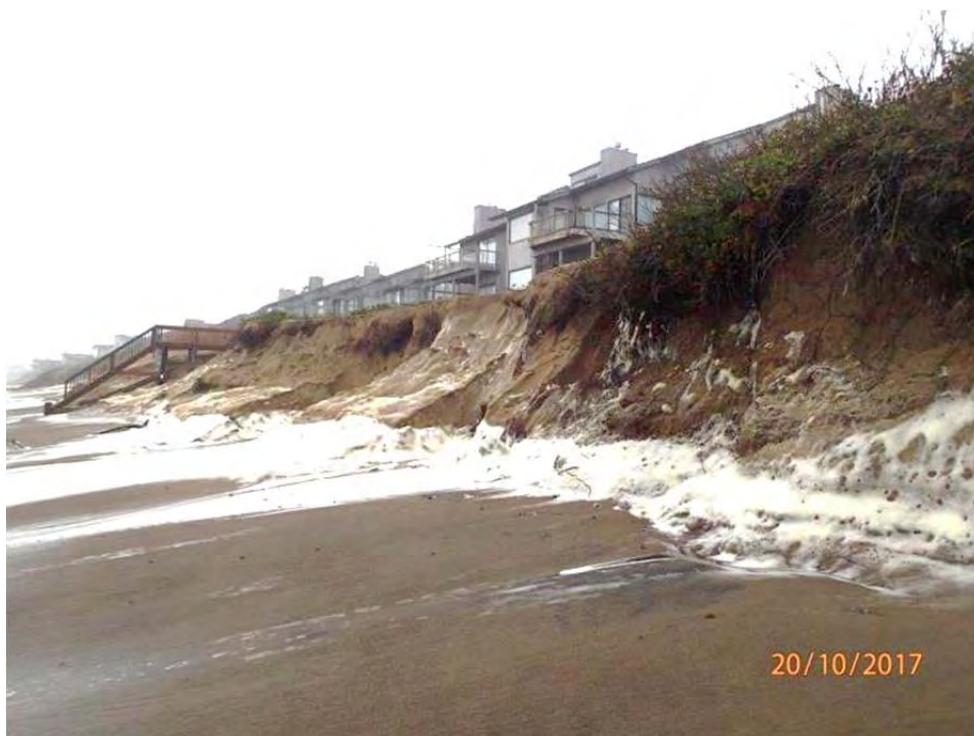
Photo 12 – Northerly view of the central portion of the site as waves impact the bluff and erode the base of the bluff slope (From 10/20/2017 by Sennewald/OPRD)
