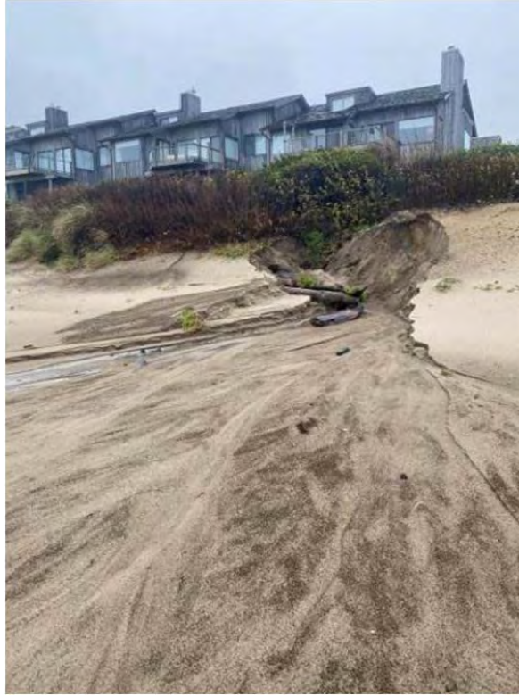
Photo 19 – View of a washout of the bluff slope from stormwater (From 11/15/2021 by B. Dummer)
