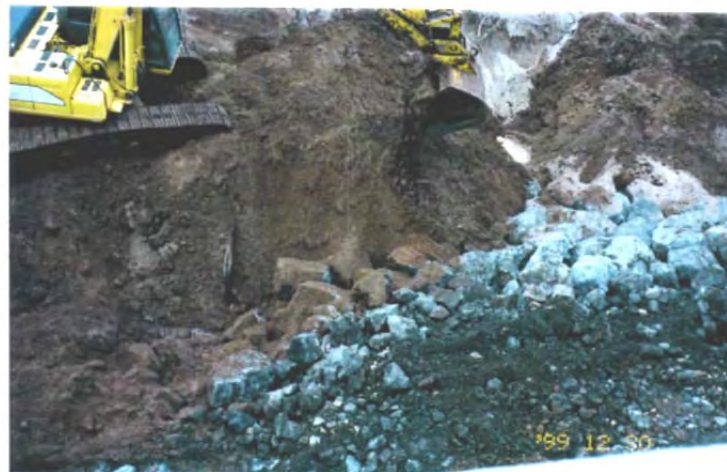
Photo 24 – Composite of 3 photographs showing the construction of the curtain drain (From 12/30/1999 by SeaRidge).
