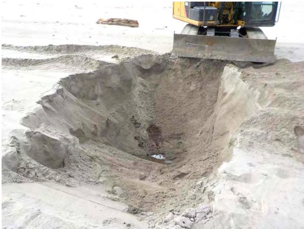
Photo 14 – View of a test pit being excavated; note the water in the bottom of the pit (From 02/24/2022).
