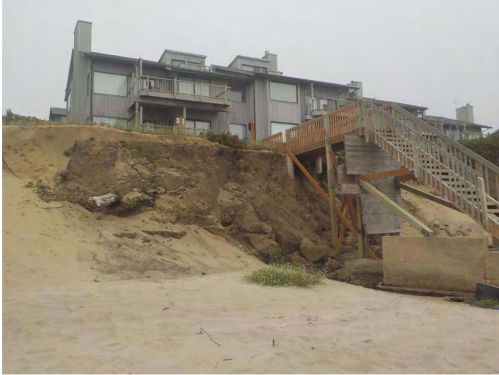
Photo 3 – View of the oversteepened and sloughing bluff slope (From 08/15/2018)
