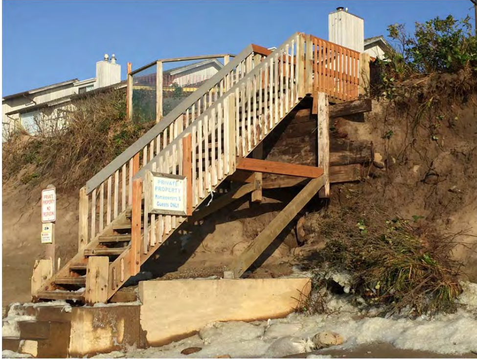
Photo 15 – View of the beach access staircase and oversteepened bluff after a severe erosion episode (From October 2016 by SeaRidge).
