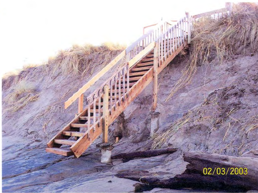
Photo 19 – View of the beach access staircase after being undermined during a severe erosion episode (From 02/03/2003 by SeaRidge)
