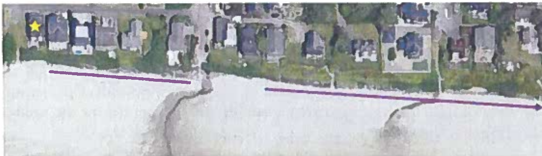
Riprap South of the Property 92
