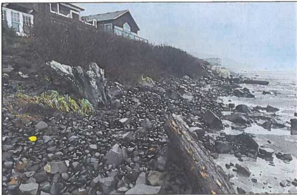
Photo 8: Site conditions at 3276 Pacific Avenue on November 21, 2024, showing the angular rock and cobble along the property's shoreline acting as a dynamic revetment for the property.
