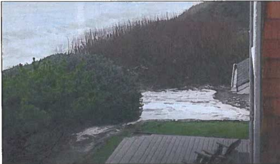
Photo 1: Snapshot captured from a video showing water pooling on the subject property during an event with repetitive waves breaking over the bluff. The deck of the subject residence can be seen in the foreground.
