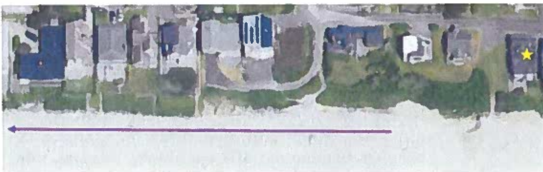
Riprap North of the Property 93
