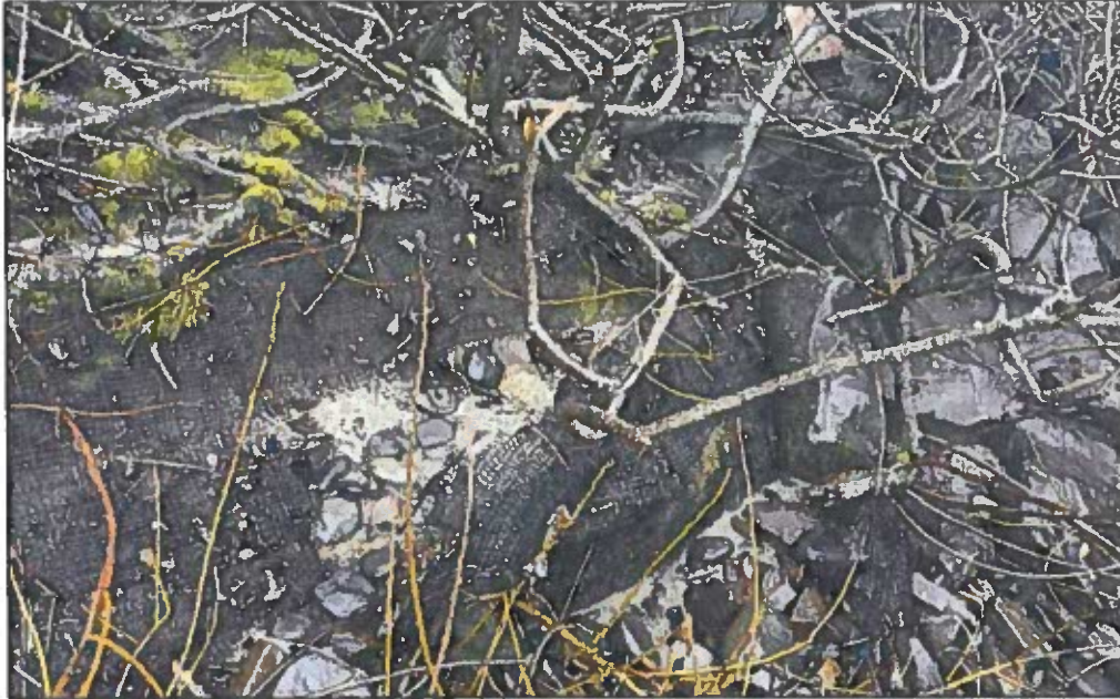
Photo 9: Site conditions at 3276 Pacific Avenue on November 21, 2024, showing the failing sand burrito, as well as the angular rock and cobble along the property's shoreline.
