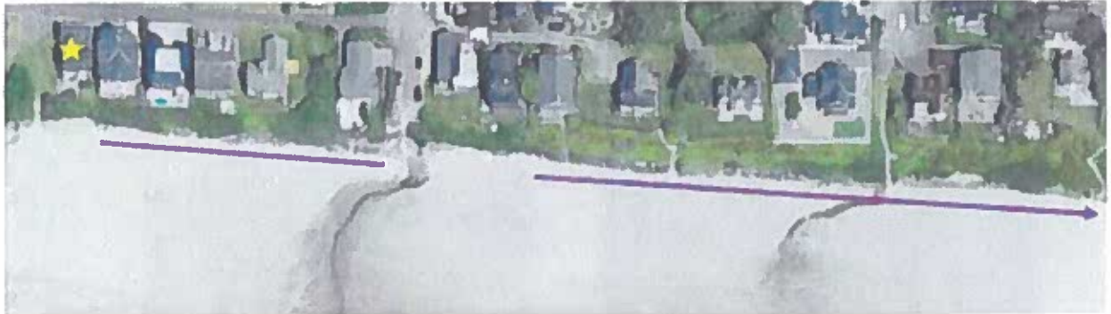
Riprap South of the Property 19
