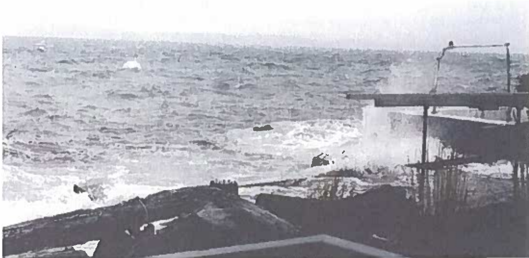
Figure 6. Inundation of lawn and house foundation by waves (West Seattle, 2006)
