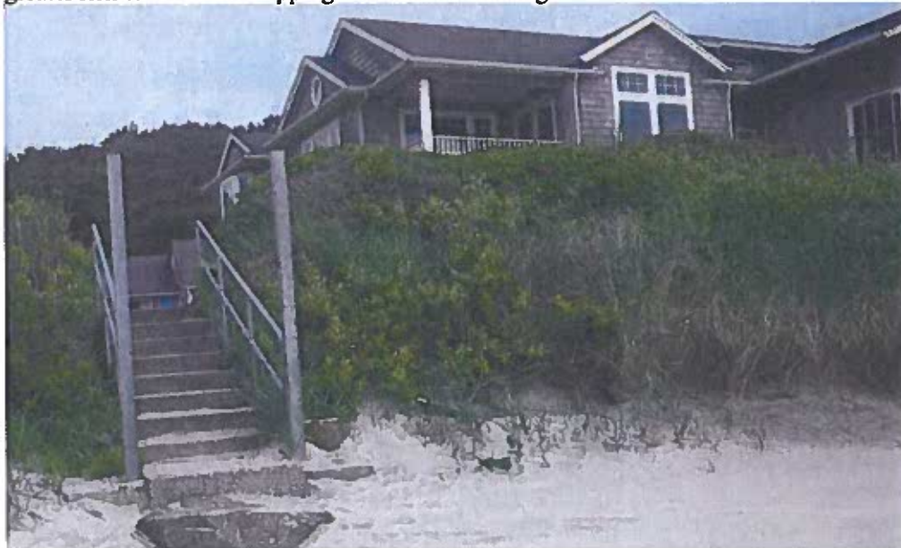
Figure 8. Eroding bluff that fronts the Siegel residence, May 10, 2025
