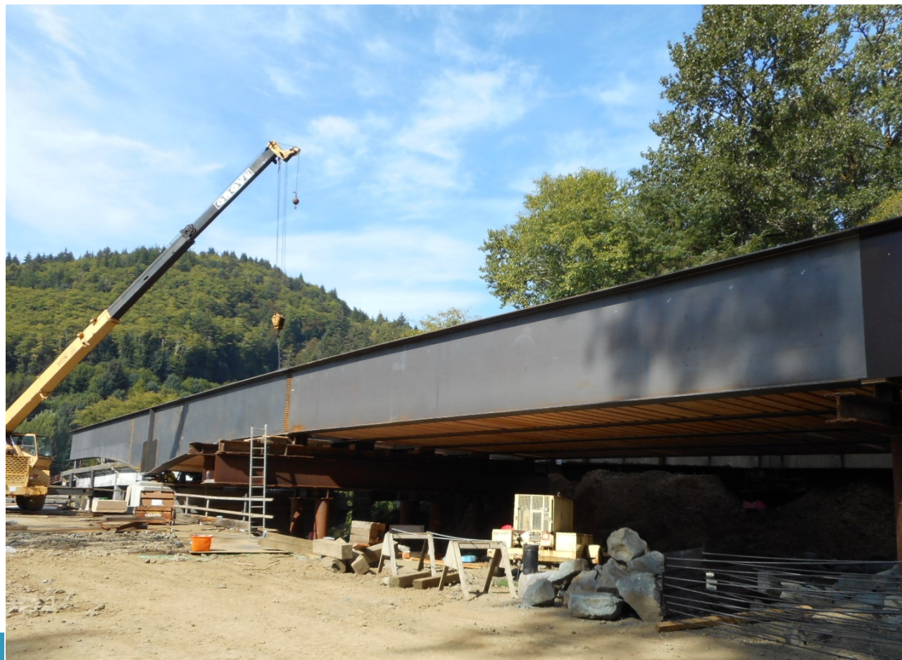
Beam Installation
