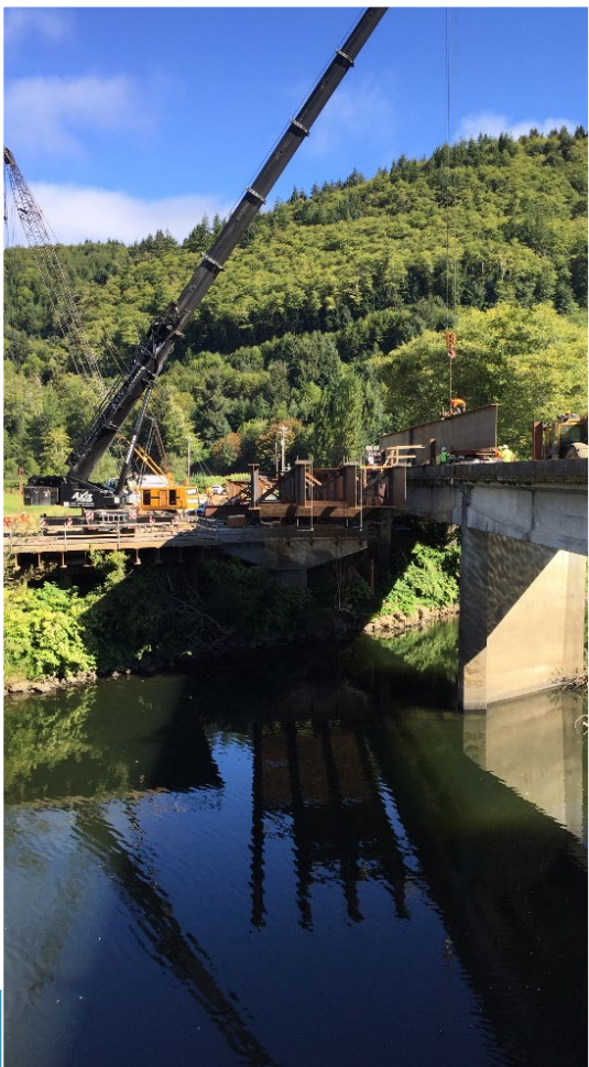
Beam Installation
