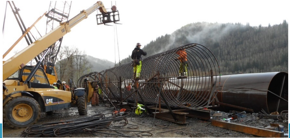
Drill Shaft Installation
