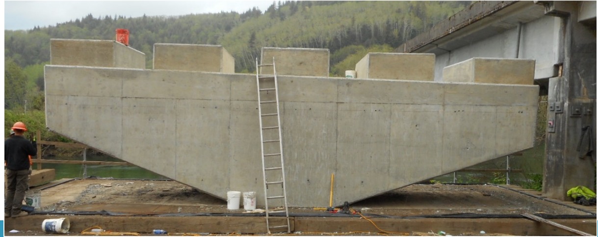
Bent Cap Installation
