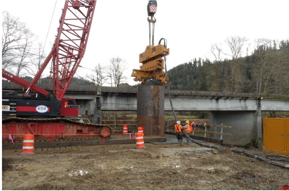
Drill Shaft Installation
