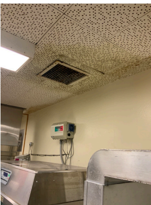
D30 HVAC Systems – Deferred Maintenance
