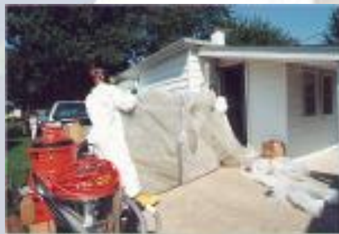
View of mercury-contaminated carpet removal.
