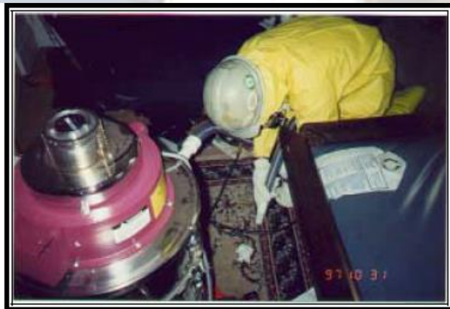
View of U.S. EPA ERRS contractor using a mercury vacuum to collect liquid mercury from the floor of a bedroom.
