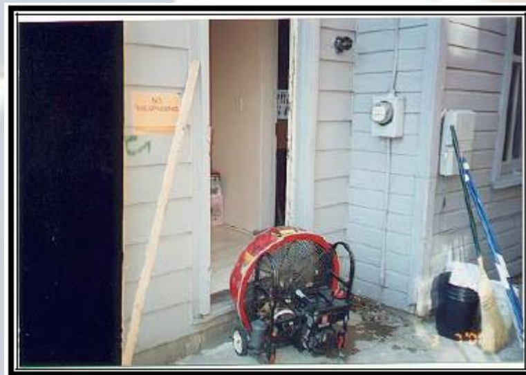
View of industrial fans blowing air into the house to allow venting of volatilized mercury.
