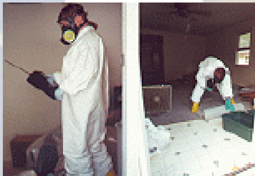
View of Jacome mercury vapor air sampling and mercury-contaminated carpet removal.
