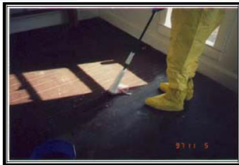
View of U.S. EPA ERRS contractor mopping floors with HgX solution.
