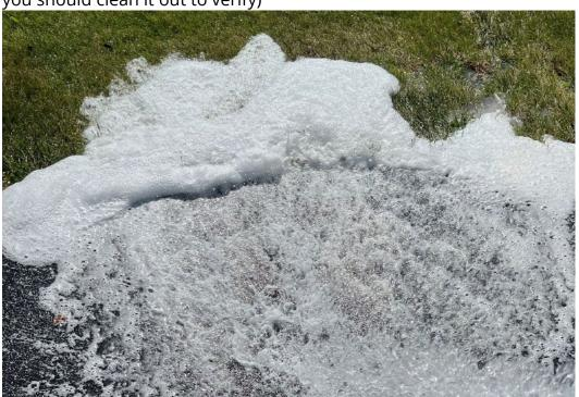
Keep flushing the system until the discharged water is clear and no bubbles as shown below.
