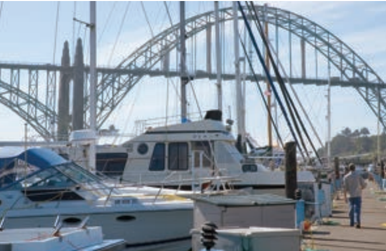
The Yaquina Bay Bridge looms over South Beach
