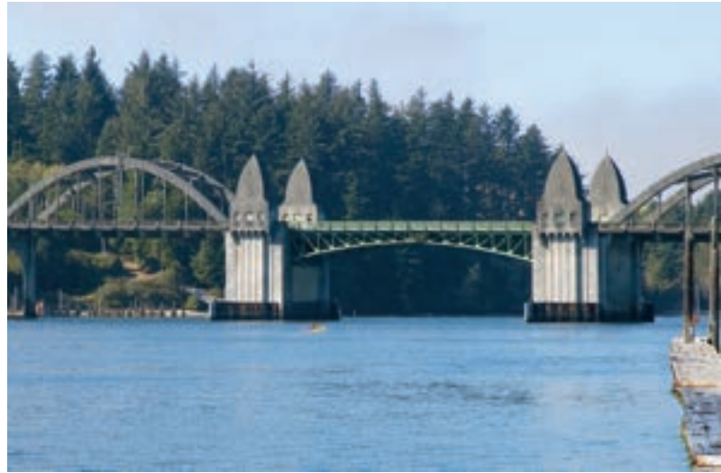
Historic Siuslaw River bridge
