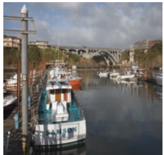
Depoe Bay bridge from the harbor side
