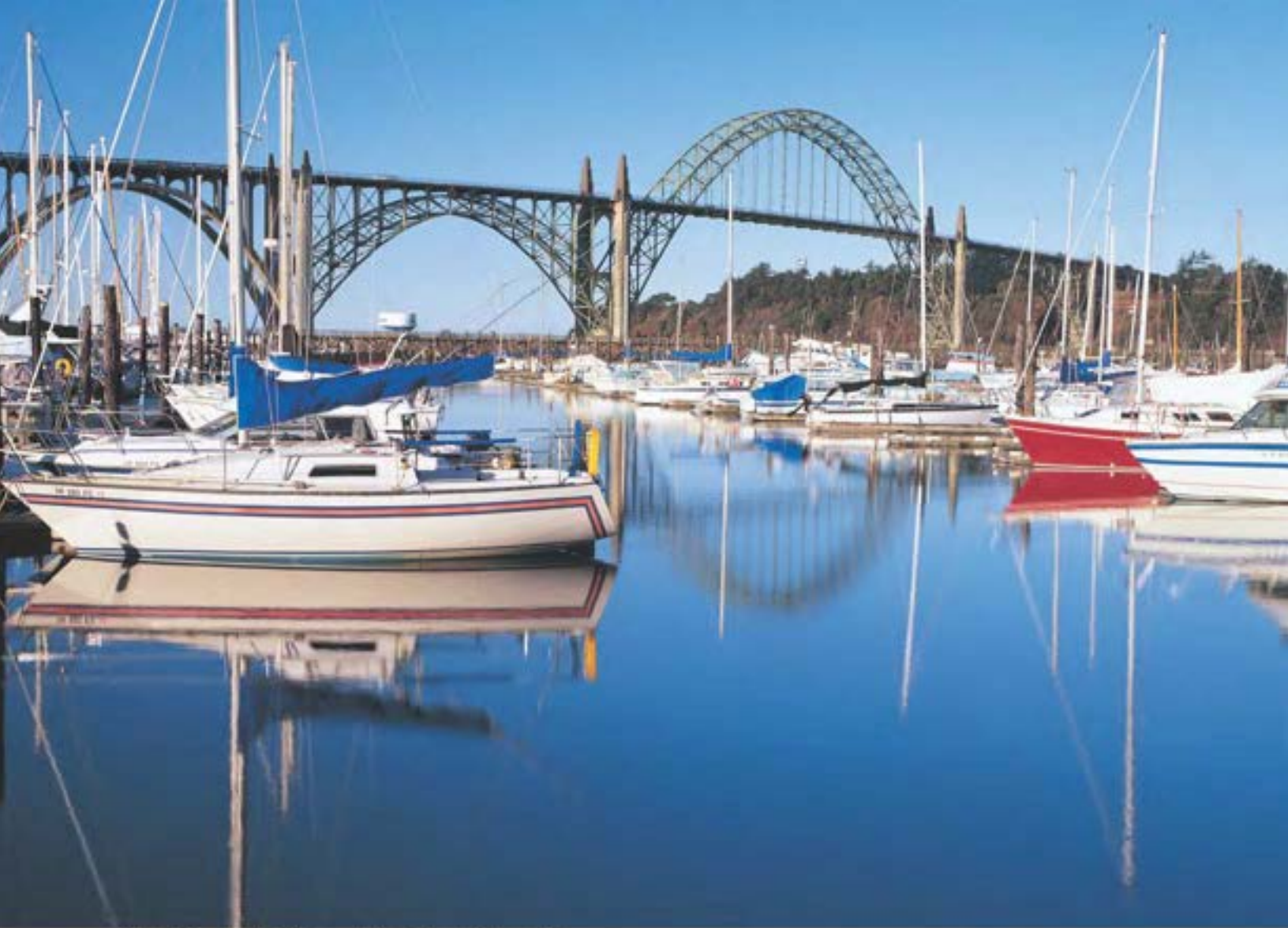
Historic Yaquina Bay Bridge and South Beach Marina at Newport.
