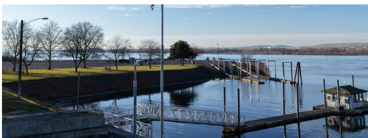
Fuel dock with boat ramp in the background
