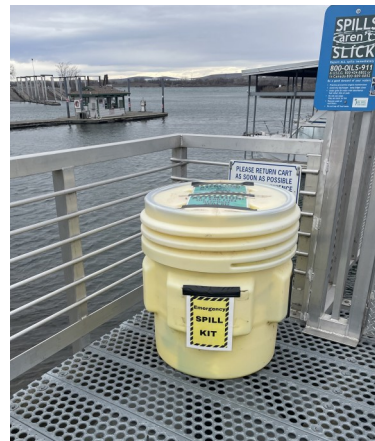
Emergency oil spill kits at the top of each gangway
