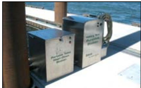
Photo 5-2 Float mounted pumpout and dump station
