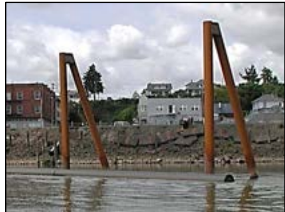
Photo 6-2 Batter supported vertical piles
