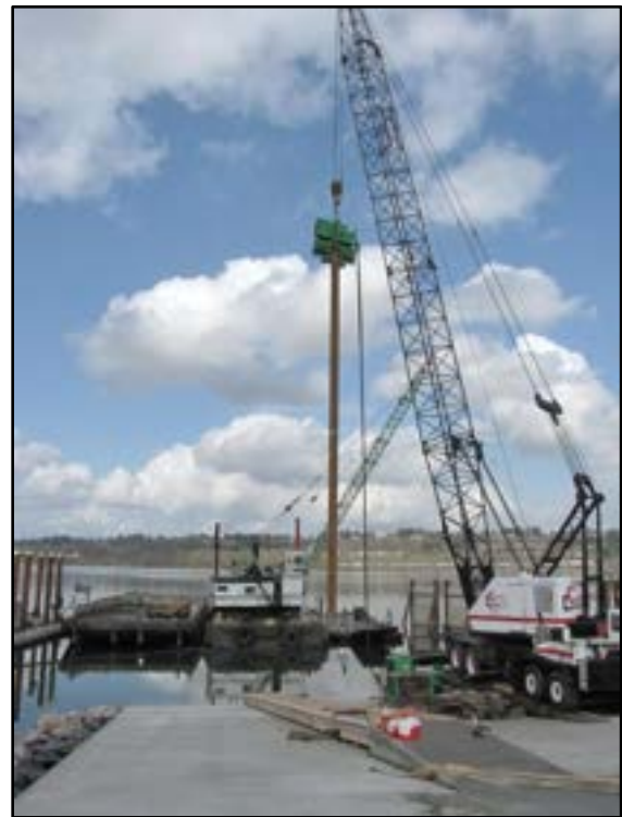
Photo 6-4 Land-based pile driving crane with vibratory hammer
