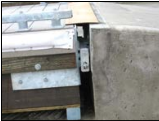
Photo 4-13 Hinged abutment connection
