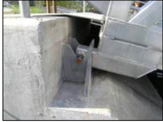
Photo 7-7 Lift-off connection at abutment end of gangway
