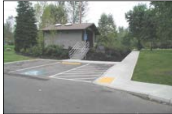
Photo 10-3 Restroom built on fill to be above the 100-yr flood elevation. The sidewalk provides ADA accessibility while the stairs provide a more direct route.
