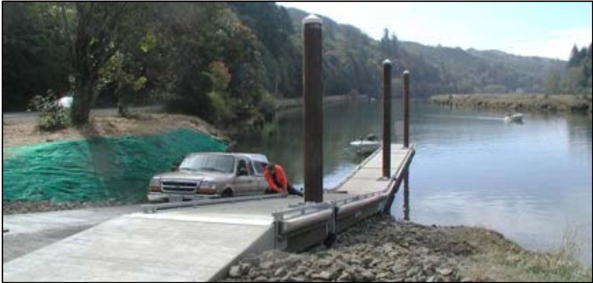
Photo 4-2 Preferred boarding float location for a single-lane launch ramp. Floats are placed on the right-hand and upstream side of launch ramp with internal pile pockets opposite the launch lane. Also note angle of launch ramp in the downstream direction.
