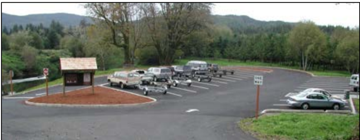
Photo 9-11 Typical one-way grid system parking area with angled stalls
