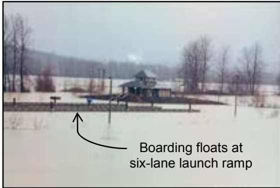
Photo 10-2 This photo was taken during a 100-yr flood event. The restroom was built well above the flood elevation.
