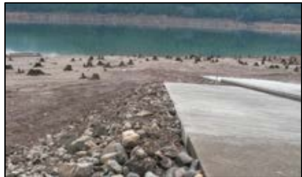
Photo 3-2 Two-lane ramp with short lane on left and long lane on right
