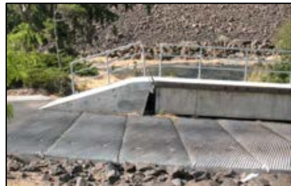
Photo 4-9 Example of floats that are too tall when grounded on the launch ramp. The slope of the abutment is also excessive.
