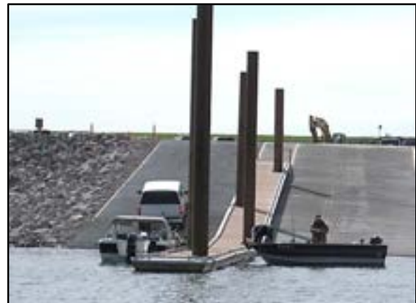
Photo 4-3 Boarding floats between launch lanes
