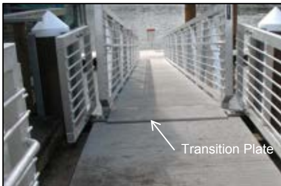
Photo 7-4 Transition plate at shore-end of gangway
