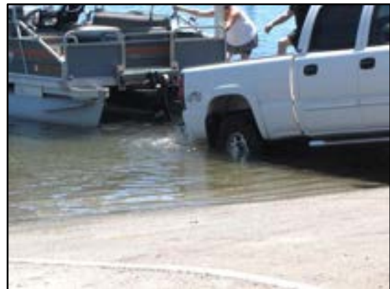
Photo 3-6 Insufficient ramp slope places tow vehicle in the water and does not provide access to the trailer without getting wet
