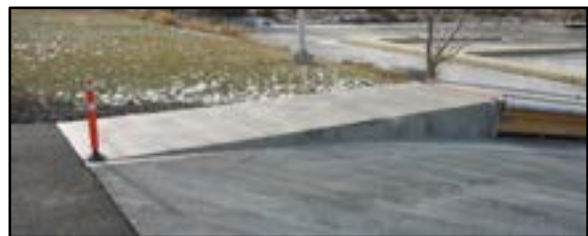
Photo 4-4 Concrete float abutment
