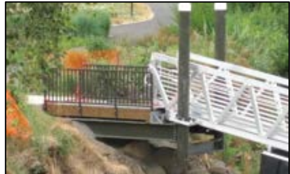
Photo 7-10 Cantilevered steel and timber fixed-pier connection
