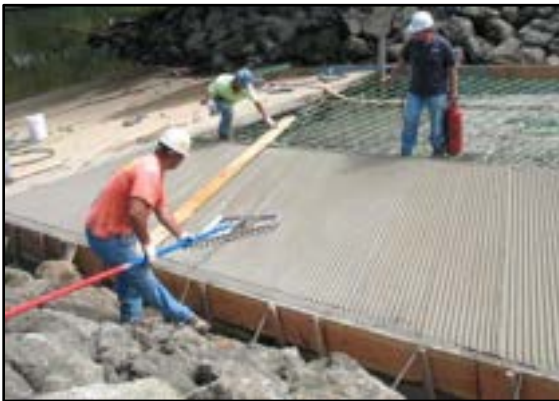
Photo 3-33 Subsequent passes with the groove tool cleans up the grooves and adds definition
