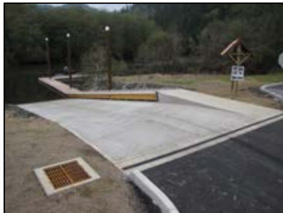
Section 3 – Launch Ramps
