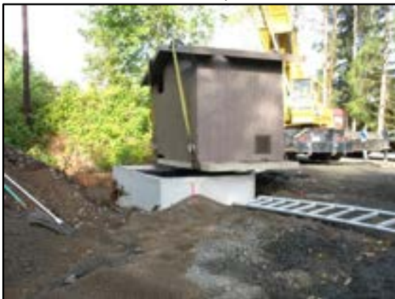
Photo 10-8 Installation of precast vault toilet
