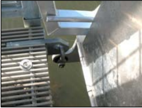
Photo 7-6 Link connection at pier-end of gangway
