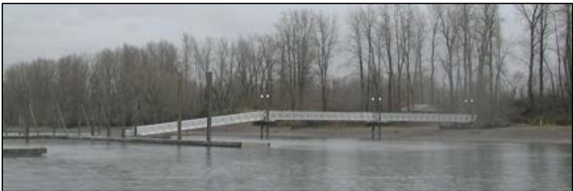
Photo 7-2 A series of gangways is required at this facility to access the transient floats. The two shoreward gangways are considered elevated walkways.
