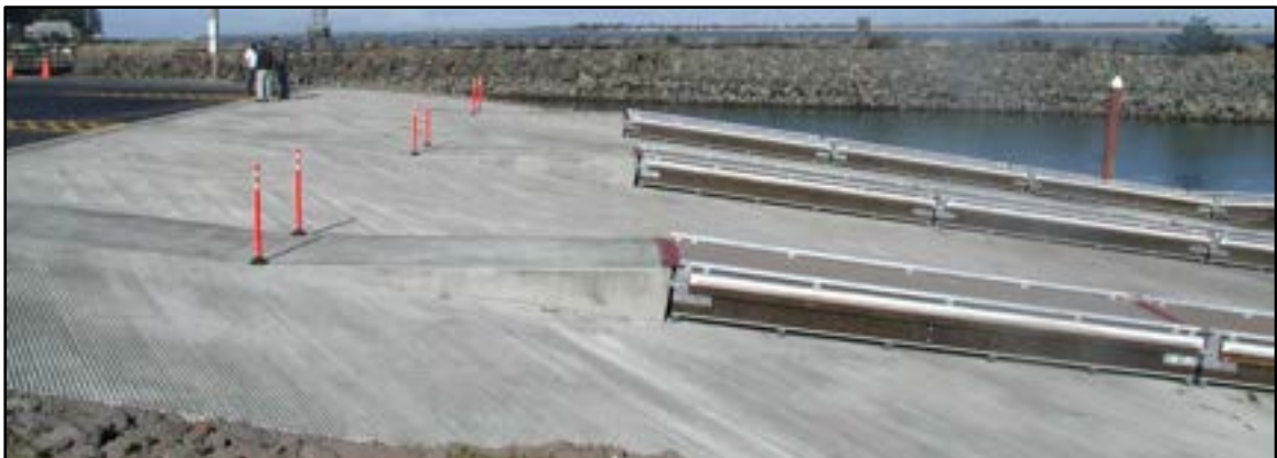
Photo 3-16 Six-lane launch ramp with boarding float access for each lane
