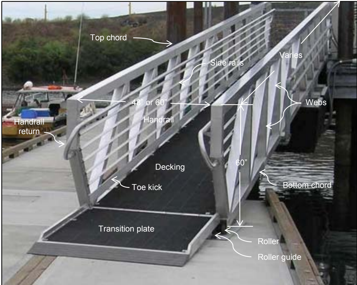
Photo 7-8 Gangway design components
