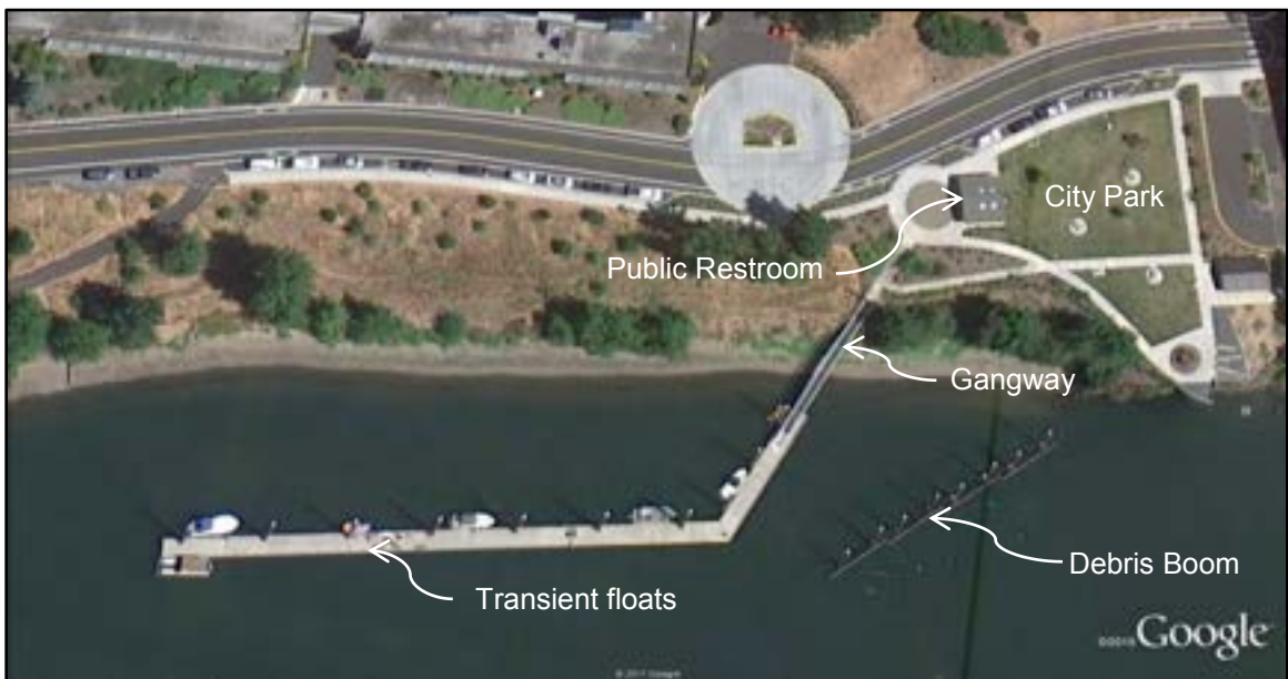
Photo 5-1 Transient facility showing gangway connection to upland amenities
