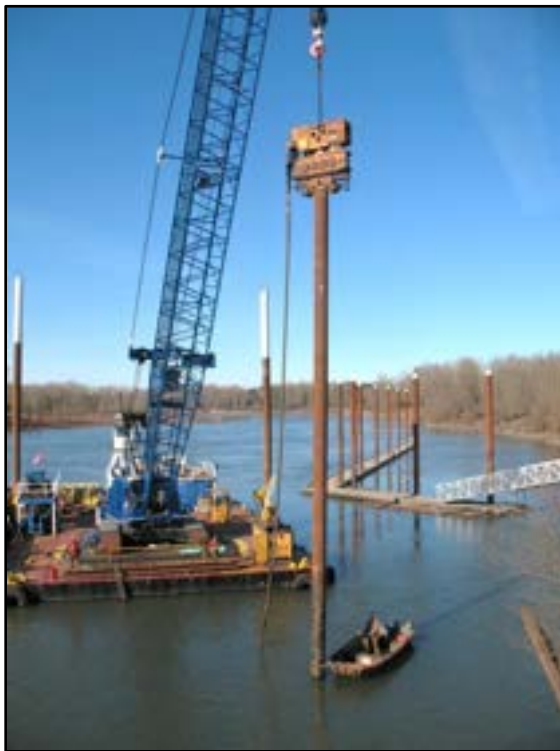
Photo 6-3 Barge mounted pile driving crane with vibratory hammer
