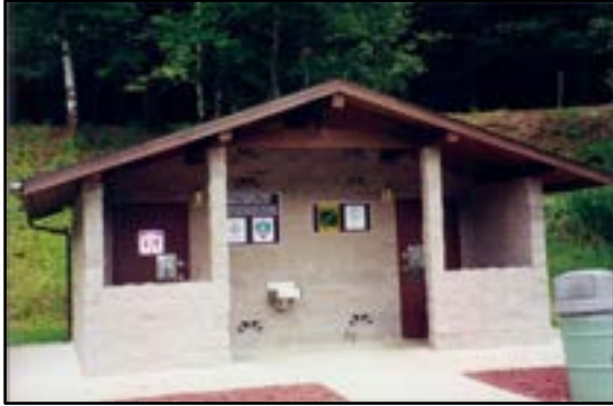
Photo 10-6 Site-built flush restroom
