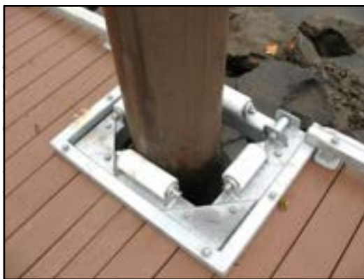
Photo 4-11 Internal pile pocket
