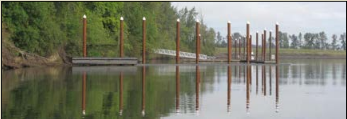
Photo 8-7 Poly-pipe debris boom protecting a transient facility
