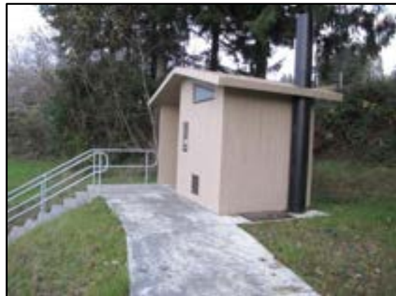
Photo 10-9 Precast concrete vault toilet
