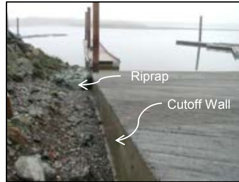
Photo 3-19 Cutoff wall along edge of ramp and riprap backfill
