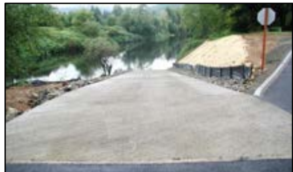
Photo 3-3 Launch ramp angled approximately 45 degrees in the downstream direction
