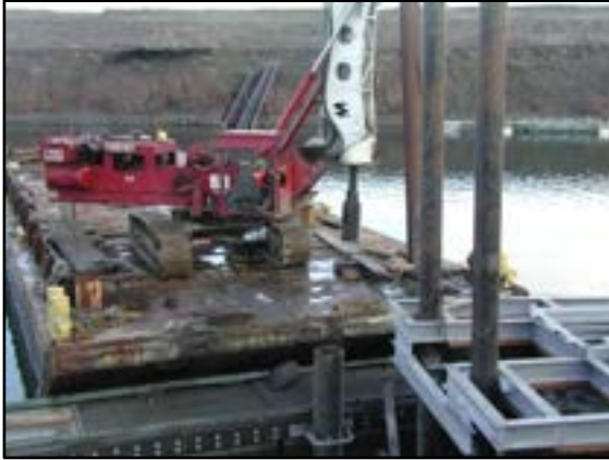
Photo 6-7 Drill rig preparing for drilling
