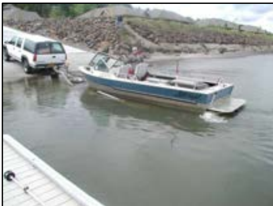
Photo 3-5 Proper ramp slope keeps tow vehicle out of the water and provides access to the trailer
