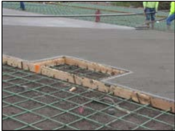
Photo 3-21 Longitudinal cold joint at edge of launch lane and form boards notched for rebar. Rebar will be blocked prior to placement of concrete.
