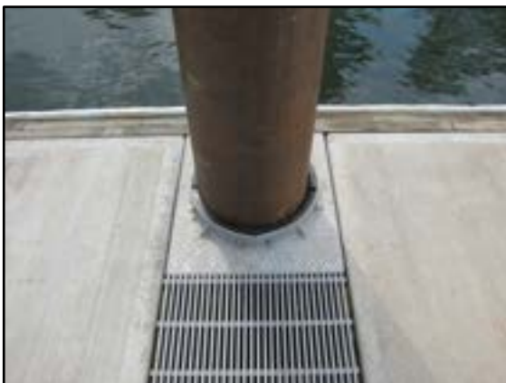
Photo 5-13 Internal pile pocket
