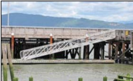
Photo 7-9 Timber fixed-pier connection
