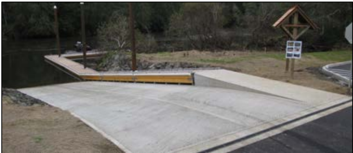
Photo 3-10 Single-lane launch ramp with boarding floats. Lane width is 20 feet with cold joint centered on launch lane.
