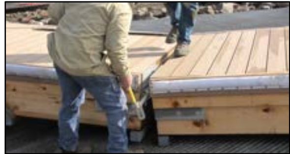
Photo 4-15 Connecting boarding float sections
