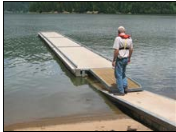
Photo 4-8 Self-adjusting boarding floats
