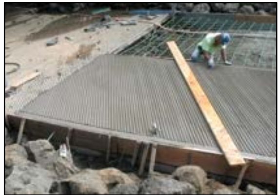
Photo 3-34 Final refinement is done with hand tools including a flat 4" border at edges. Note groove angle matches precast planks.
