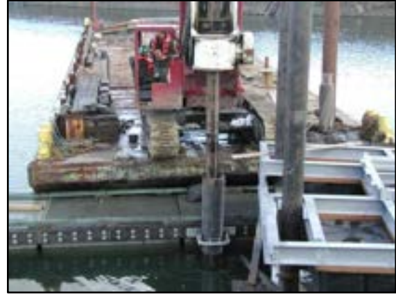
Photo 6-8 Drill rig in position and drilling
