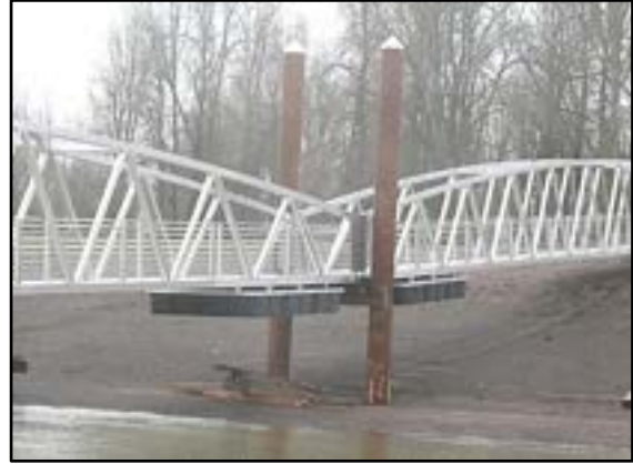
Photo 7-14 Pile supported connection for two gangways
