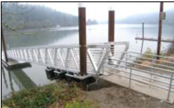
Photo 7-11 Concrete abutment connection
