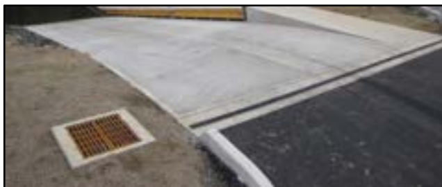
Photo 3-37 Trench drain installed along top of launch ramp
