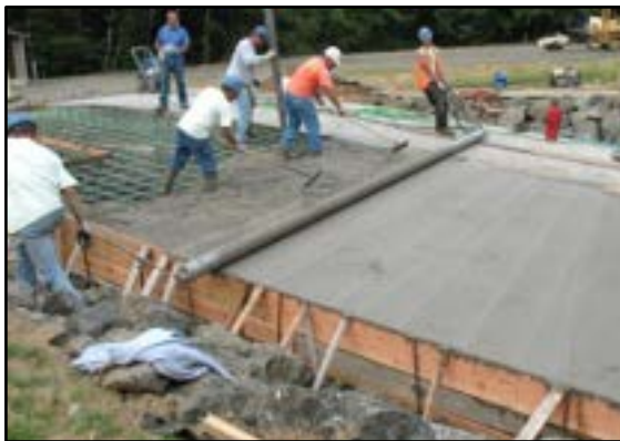
Photo 3-31 Placing fresh concrete into forms and using a power screed to level concrete with tops of forms
