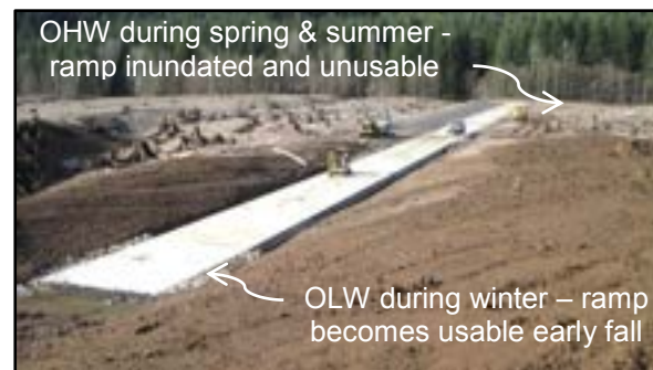
Photo 3-7 Low water launch ramp at a reservoir
