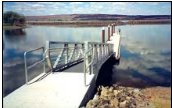
Photo 7-1 Typical gangway application
