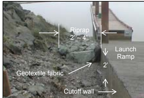
Photo 3-36 Riprap being placed along edge of launch ramp
