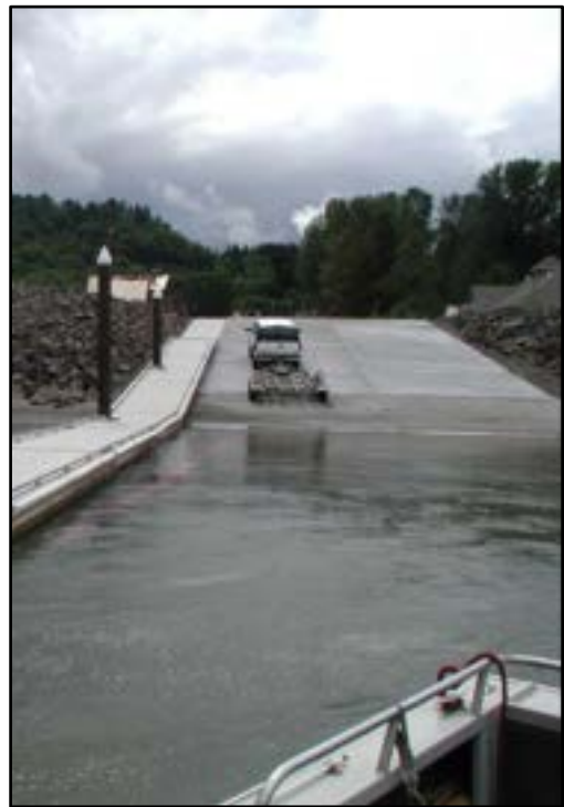
Photo 3-12 Two-lane launch ramp with boarding floats down one side only
