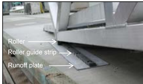
Photo 7-8 Runoff plate at float end of gangway. A grooved roller rides on the HDPE roller guide strip and provides side-restraint.
