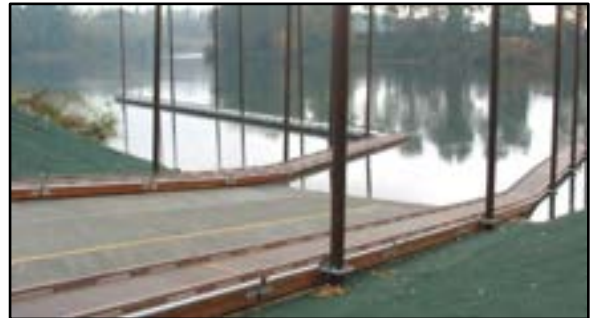
Photo 4-1 Boarding floats with dogleg section
