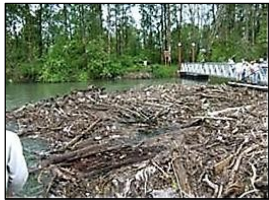
Photo 8-2 Debris accumulation at a transient float facility. This occurred during a normal high water event. A debris deflection boom was subsequently installed to protect the facility.
