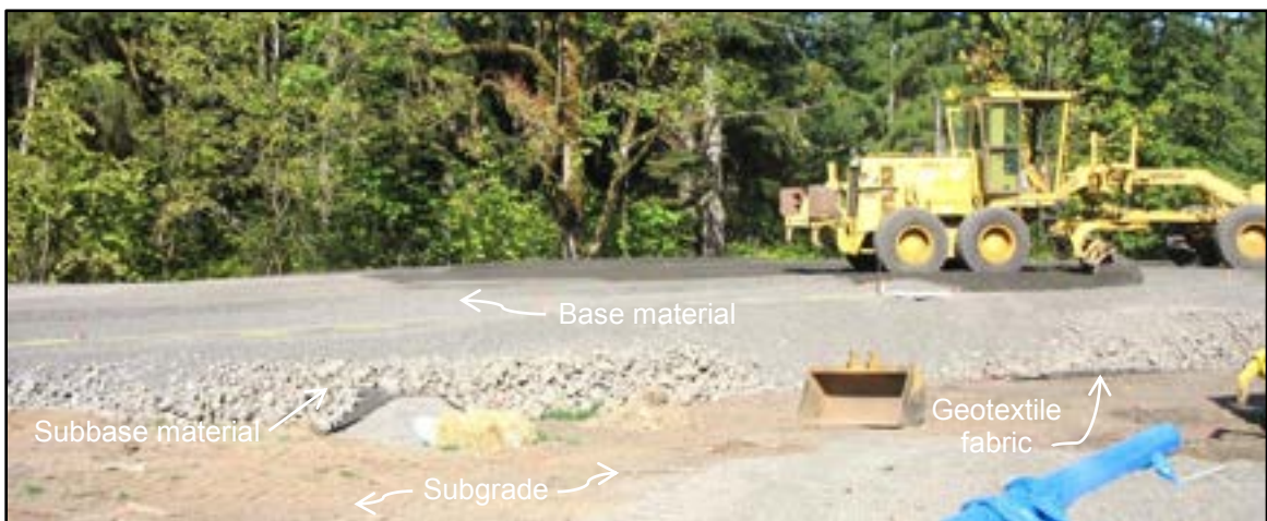
Photo 9-3 Pavement section during final grading
