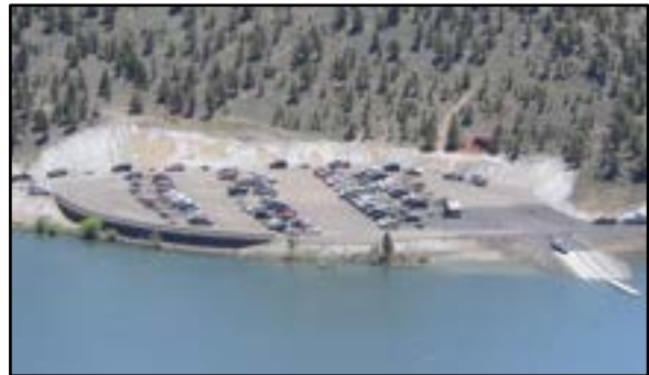
Photo 3-1 Launch facility where a large cut (parking lot) and fill (launch ramp) was required to fit the local topography
