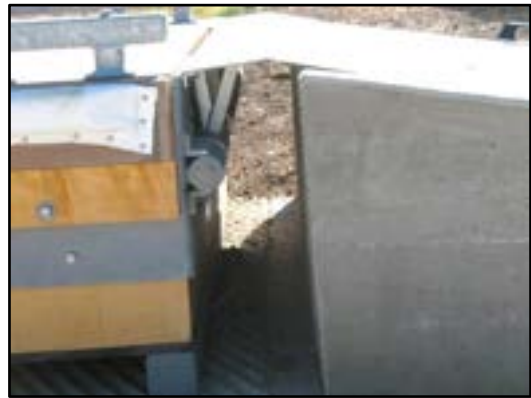
Photo 4-14 Transition plate connection
