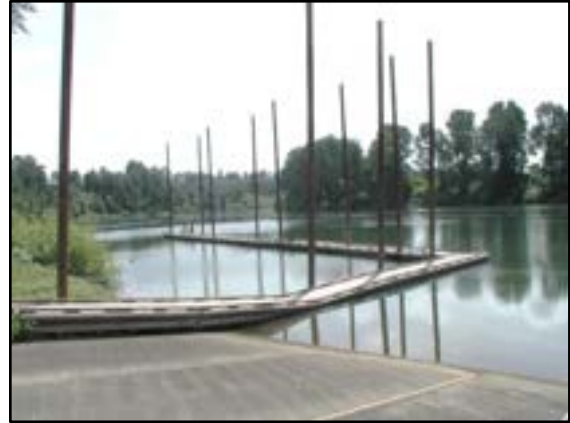
Photo 5-16 Boarding float connection to uplands
