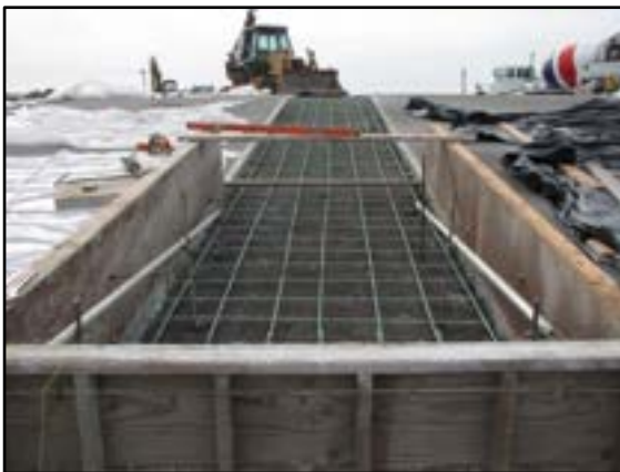
Photo 4-5 Float abutment formed and ready for concrete
