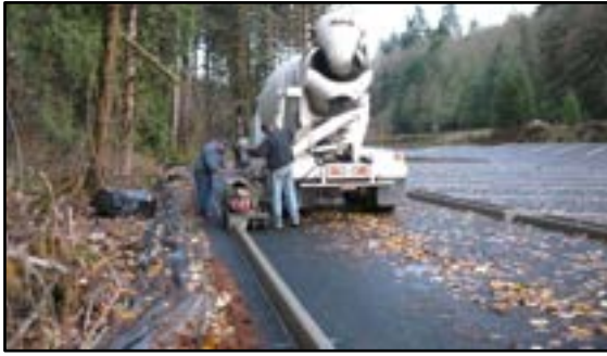
Photo 9-4 Installation of extruded concrete curb
