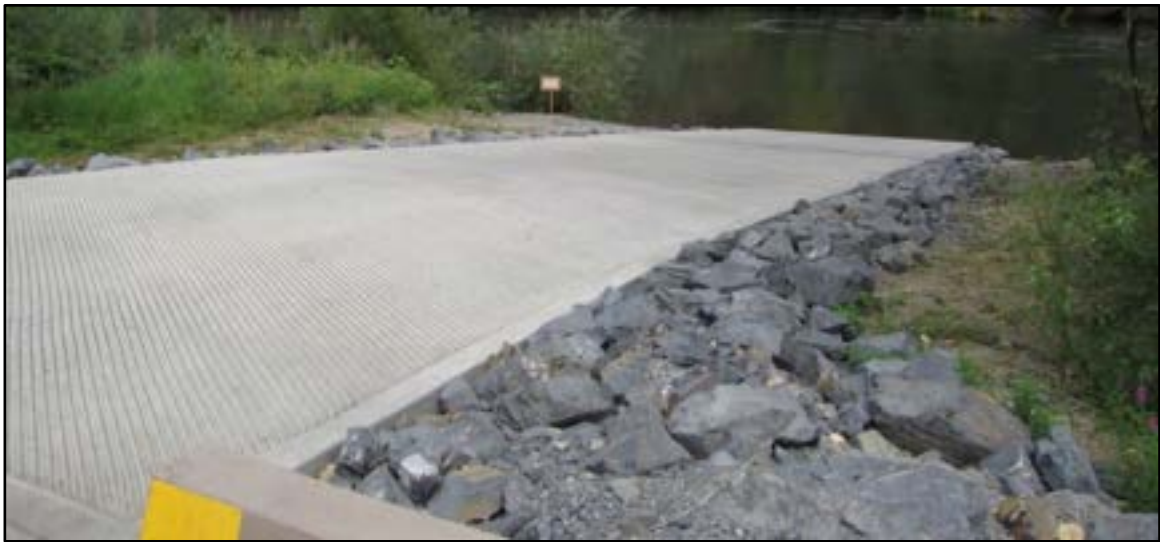
Photo 3-9 Single-lane launch ramp without boarding floats
