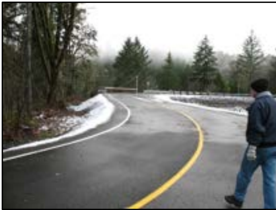
Photo 9-6 Typical two-lane access road
