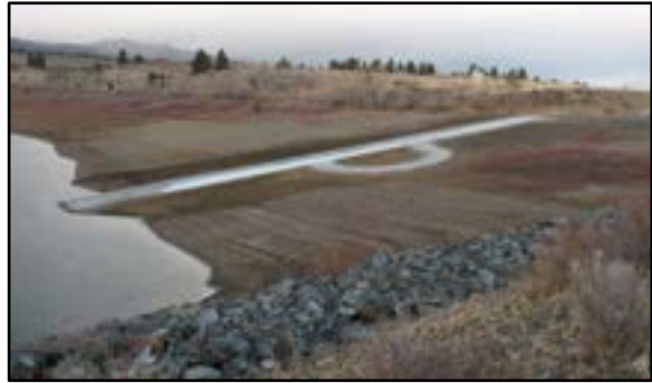
Photo 3-8 This launch ramp is nearly 400 feet in length and is designed with a turnout at the halfway point
