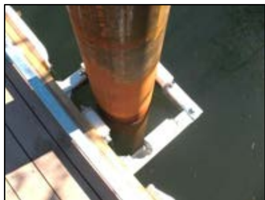
Photo 4-12 External pile hoop
