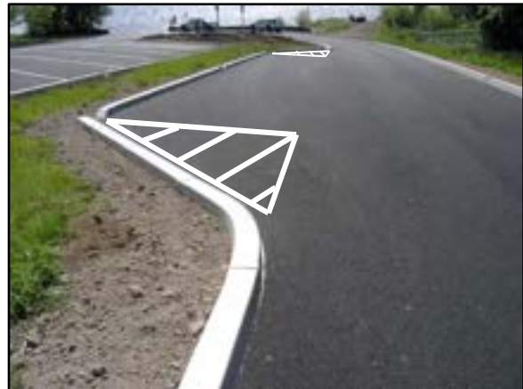
Photo 9-8 Ready area adjacent to travel lane
