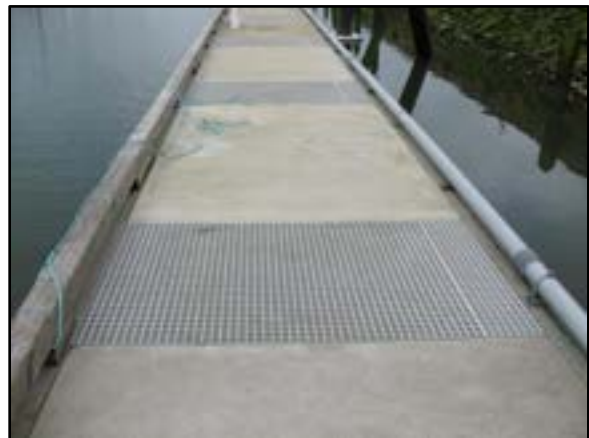
Photo 5-12 Grating in deck surface to allow for light penetration through the float
