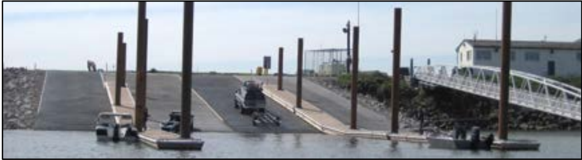
Photo 3-15 Four-lane launch ramp with boarding float access for each lane
