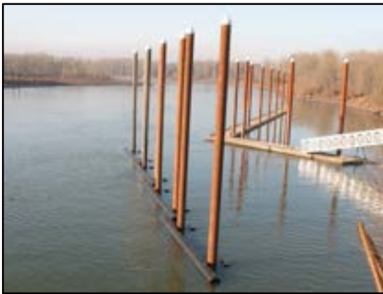
Photo 8-4 Poly-pipe debris boom
