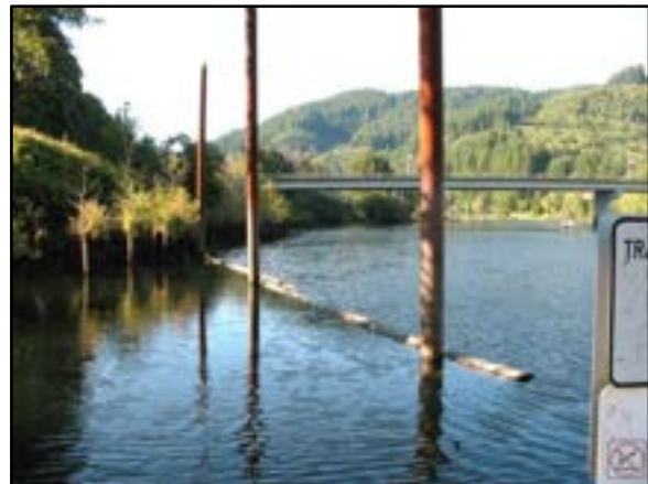
Photo 8-3 Log debris boom
