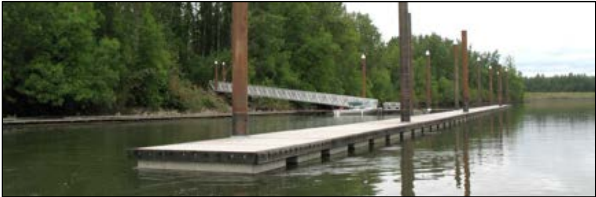
Photo 5-9 Transient float configuration with gangway located at midpoint
