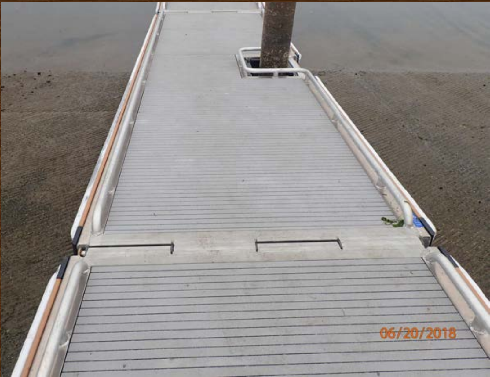
DOCK JOINT & PILE POCKET
