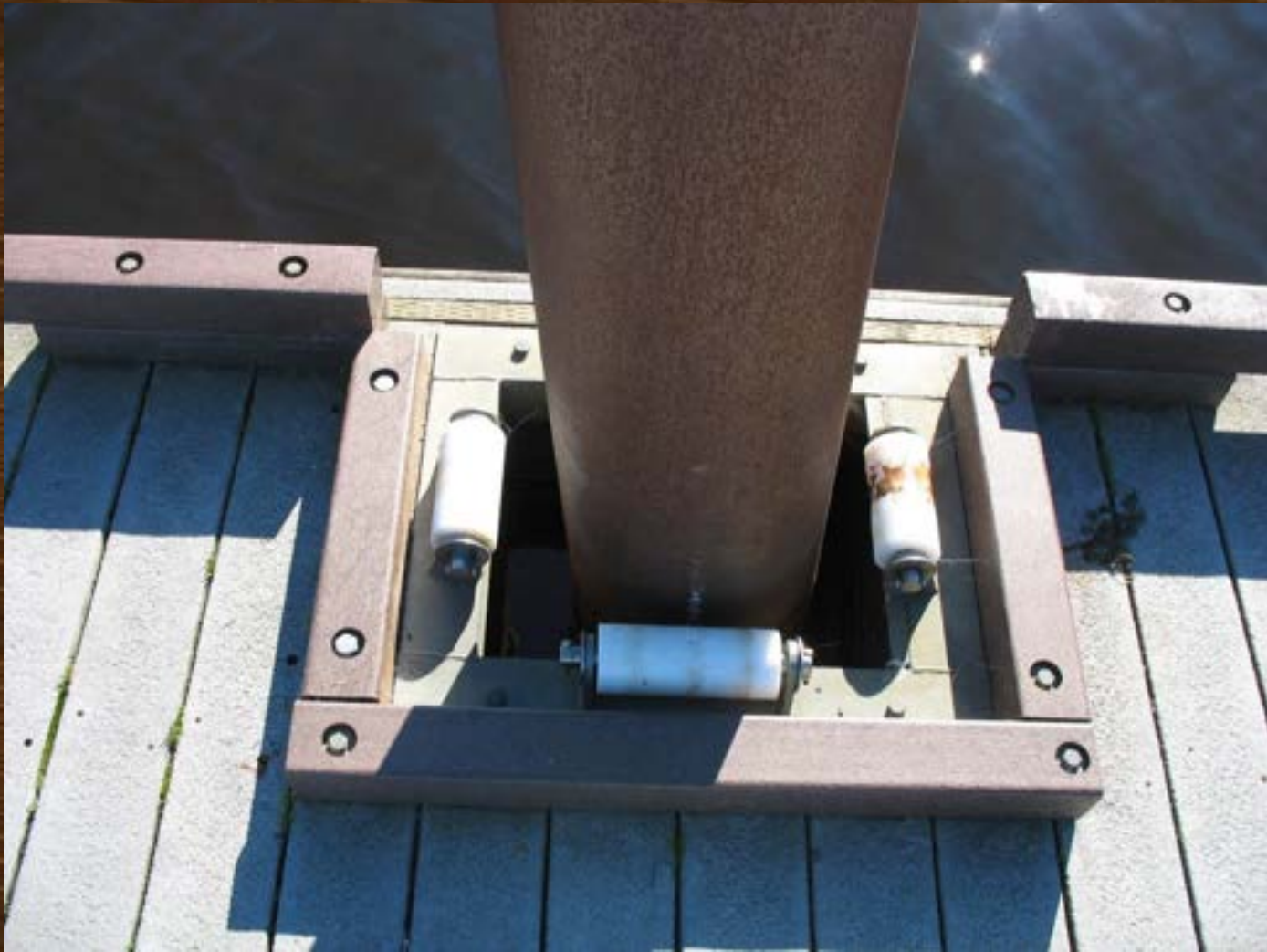
INTEGRATED PILE HOOP
