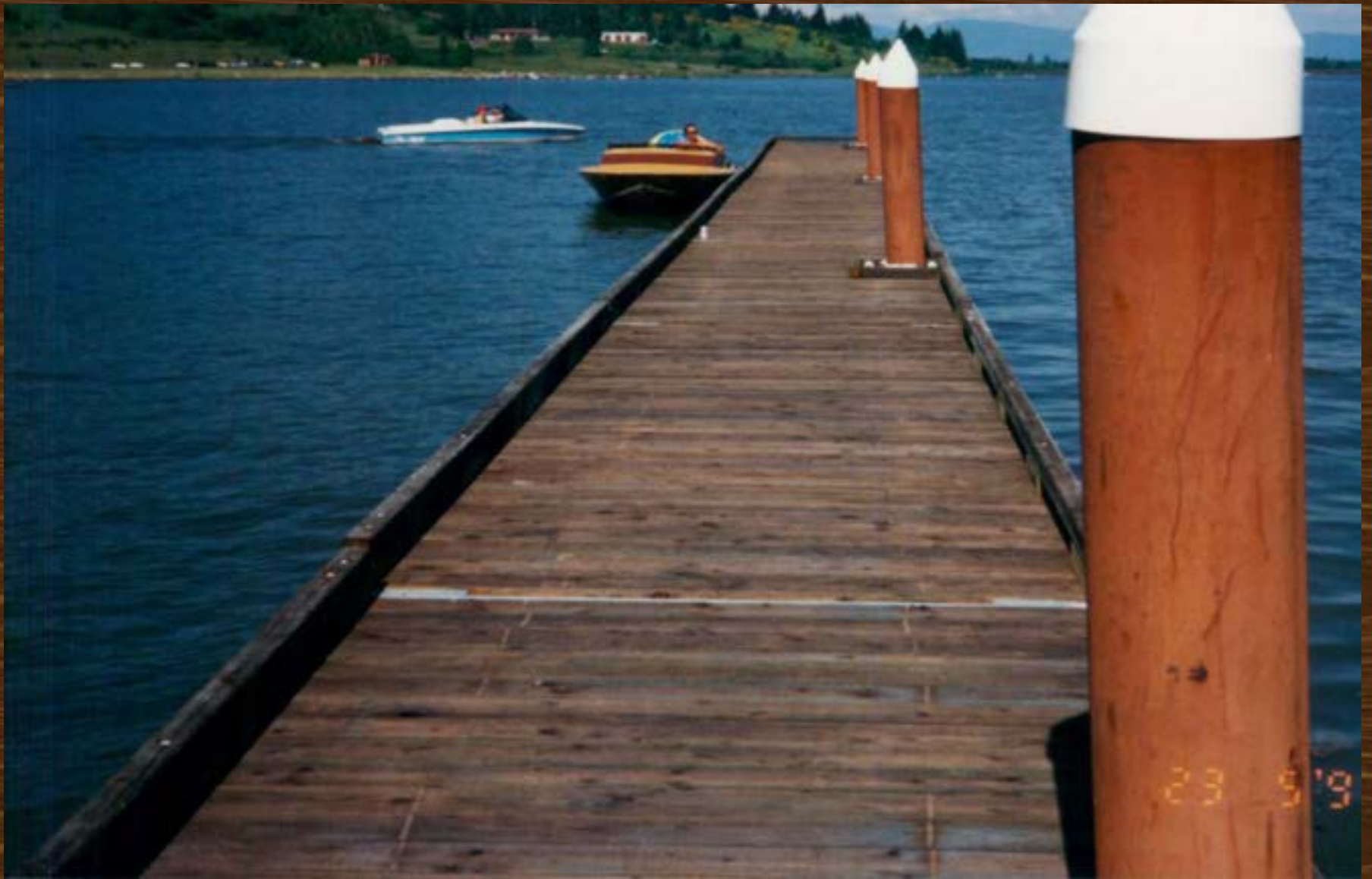
PERPENDICULAR DECK BOARDS
