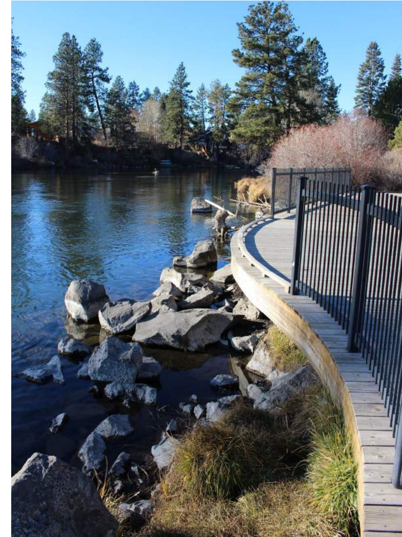
The boardwalk access point is challenging for users given the significant height difference between the water and the boardwalk, and the existing jagged rocks. Current design limits the number of individuals who can access the water with their kayaks and SUPs at this access point.
