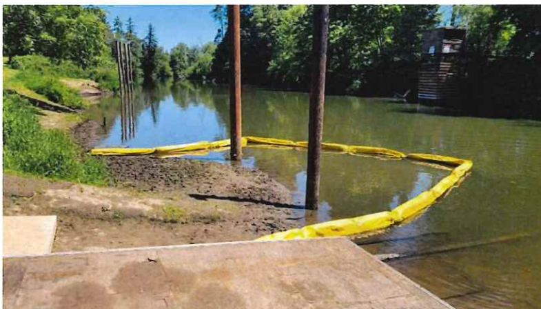
New Tigard Dock – First Water Trail improvement since 2017
