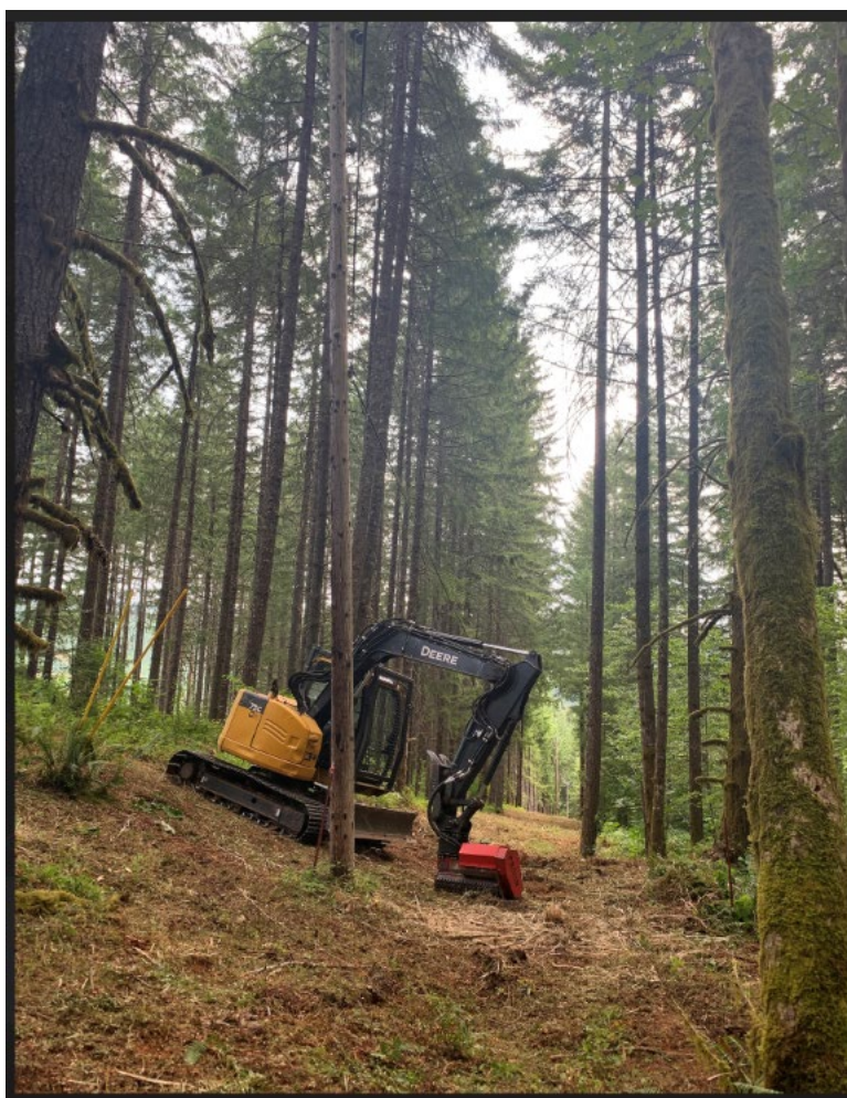
Figure 16: SlashBuster Clearing Right-of-Way
