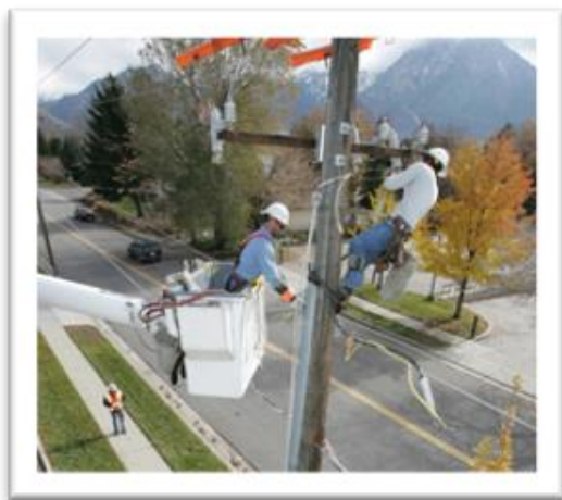
Figure 18: Lineworkers Preparing a Pole for New Covered Conductor
