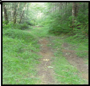
Weyerhaeuser road decommission to help prevent long term culvert failure and road washout.
