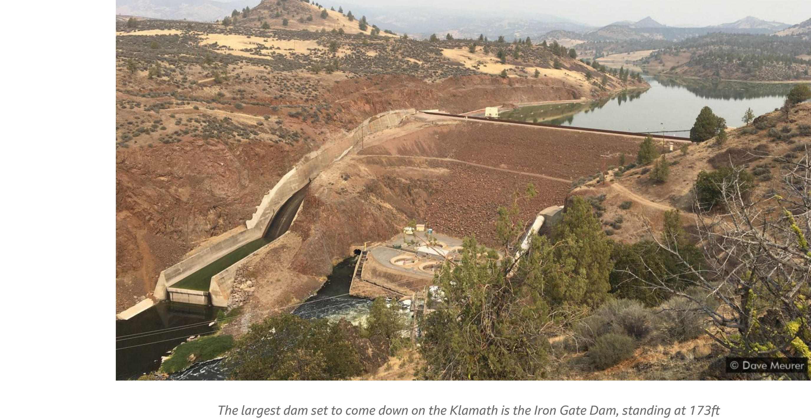
The largest dam set to come down on the Klamath is the Iron Gate Dam, standing at 173ft (53m) high (Credit: Dave Meurer)
