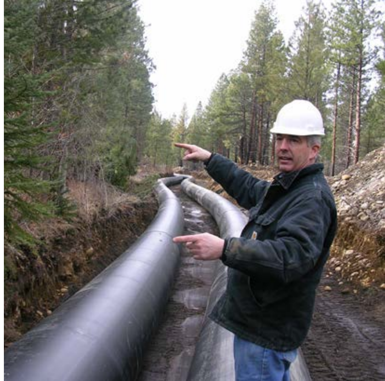
Deschutes Basin Partnership - Three Sisters Irrigation District Manager Marc Thalacker oversees canal piping, enabling flow restoration in the Creek.
