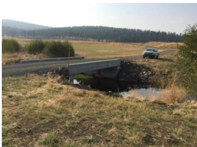
Photo 1. Upper Fox Creek, in the John Day Basin, before and after photos of a culvert replacement and bridge installation project completed by the Confederated Tribes of Warm Springs.
