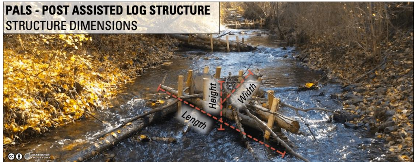
FIGURE 15. EXAMPLE OF DIMENSIONS USED IN THE RECORDING OF PALS OR NATURAL WOODY DEBRIS ACCUMULATION LENGTH, WIDTH, AND HEIGHT ULTIMATELY USED TO ESTIMATE A VOLUME OF WOODY DEBRIS ACCUMULATIONS.
